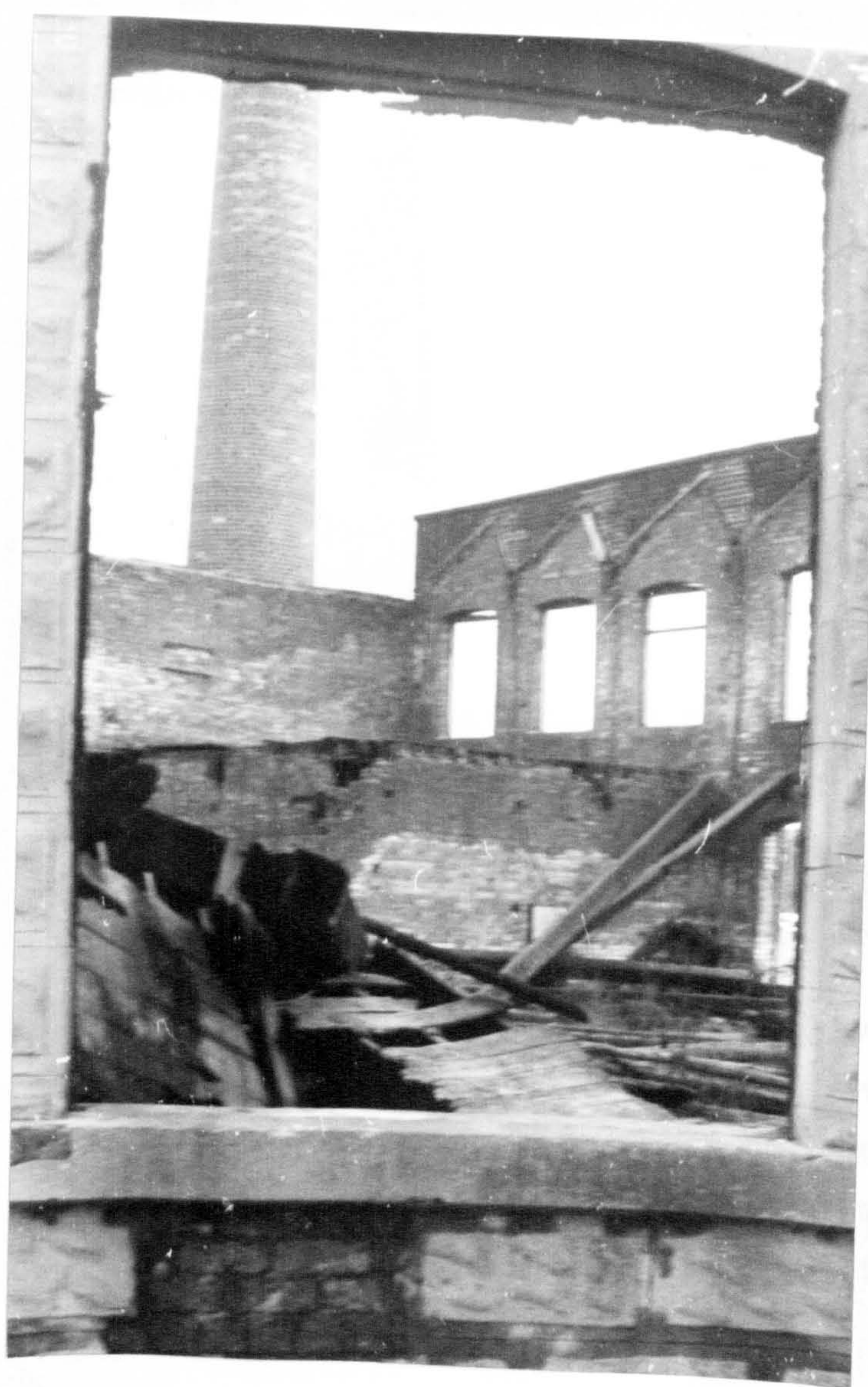
7. PERSEVERANCE MILL (67) J. Charnock built this as a dressing mill in 1839 on the site of an earlier foundry. By 1866 it had become Gillam's Trafalgar Iron Foundry. The small-paned, cast-iron framed fireproof windows are the originals but the chimney is of a later date.
