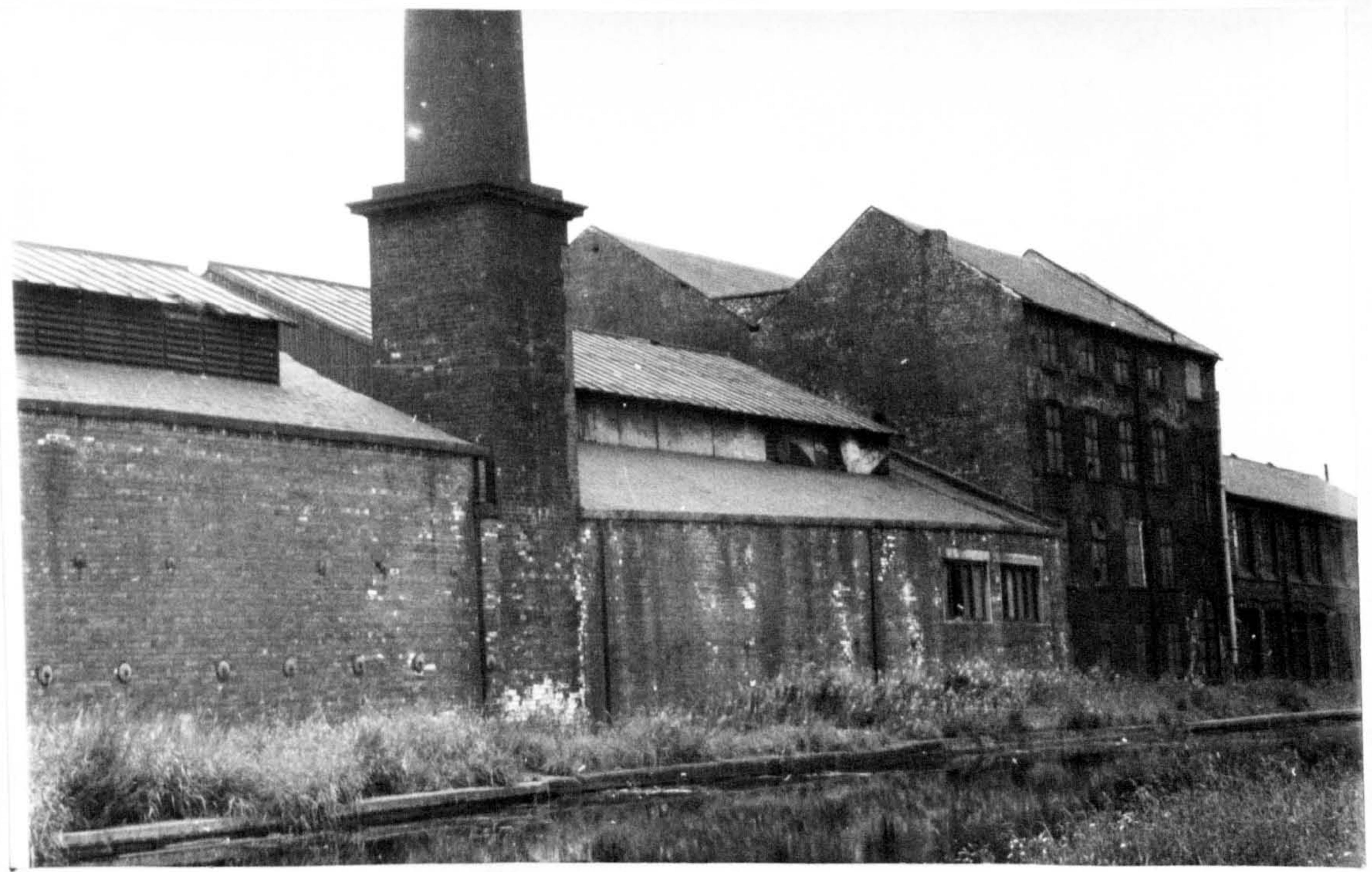
75. GLOBE FOUNDRY & FLOUR MILL (33) Architecturally this is one of the most interesting sites in Holbeck. From the canal bank can be seen the original Globe Foundry of 1844 and to the right, Clough's Globe Flour Mill and Lewiss' Clothing Factory. The flour mill is of brick with red pantiles and until recently was a cigar factory.
