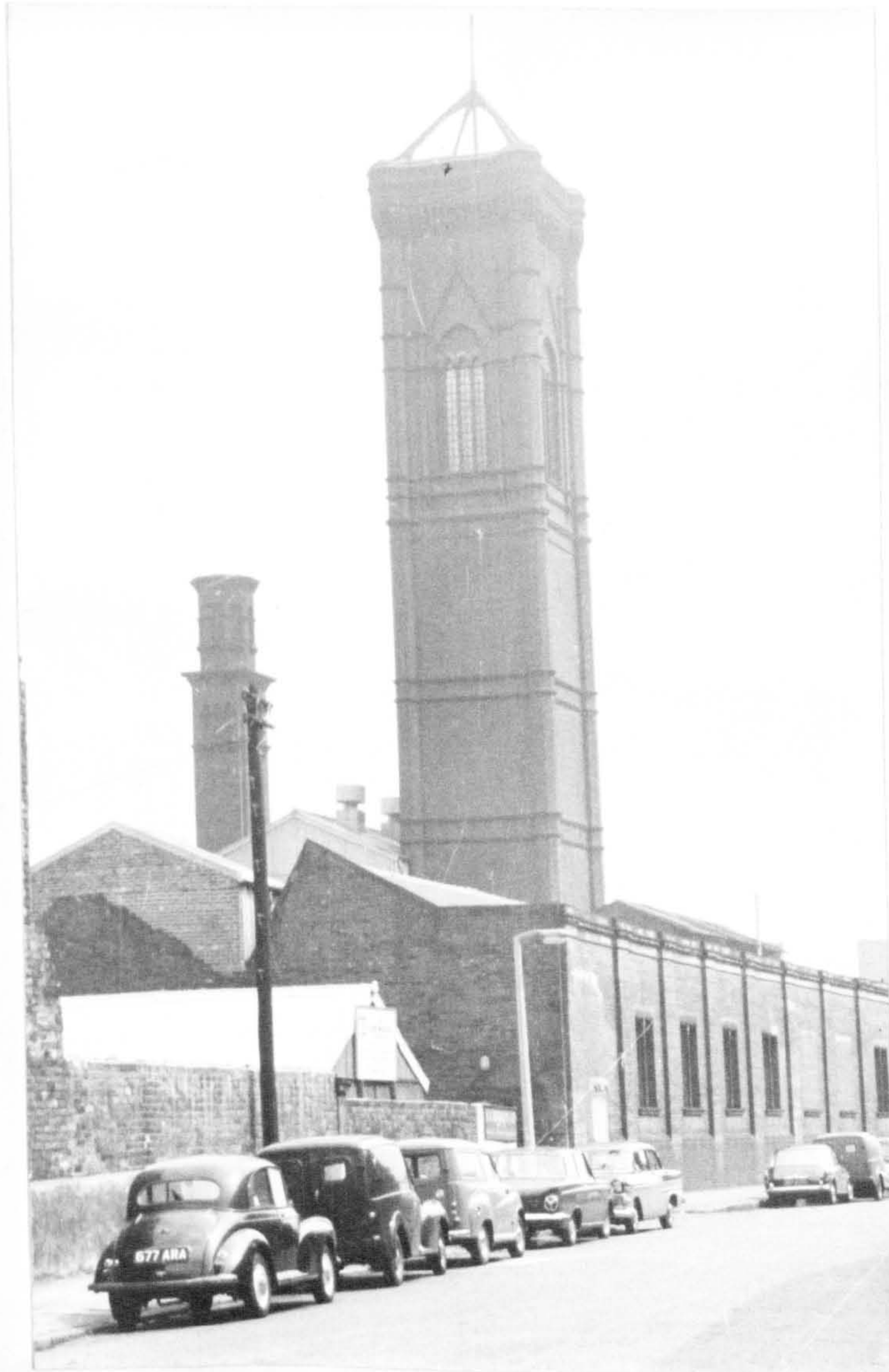
78/79 In 1900 the top of the chimney was removed and the great ventilation tower was built, this time based on a Florentine Church tower. On the base of the tower are medallion portraits of great engineers. The gates are also richly decorated with bas-relief figures.
