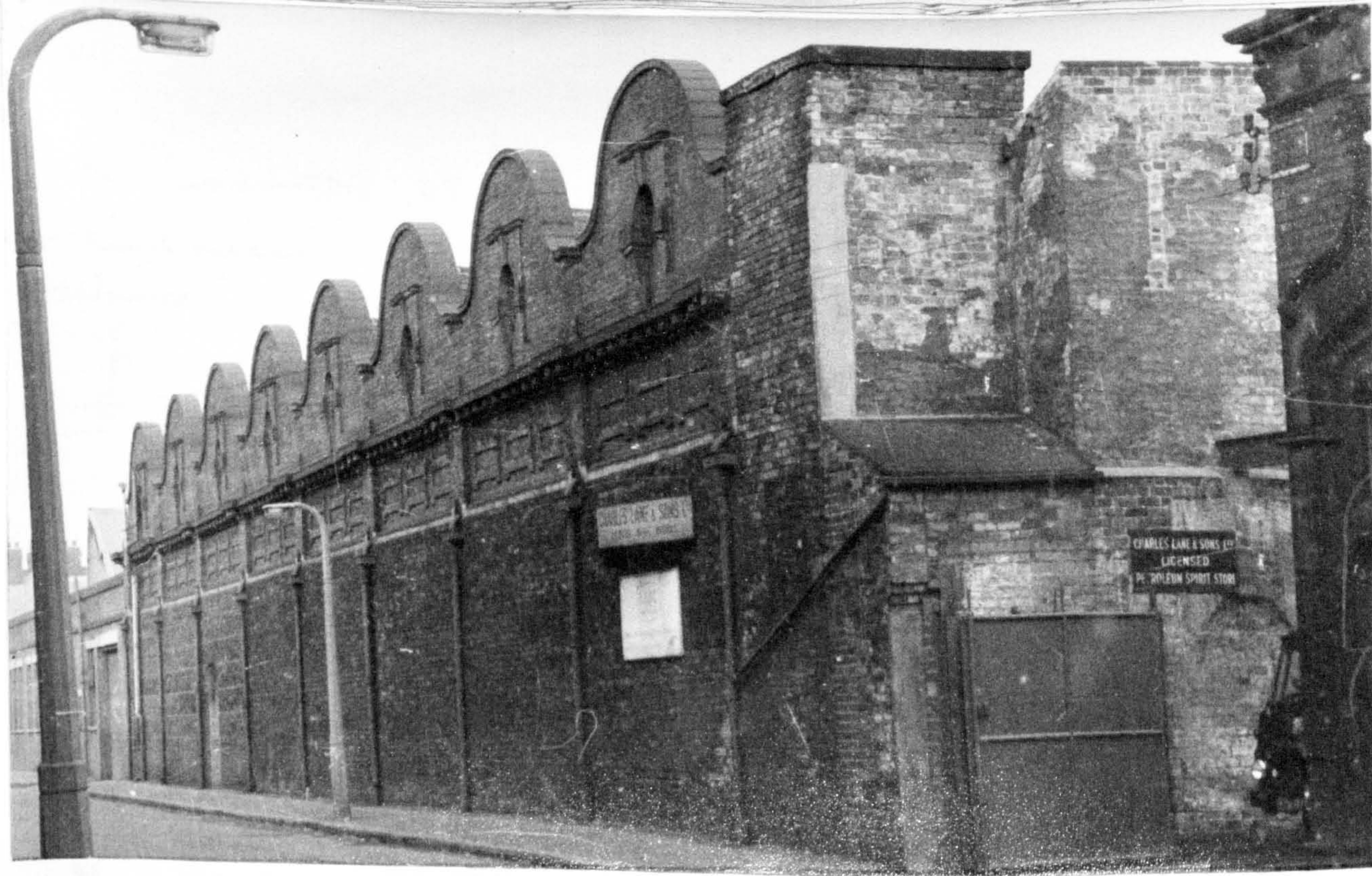
74. LEEDS NAIL WORKS (167) Charles and Edwin Roberts moved to this site in 1869 and are still in business there. The rounded gables conceal eight lines of north-light roof over the nail-making shops (c.f. Maenson Works)
