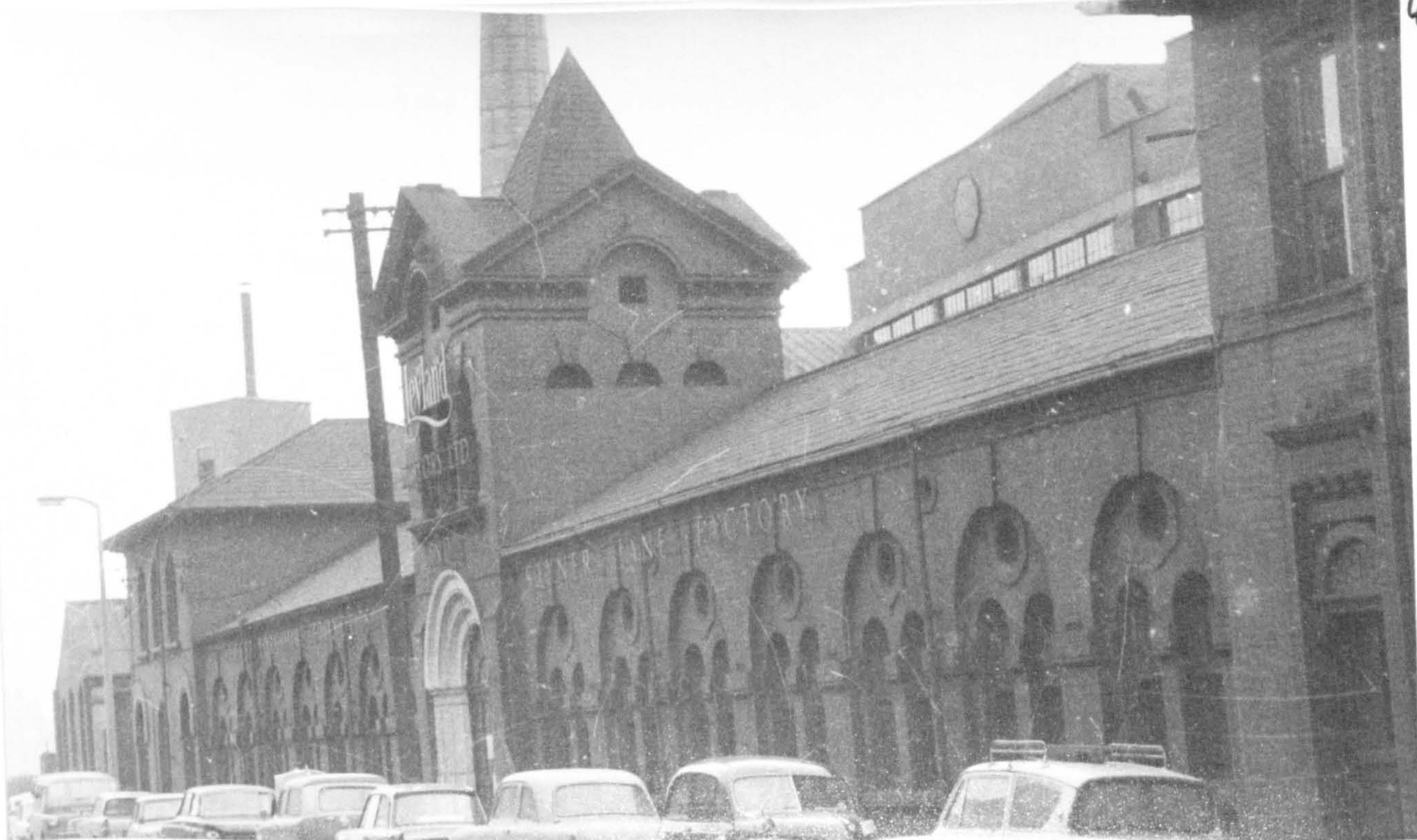
59. CLARENCE IRON WORKS (154) Taylor Bros. bought the site from the Denison and Wilkinson trustees in 1866. The round arch enclosing two round arched windows is the basic motif of the office block, built by Nicholson. Behind were 17 puddling furnaces and five rolling mills for the manufacture of 'Best Yorkshire Iron'.
