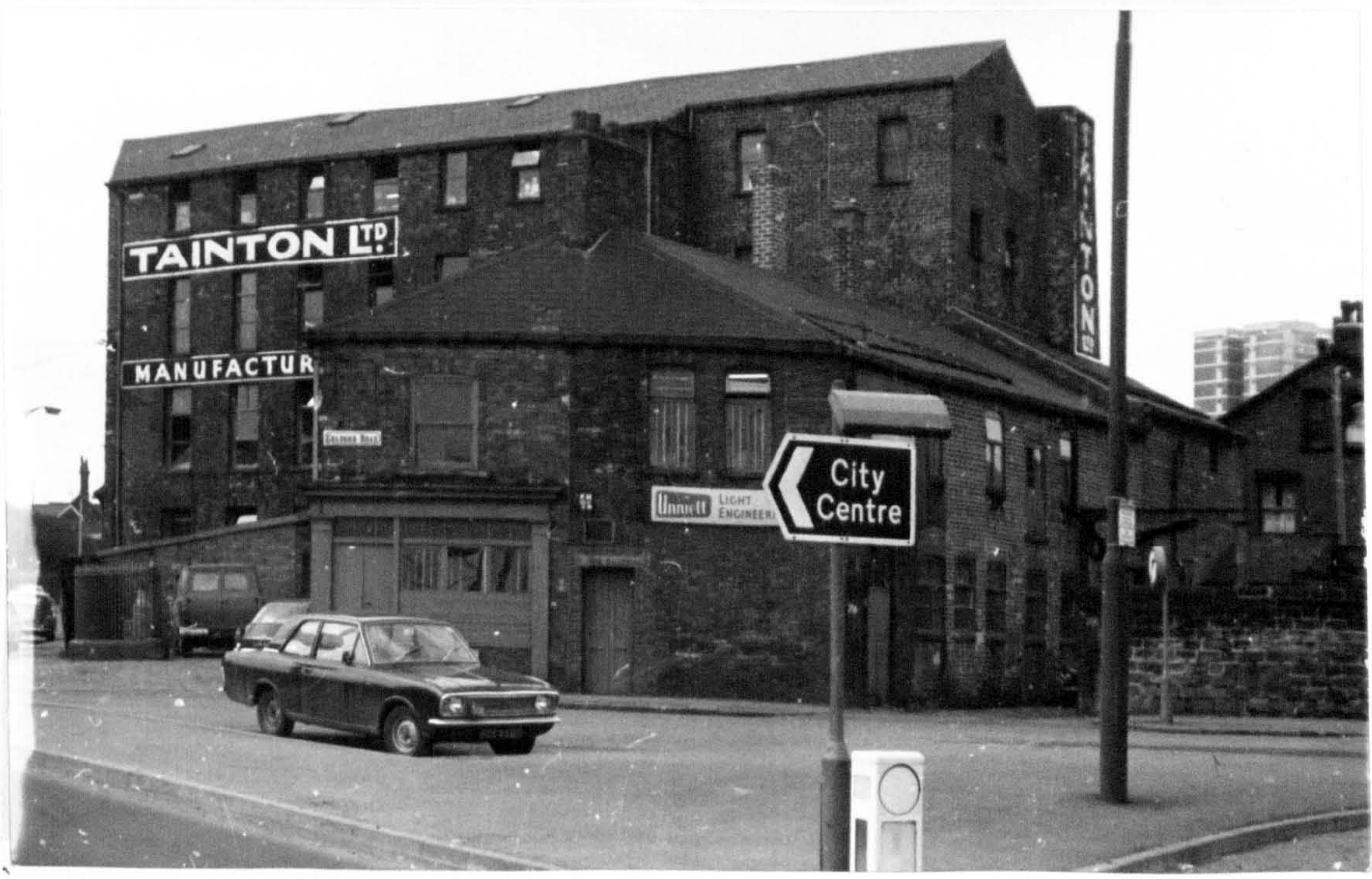
29. UNION MILL (1) The chimney has been almost removed, since it is no longer used.
