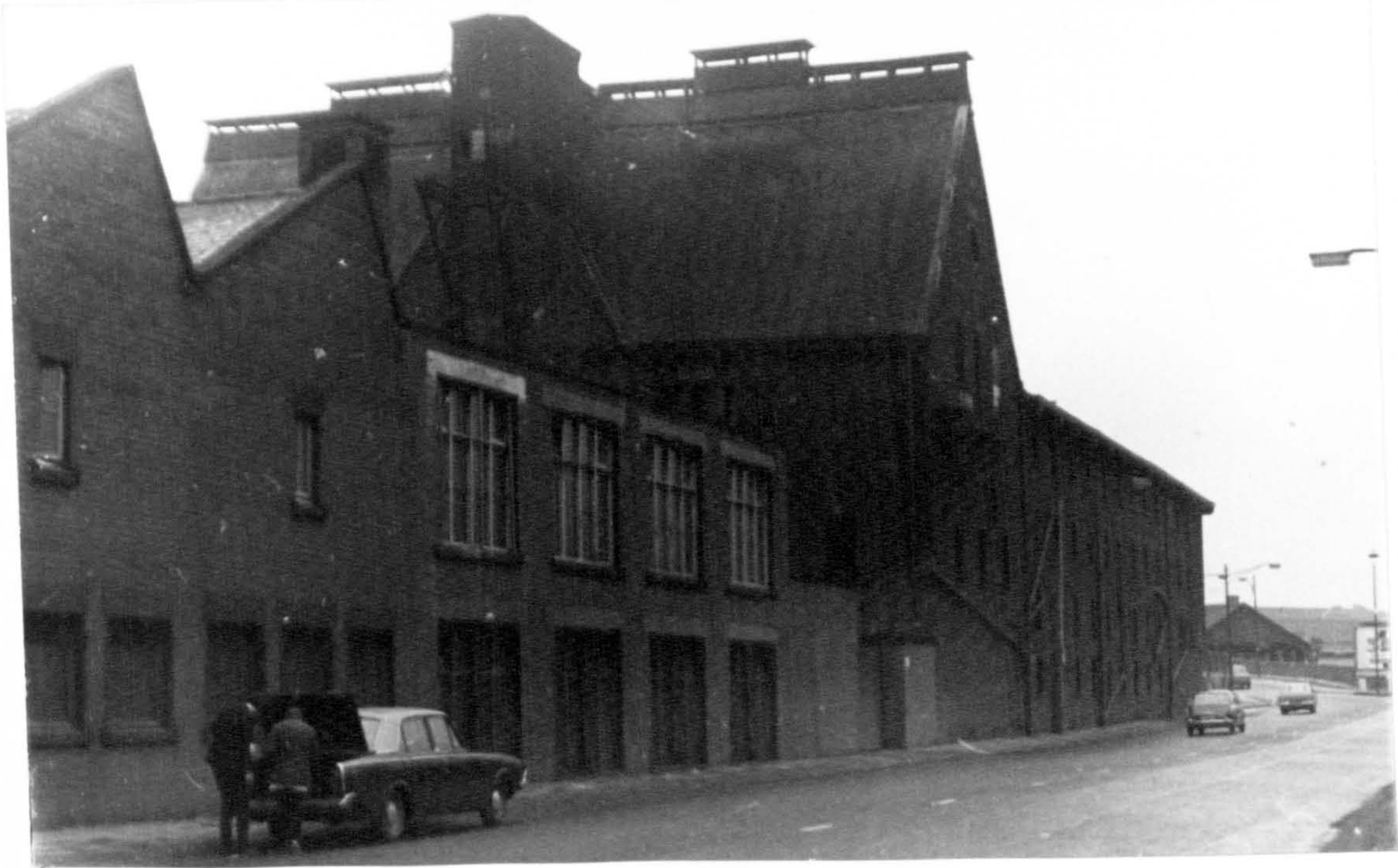
35. CROWN POINT MALKILN (90) The original maltkiln of Syke's brewery was replaced by the one shown (demolished 1974). It was built by Nicholsons for Tetleys. The design is typical of the second part of the nineteenth century, with a long, ridge flue for the kiln.
