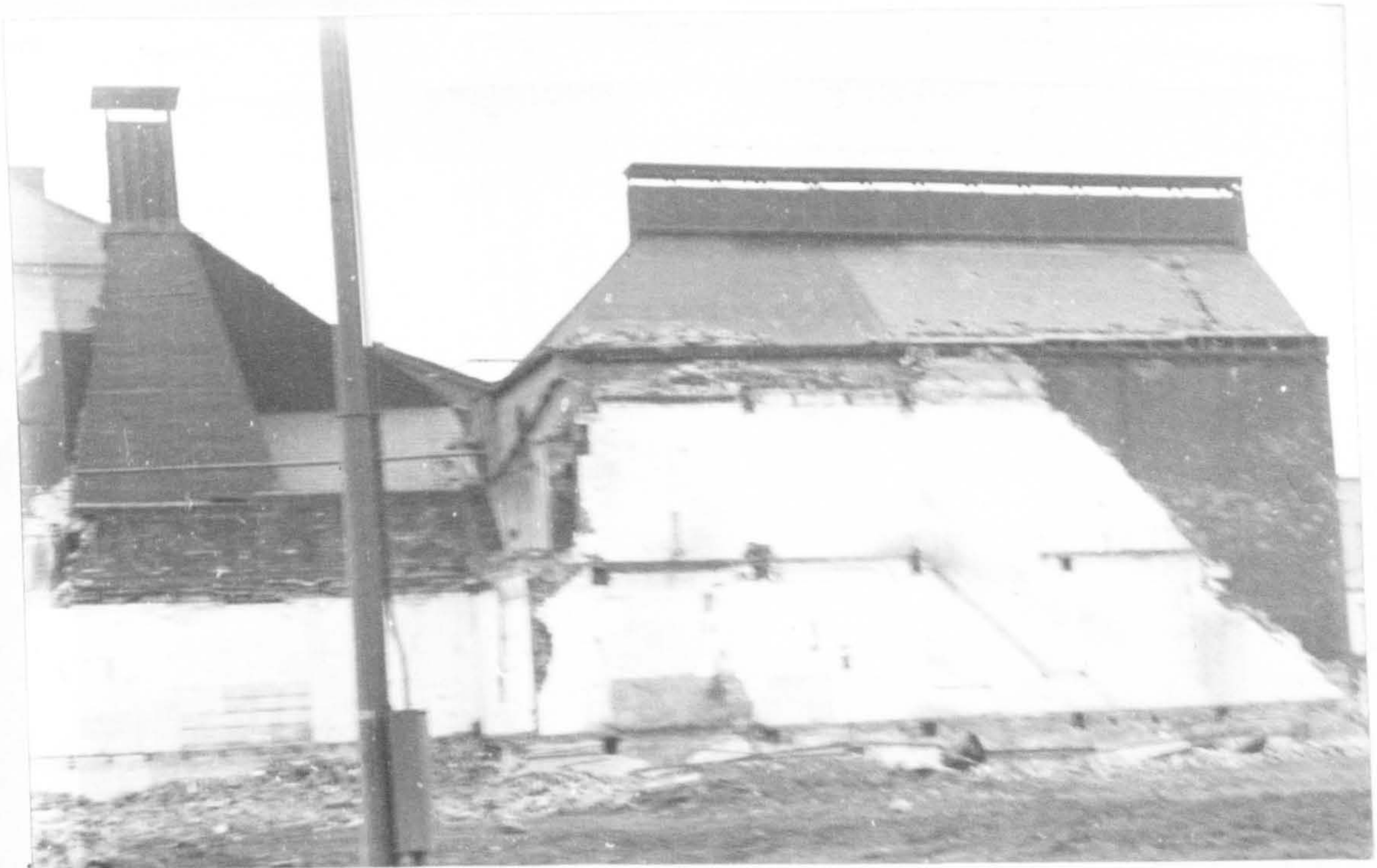
36. MEADOW MALTINGS (65) Jaques and Nells Meadow Lane Brewery was rebuilt as the Meadow Maltings in 1872 by G. Kitchen. It was the largest maltkiln unit in Leeds, there being 8 kilns with a total capacity of 197 qrs. of barley. The demolition reveals the kiln flues, the older style on the left and newer on the right.
