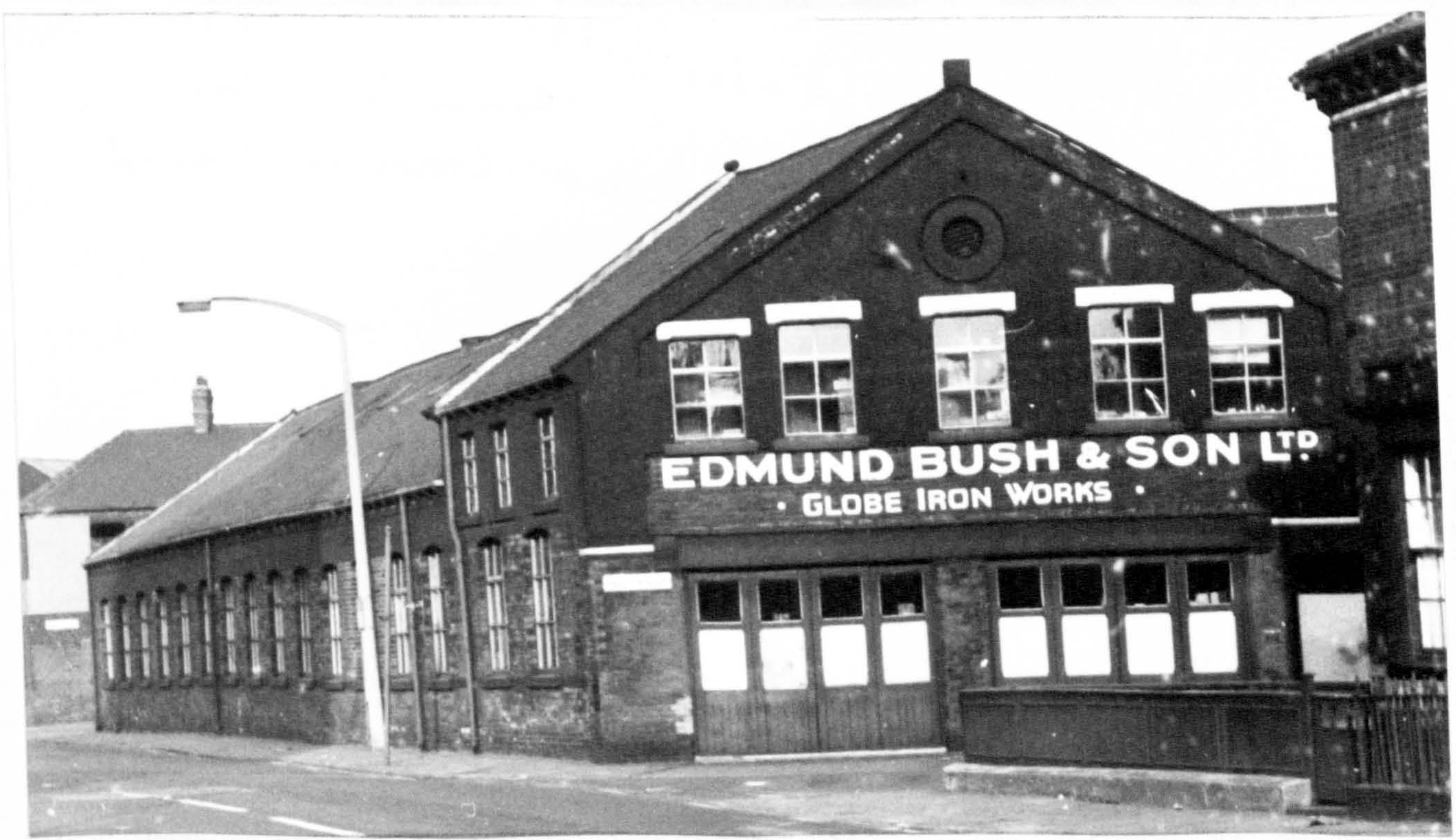
58. GLOBE WORKS (85) originally this was the 'Prospect works' of Hutton and Macdonald and in 1889 it became the Globe Iron Works of J.Green and Nephew. The output was mainly domestic castings, especially coal-chute covers. This work required a small furnace to re-melt pig-iron and a foundry for casting the molten metal. This leads to a single storey block with a wide span to give a clear floor area. The offices are over the mould shop with the sliding doors opening on to Sheaf Street.
