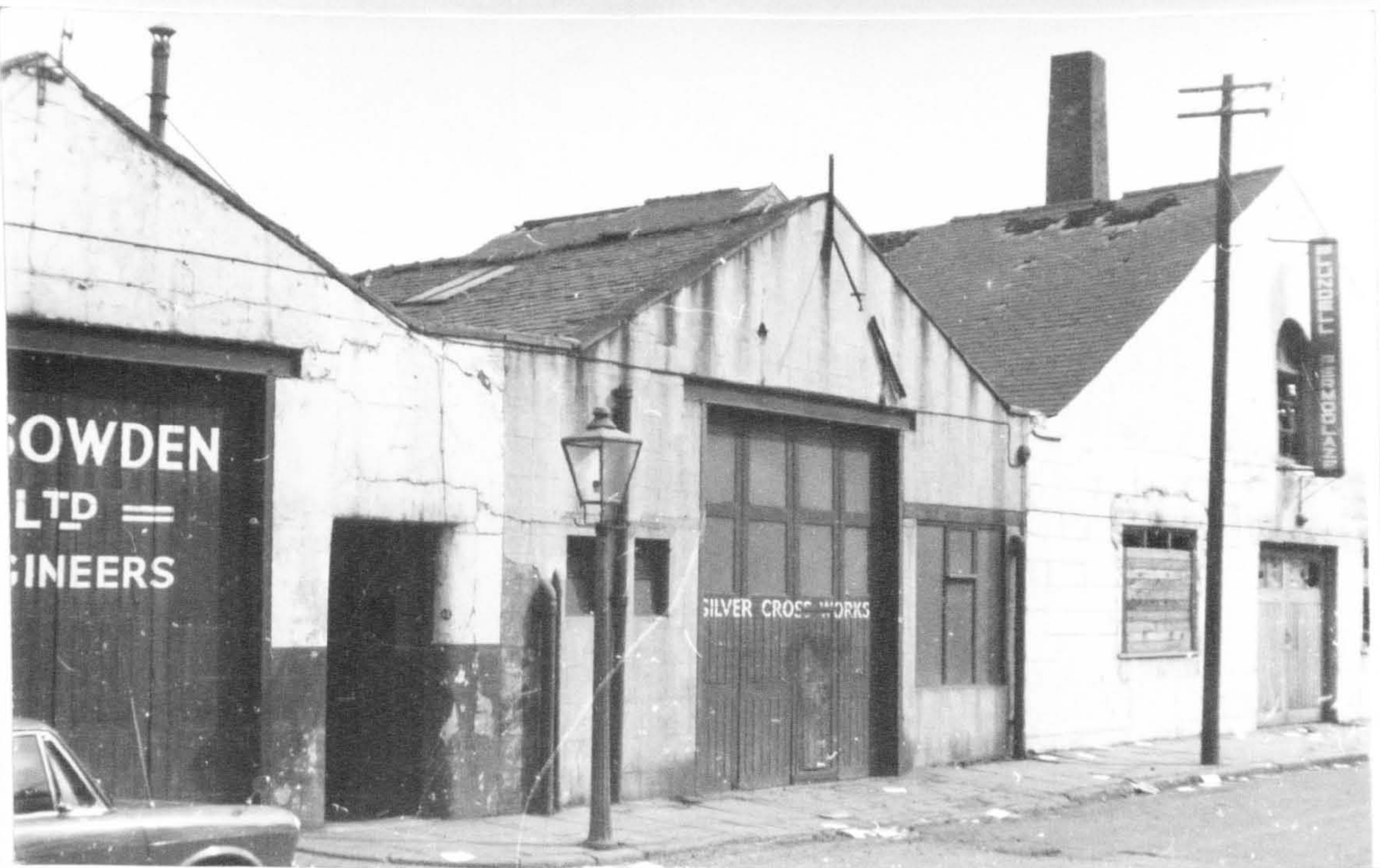
70 SILVER CROSS WORKS (140) Behind the Silver Cross Inn on Dewsbury Road John Milner built a card making workshop. In 1889 part of this was taken over by W. Wilson to make perambulators.
