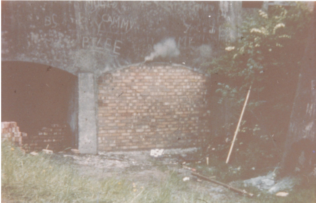
Figure 2-39 The bunkers at Potters Marston (photo from DNV GL archive)
