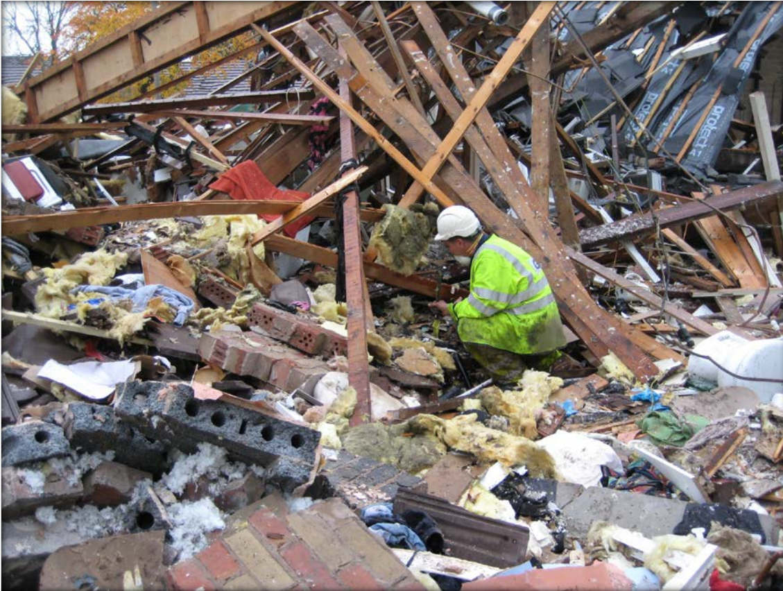
Figure 1-6 The author at the scene of a gas explosion
