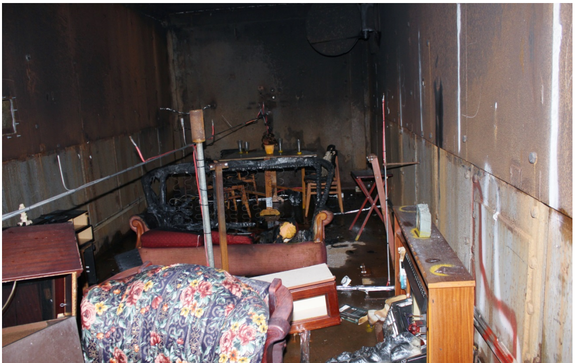
Figure 5-32 Damage following test 13
