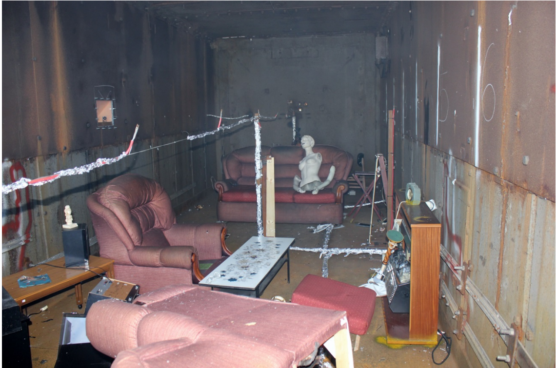
Figure 5-31 Damage following test 12
