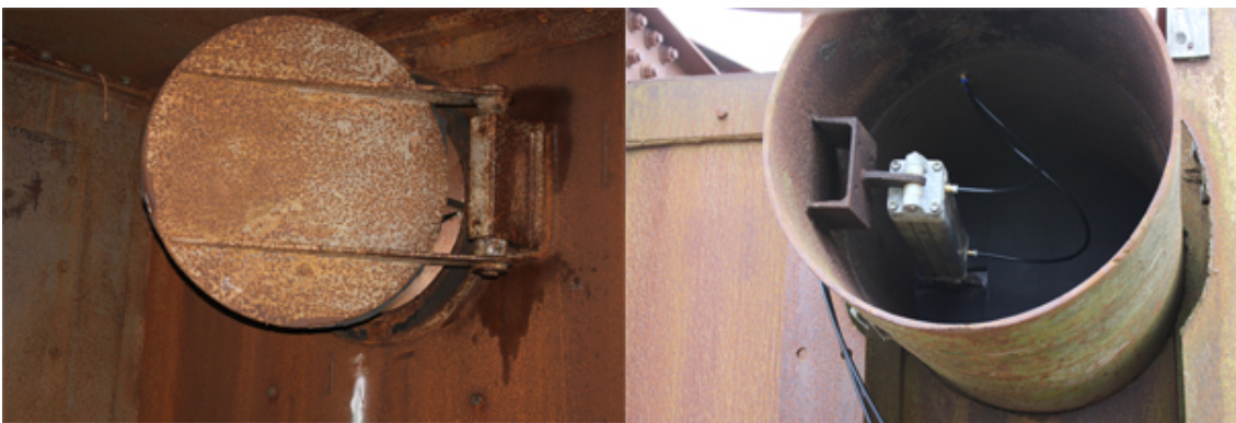
Figure 3-26 Pneumatic flap valve (left) and ram (right)
