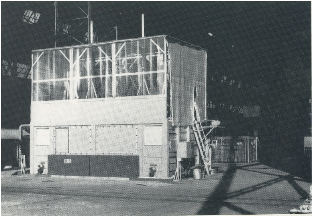
Figure 3-6 The FRS explosion chamber (Rig A)
