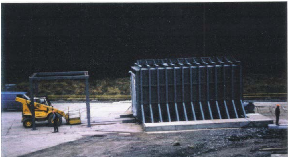
Figure 3-11 Spadeadam explosion chamber (Rig B)
