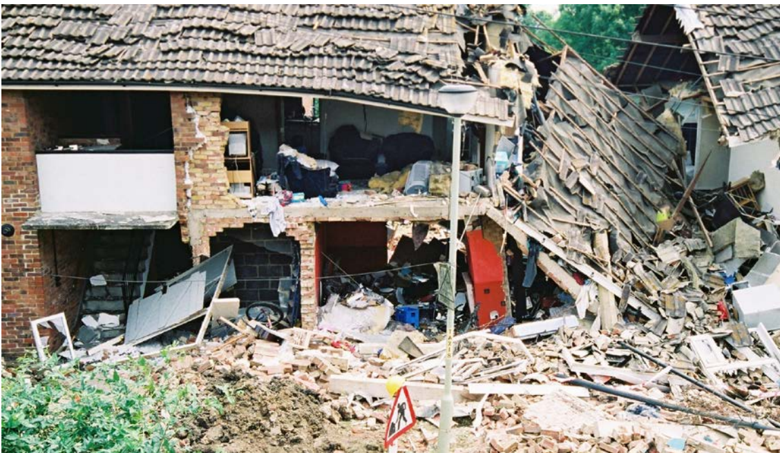
Figure 2-19 Accidental gas explosion where inadvertent venting has failed to prevent structural damage to the property
