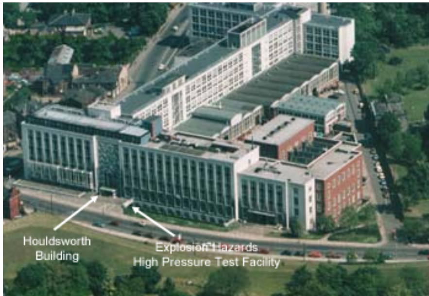
Figure 3-3 Explosion Hazards – High Pressure Test Facility
