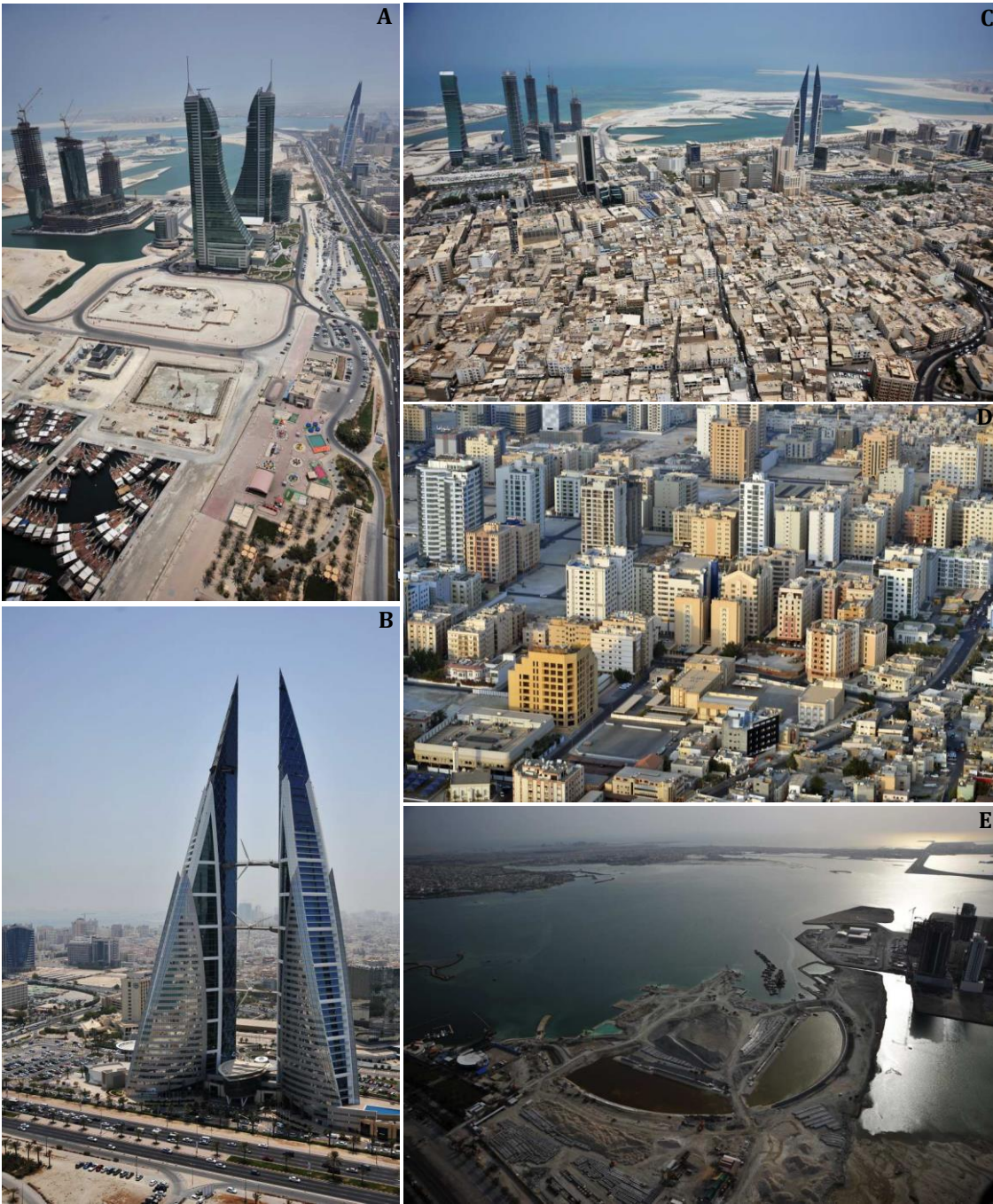
Figure 6-22 Aerial photos of Manama City, 2010 603
