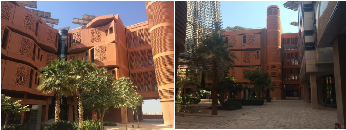
Figure 0-1 The different passive and active sustainable solutions including the solar panels, wind tower and GRC screens and louvers 853
