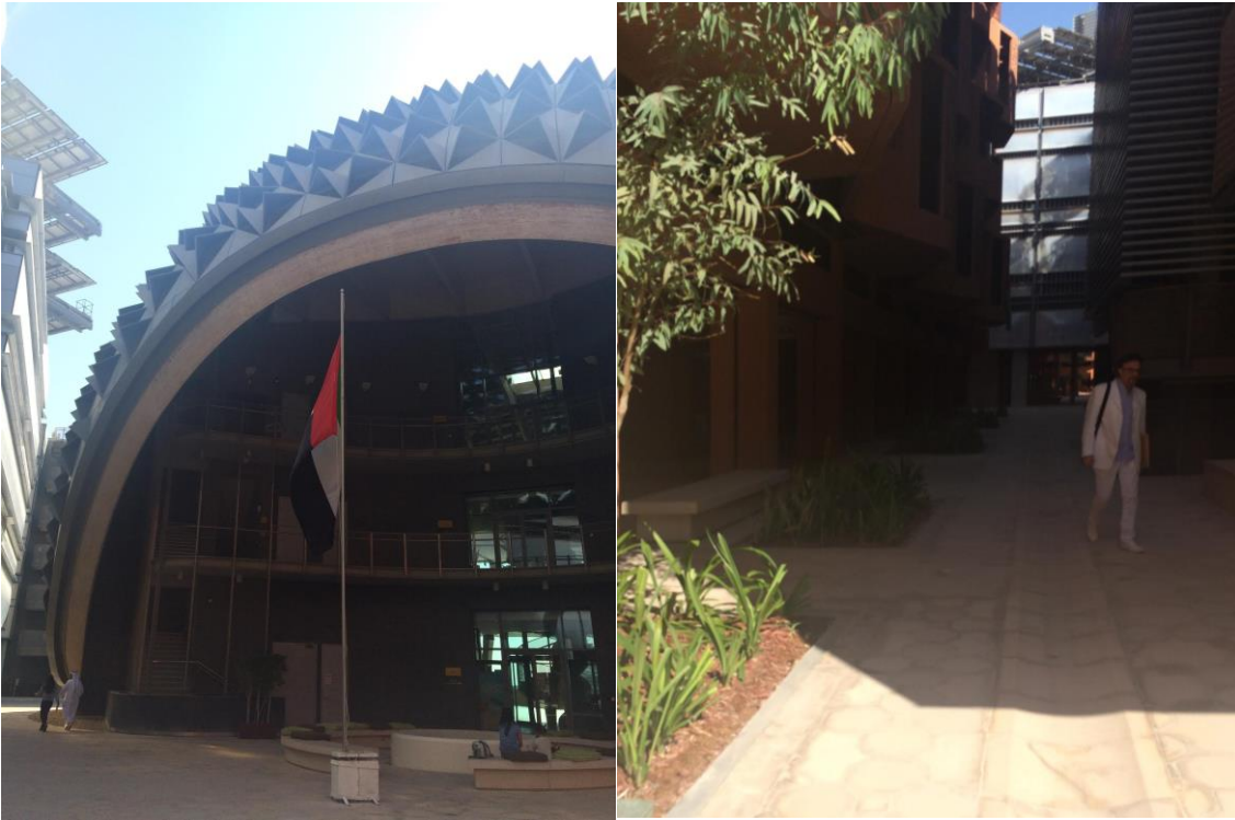
Figure 0-5 The library building and the louvers used to shade the structure (left) and the shade and shadow created by the passive design solutions (right) 857
