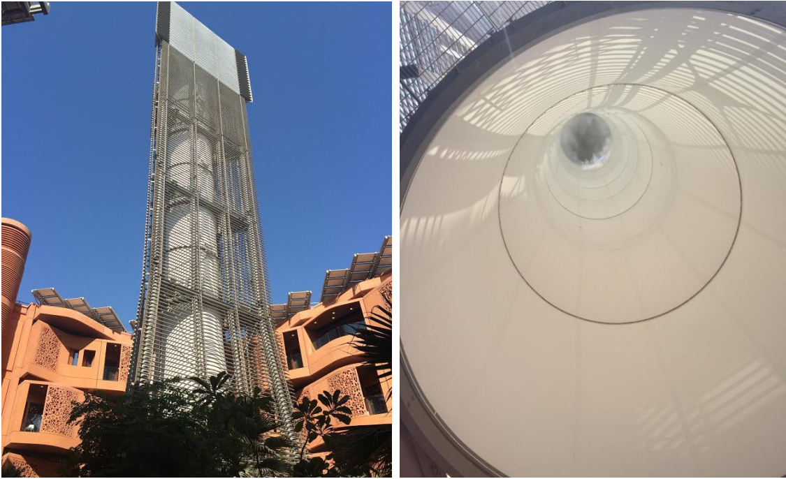
Figure 0-2 The outside of the wind tower (left) and the inside of the wind tower with the water mist (right) 854
