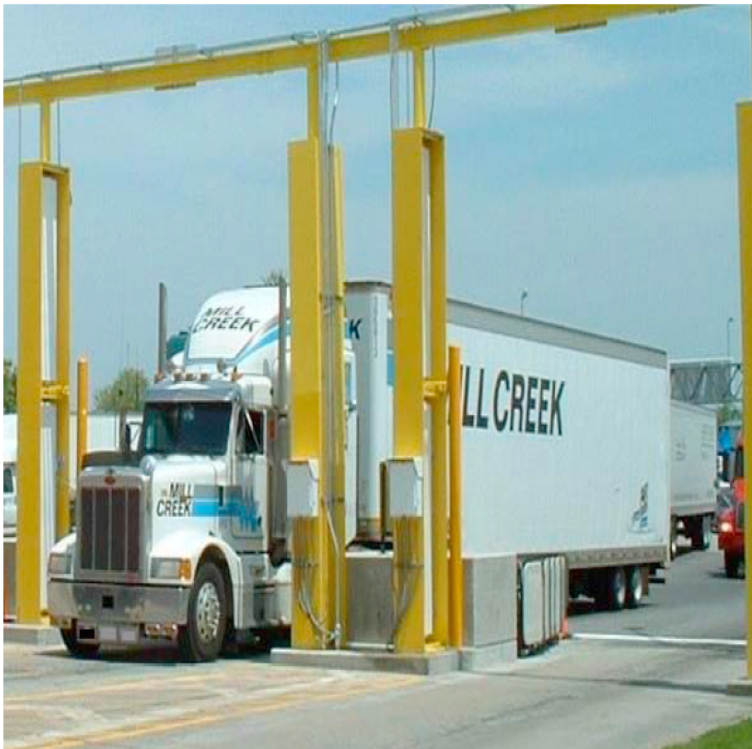
Fig. 2.1 Example display of a radiation portal monitor employed at an international border crossing [7].
