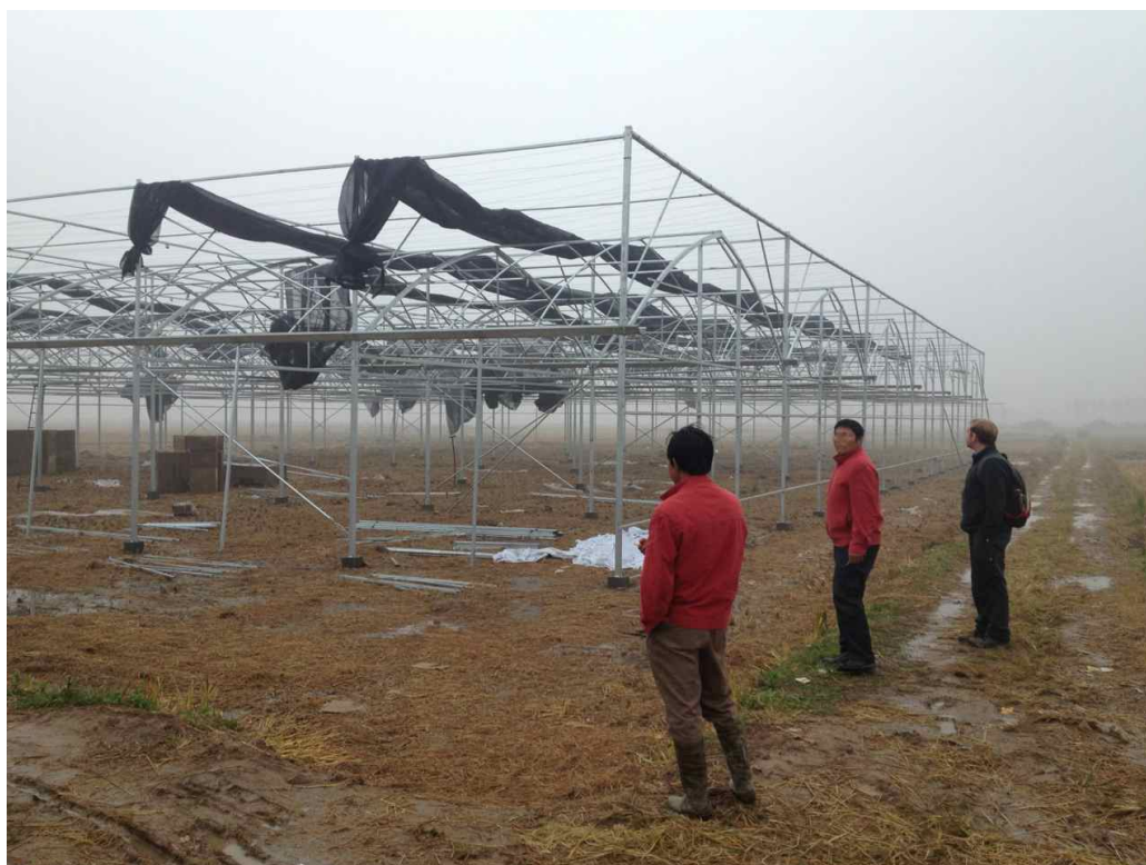
Figure 4.2: Construction of a Large Modern Vegetable Greenhouse in the AT
