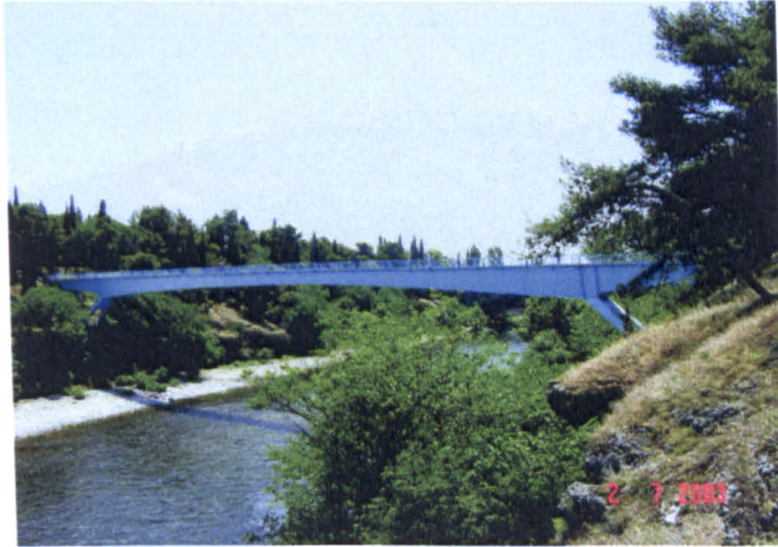
Figure 3.1: Photograph of the Podgorica footbridge.
