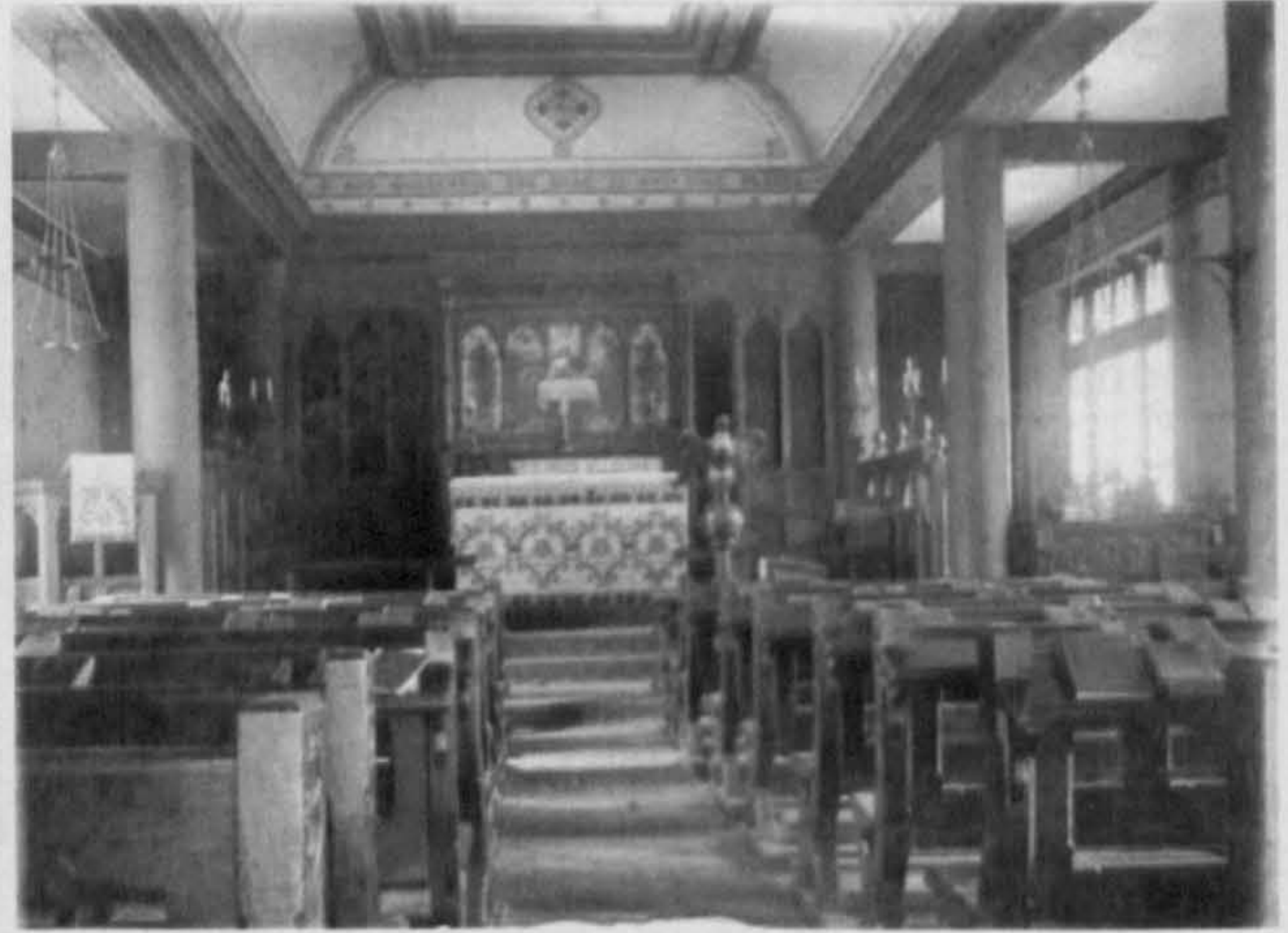
[ill.4: 10] PeKing Legation, nave and reredos of chapel. Source: WORK 10/117, date: 1946-1951.
