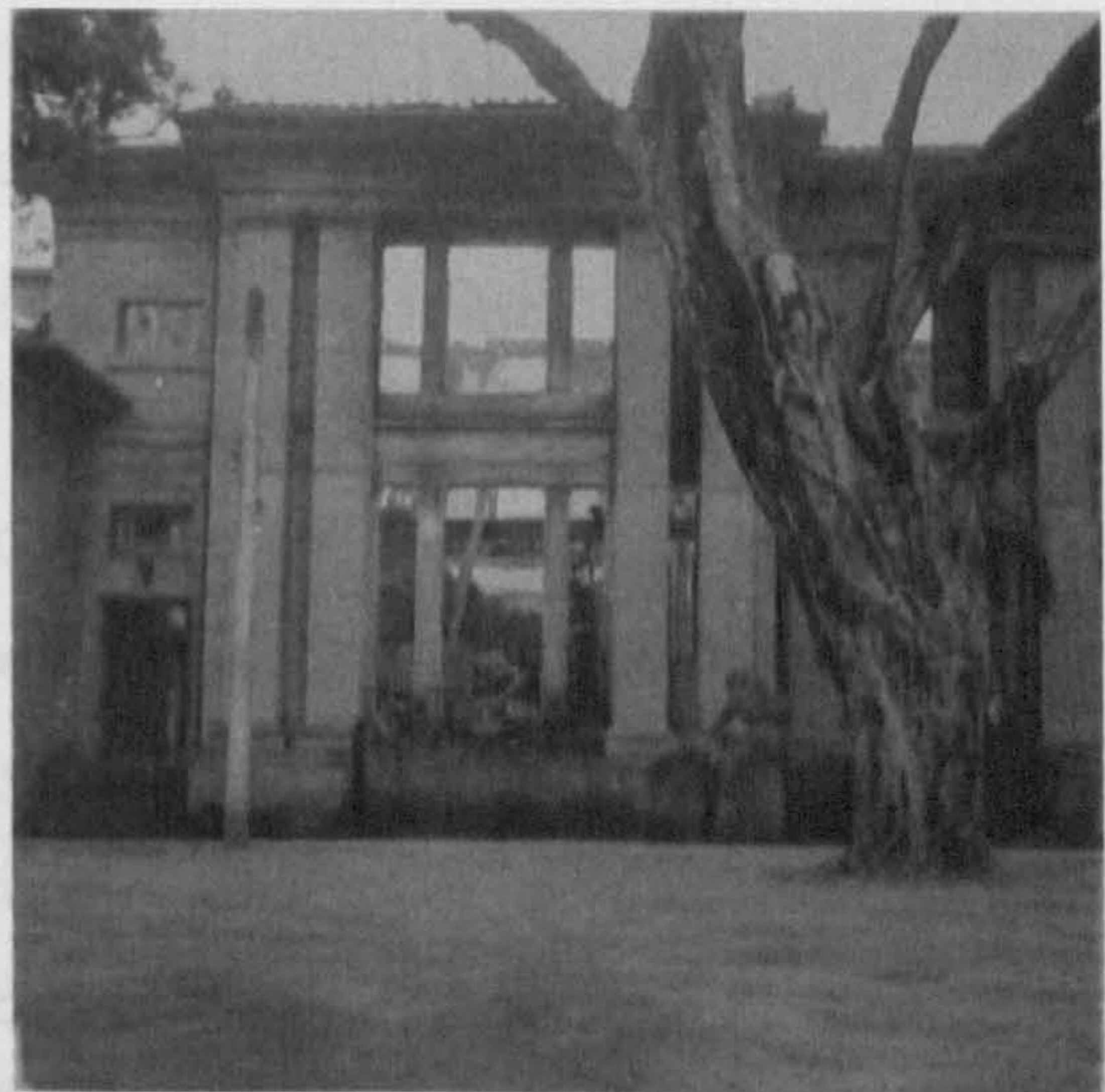
[ill.6: 24] CanTon Consulate, damaged Office building. Northwest angle. Source: 1948-1949, WORK 10/301, date: 1948
