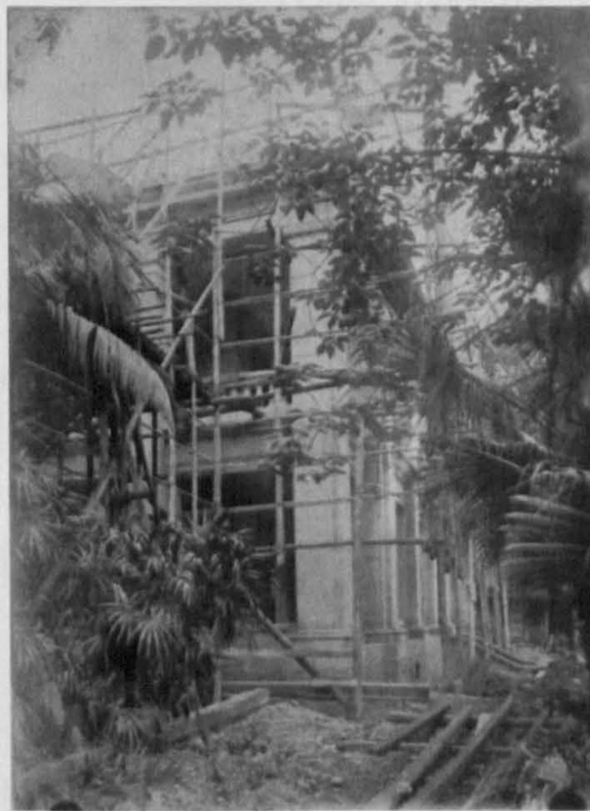
[ill.6: 16] CanTon Consulate, vice consul's residence under construction. Source: WORK 55/2, date 1924
