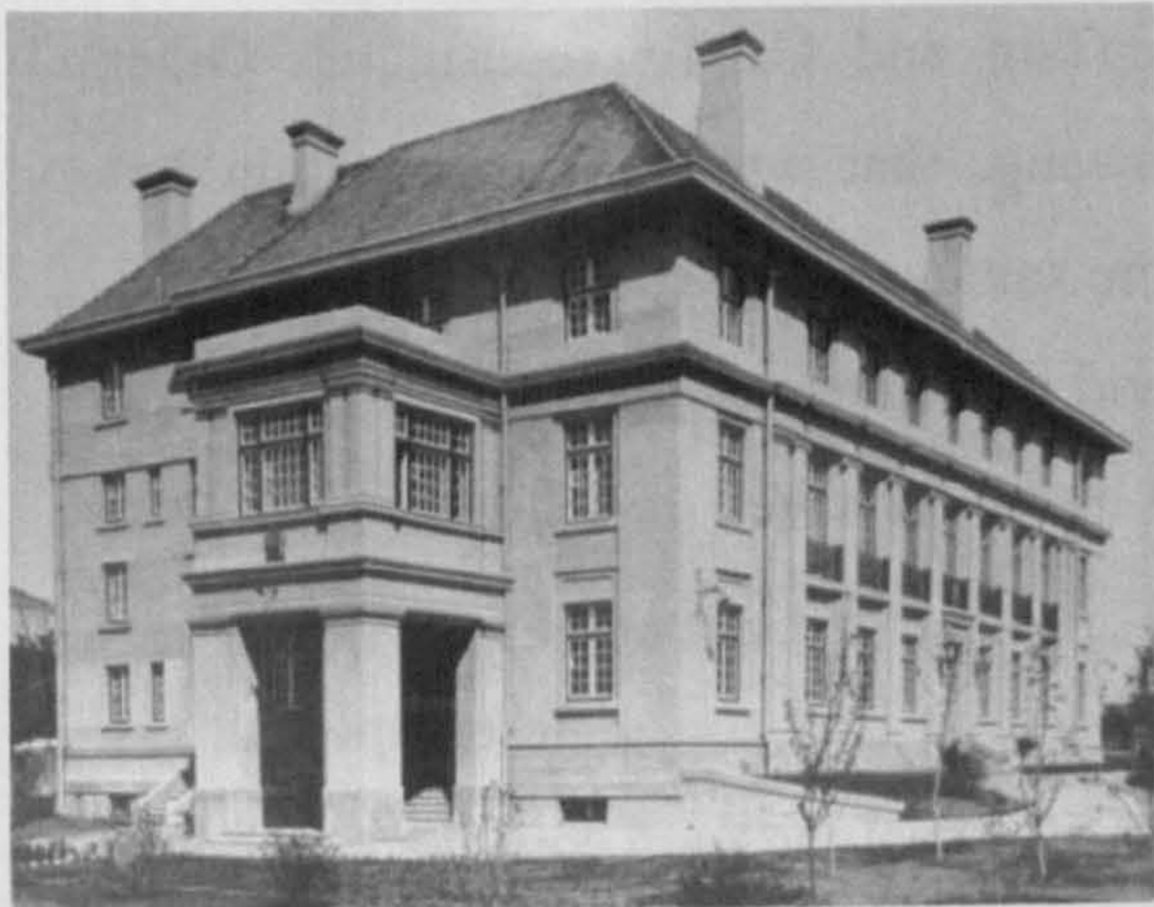
[ill.8: 11] Harbin Consulate, consul's residential entrance.
