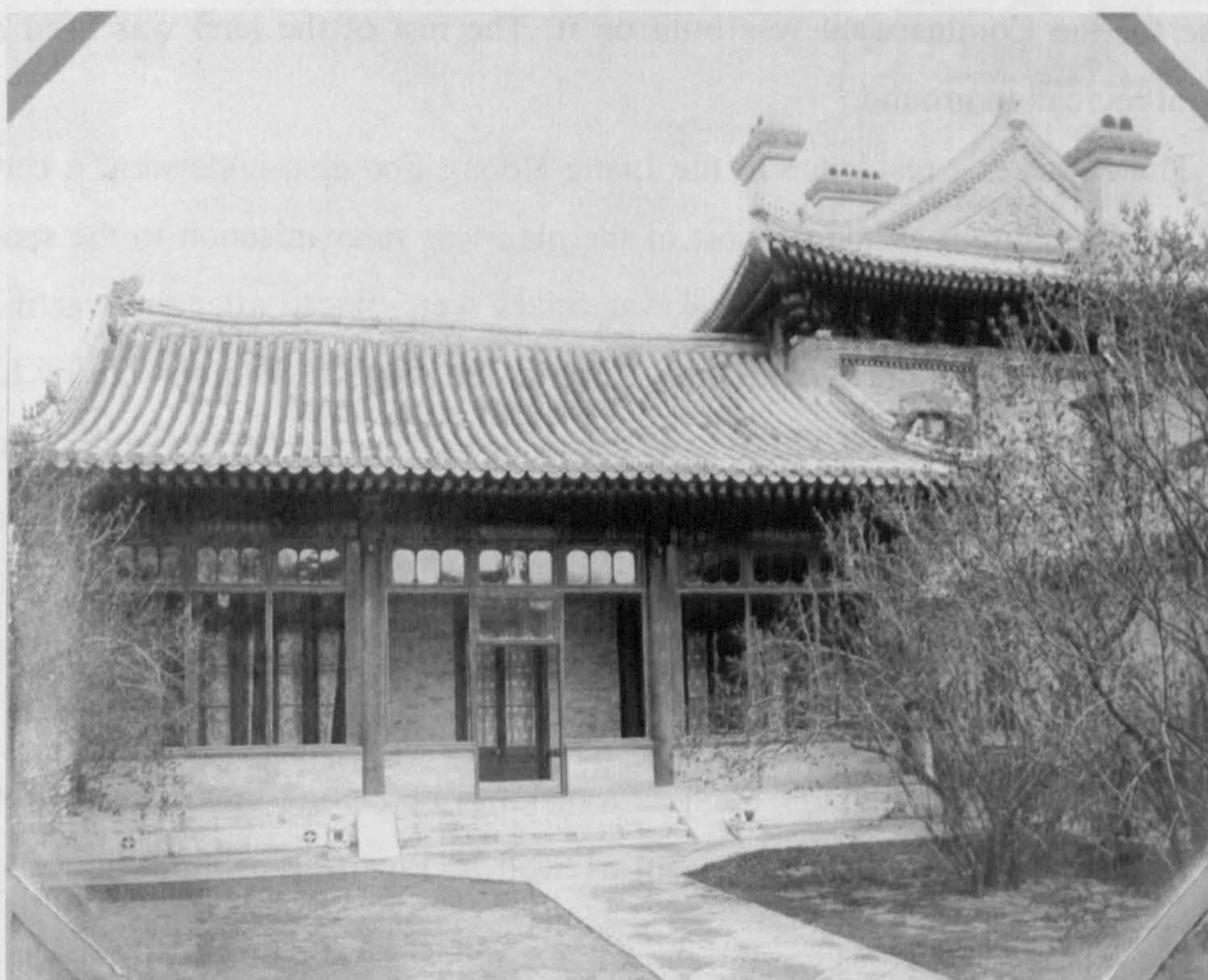
[ill.4: 6] PeKing Legation, Minister's residence. The two-storey building is the extension of the residence.
