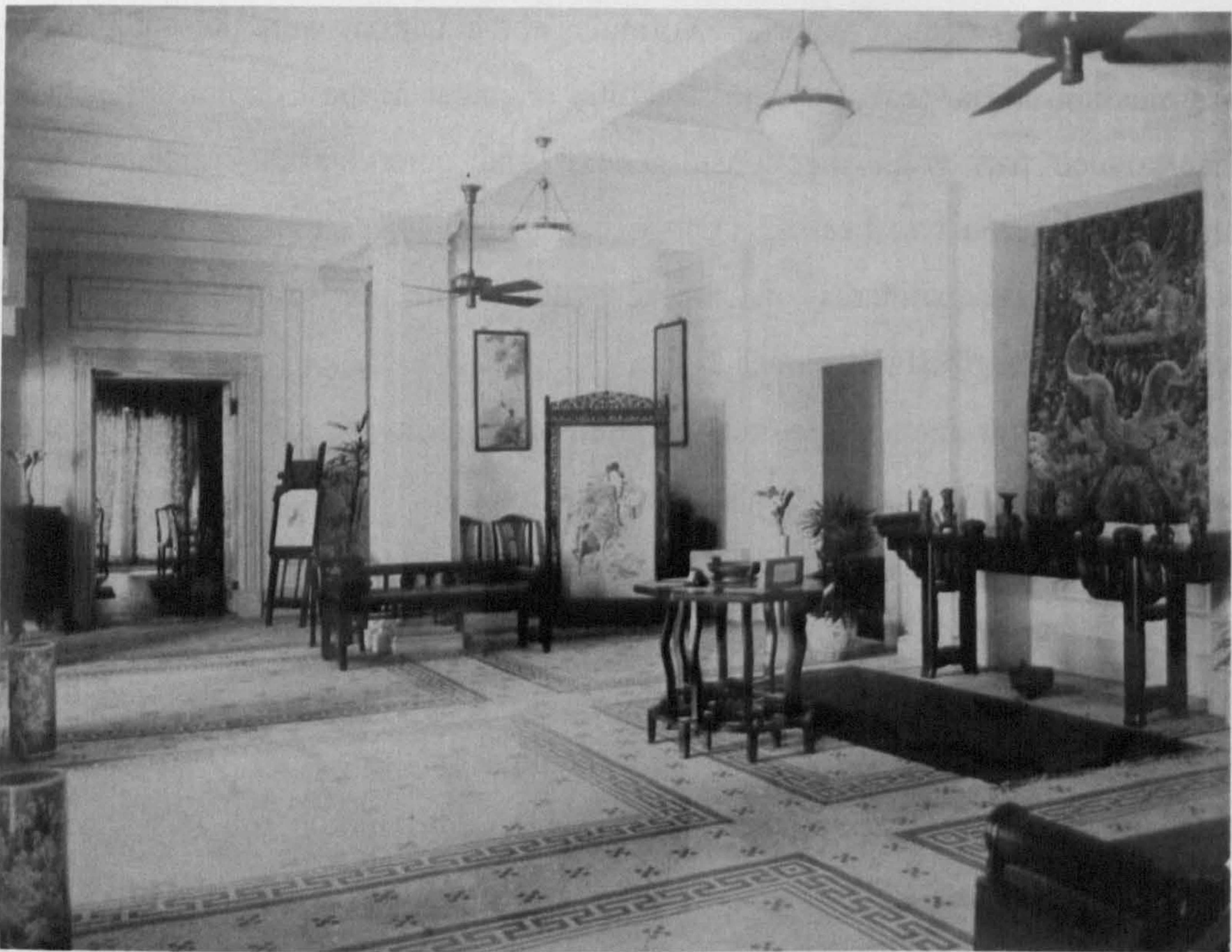
[ill.6: 22] CanTon Consulate, hall of Consul-General's house. It shows electric installations, lights and ceiling fans. Chinese arts of ordinary standard are also used to show the tastes of the consular officials.
