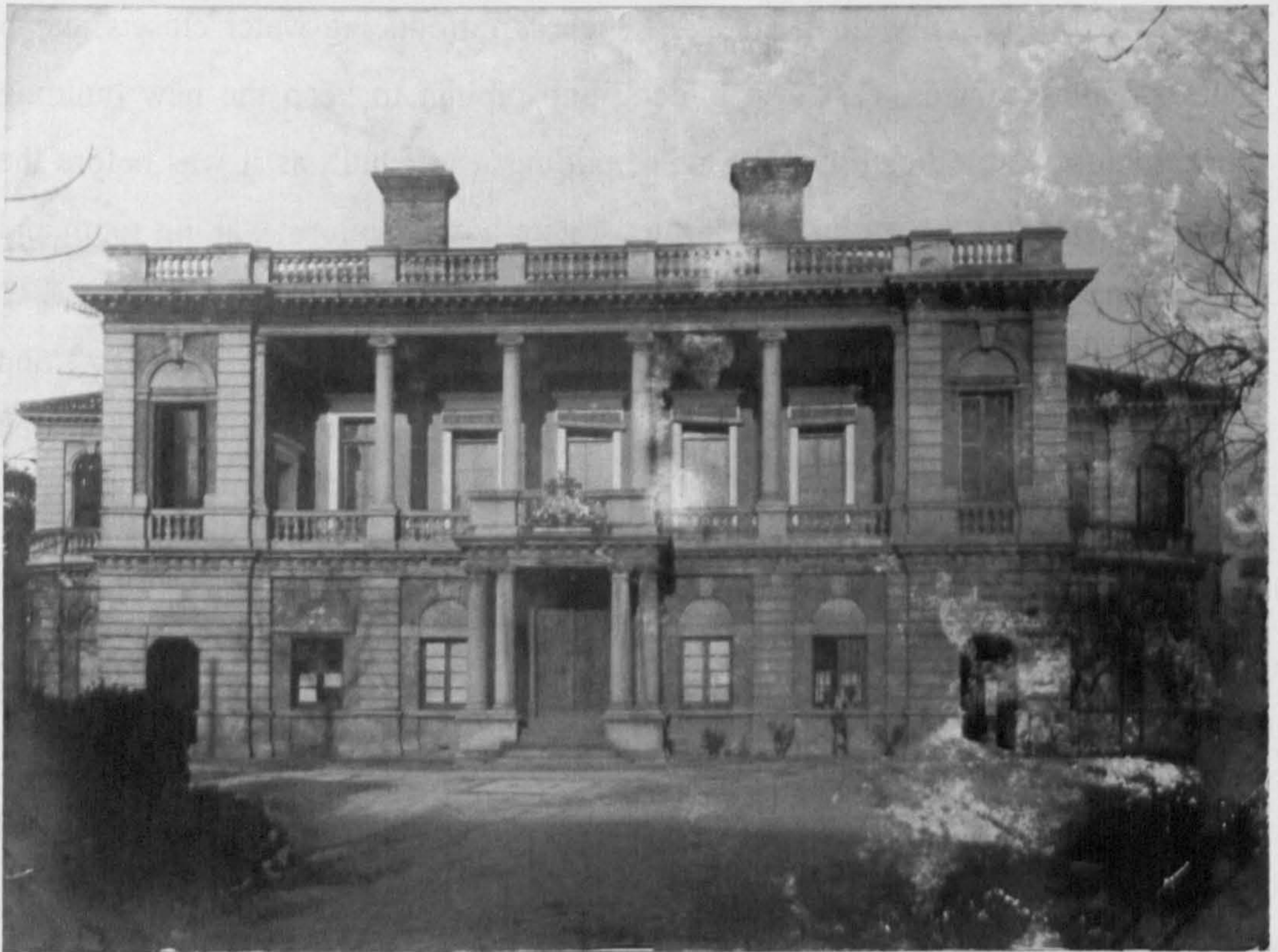
[ill.5: 6] ShangHai Consulate, front elevation of Supreme Court, facing west. Source: WORK 55/3, date: 1911
