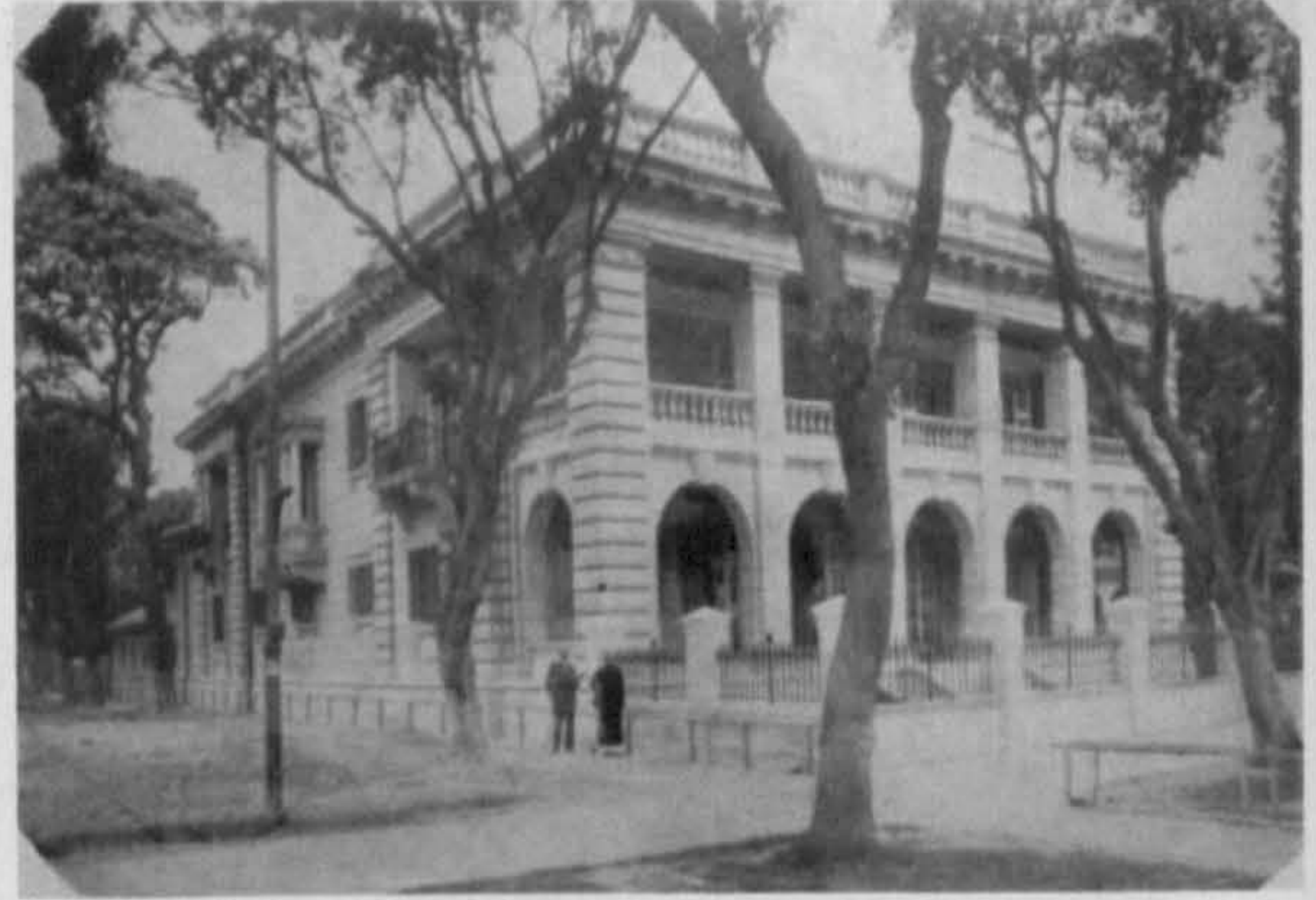
[ill.6: 20] CanTon Consulate, south and west elevation of Consul-General's residence.
