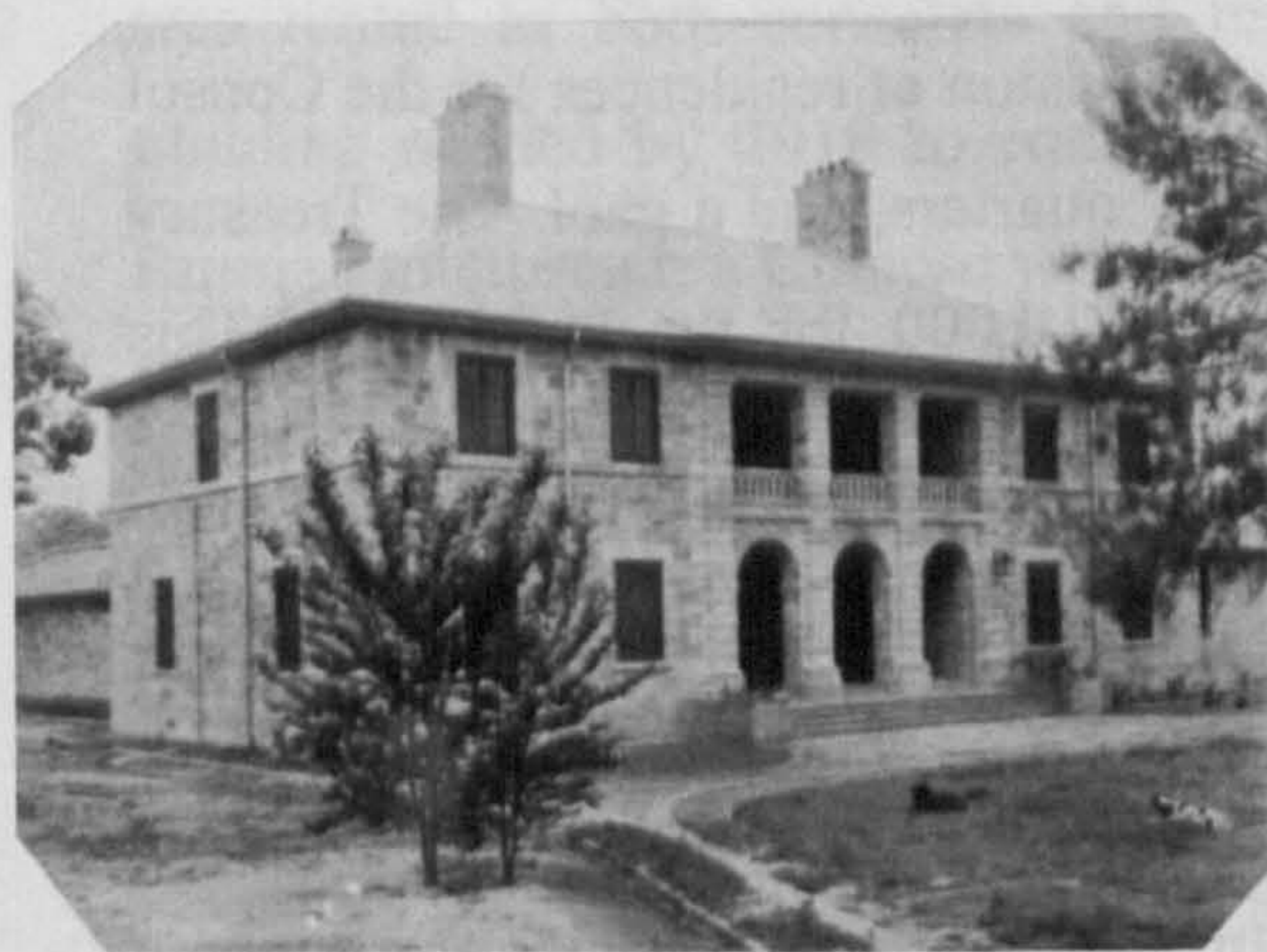
[ill.8: 7] TengYueh Consulate, front elevation of Consul's house.
