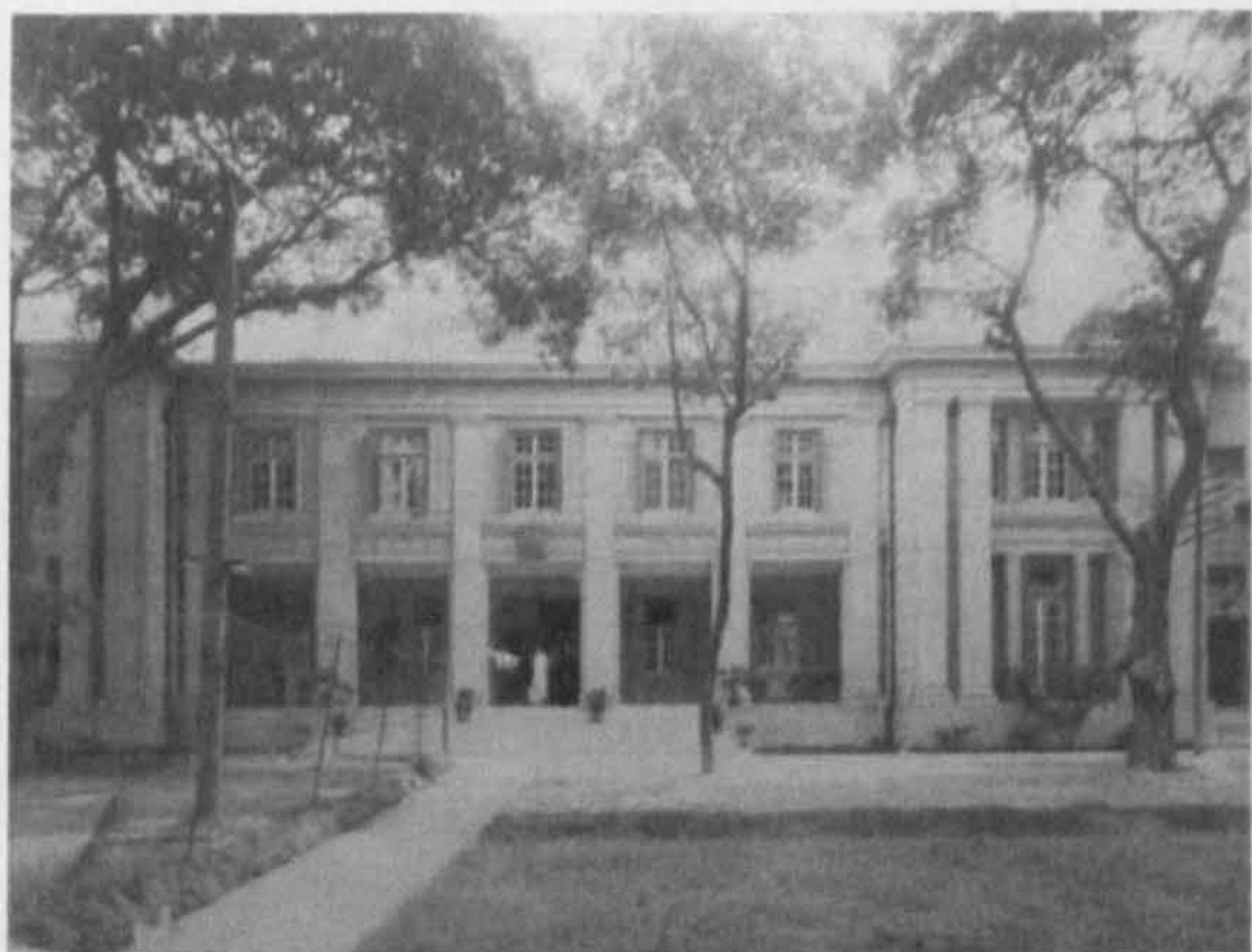
[ill.6: 11] CanTon Consulate, north and public façade of Office & Assistants' quarters. Source: WORK 55/2, date 1924
