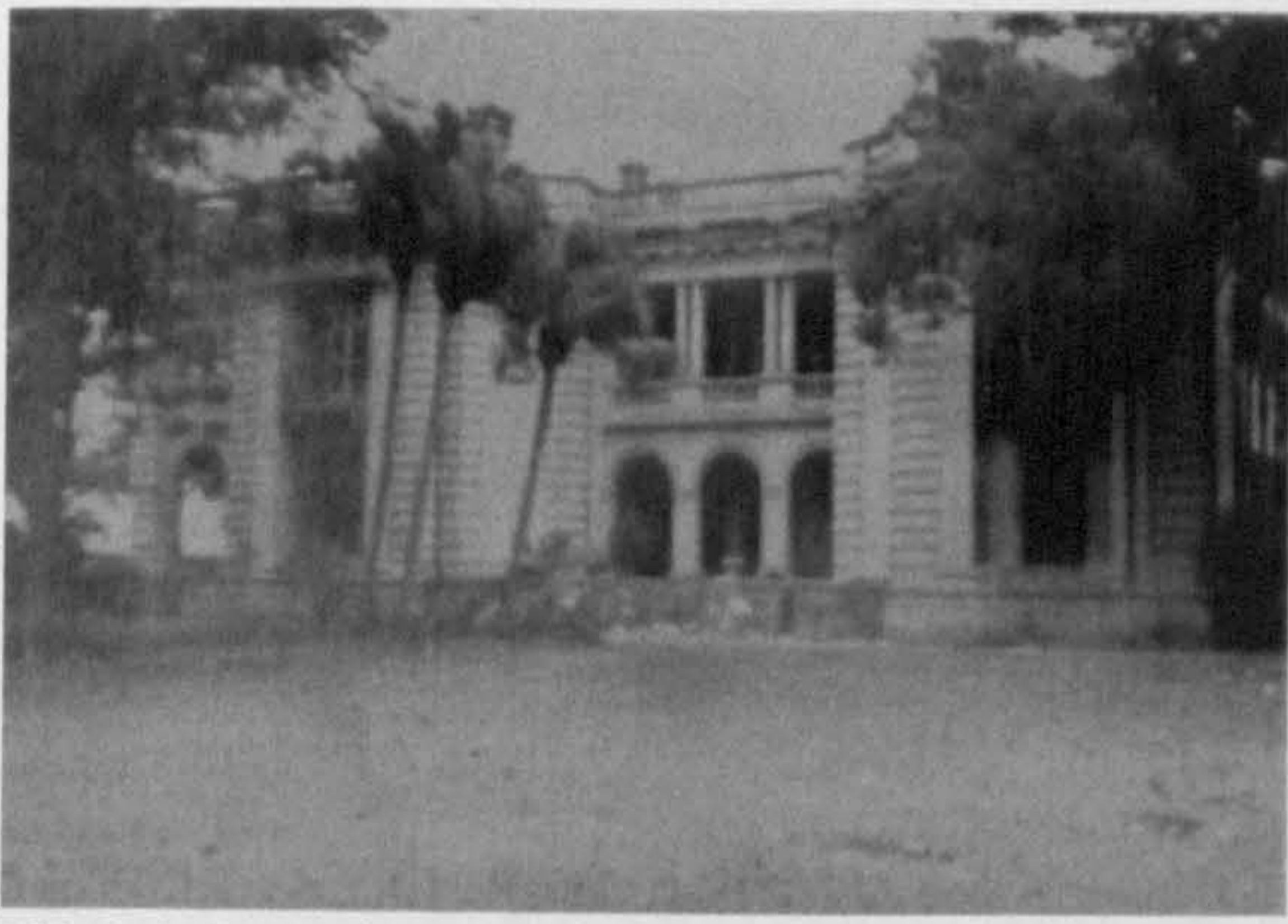
[ill.6: 26] CanTon Consulate, damaged Consul-General's house. Front façade. Source: 1948-1949, WORK 10/301, date: 1948
