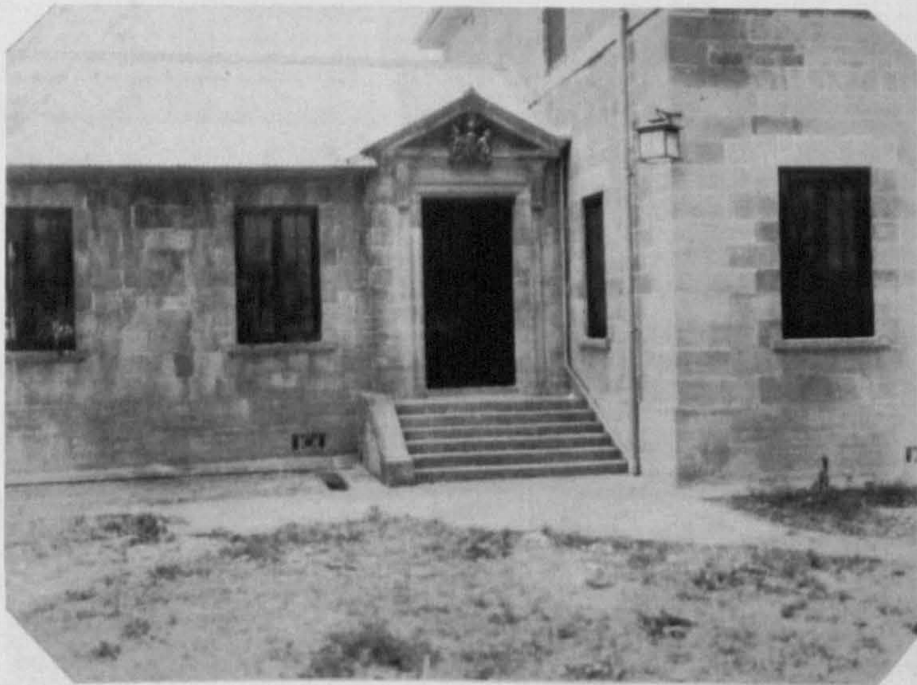
[ill.8: 16] TengYueh Consulate, office entrance. Source: WORK 55/3, date: 1911-1935
