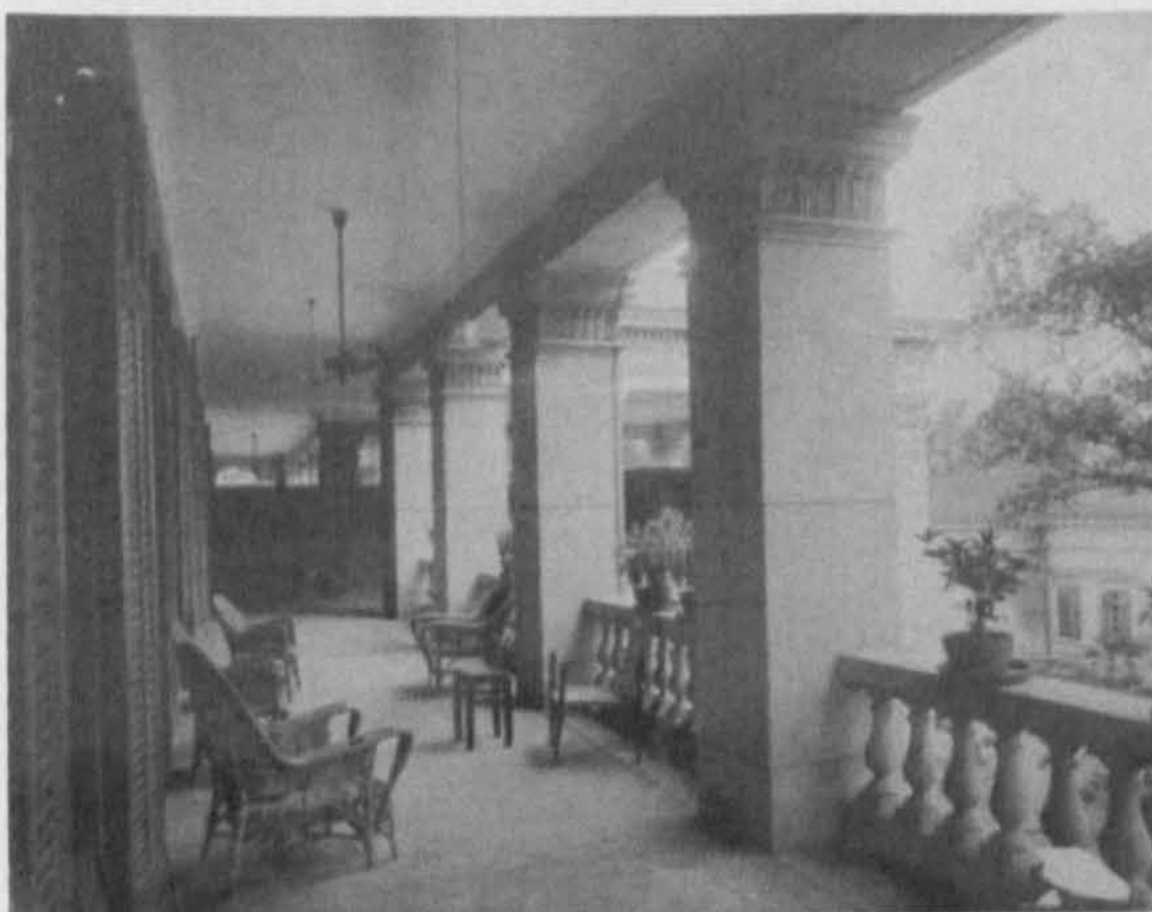
[ill.6: 13] CanTon Consulate, south verandah of assistants' quarters. Source: WORK 55/2, date: 1924
