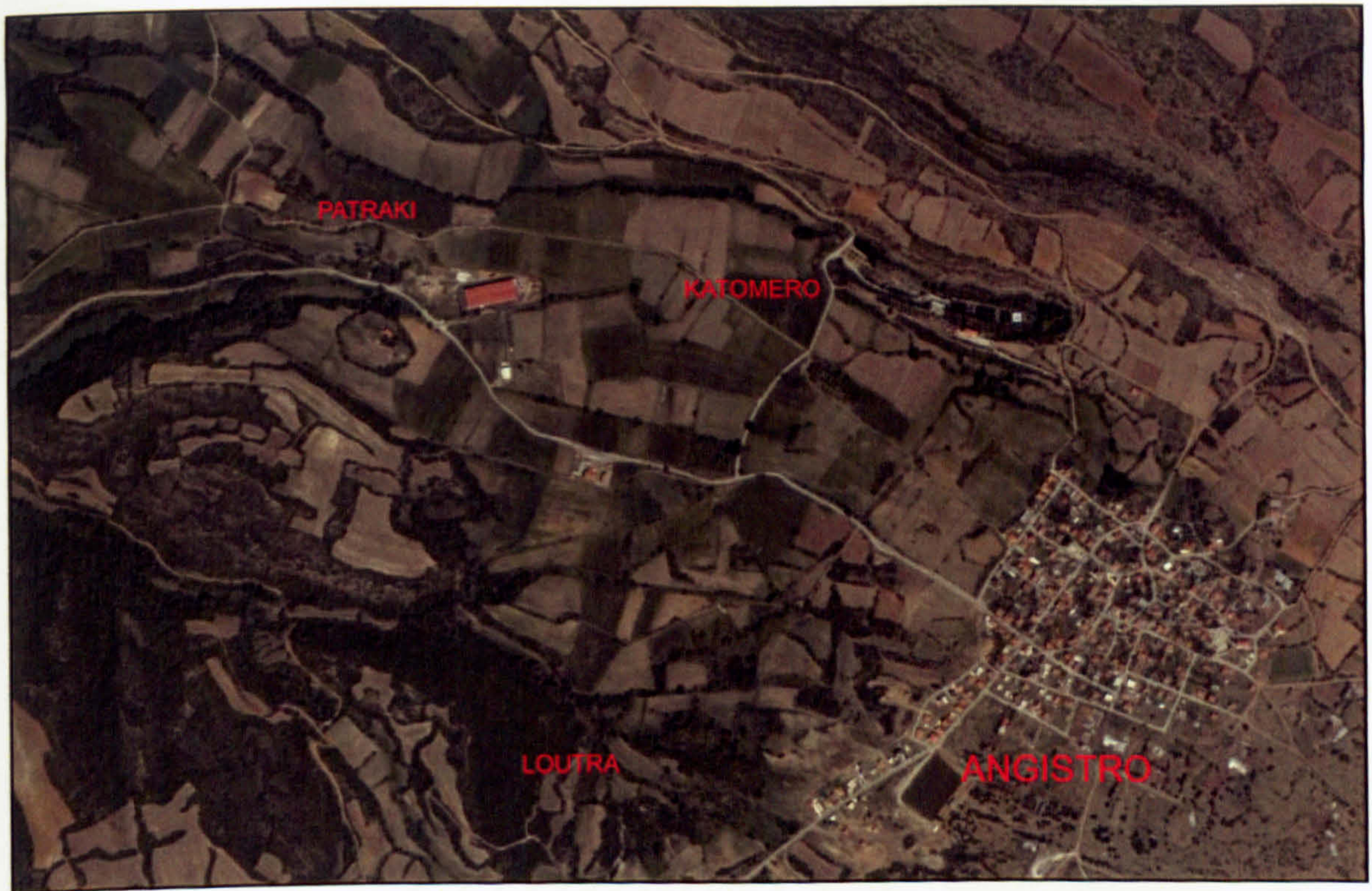
Figure 5.20 Satellite image of Angistro and the major smelting sites (source: Google Earth)
