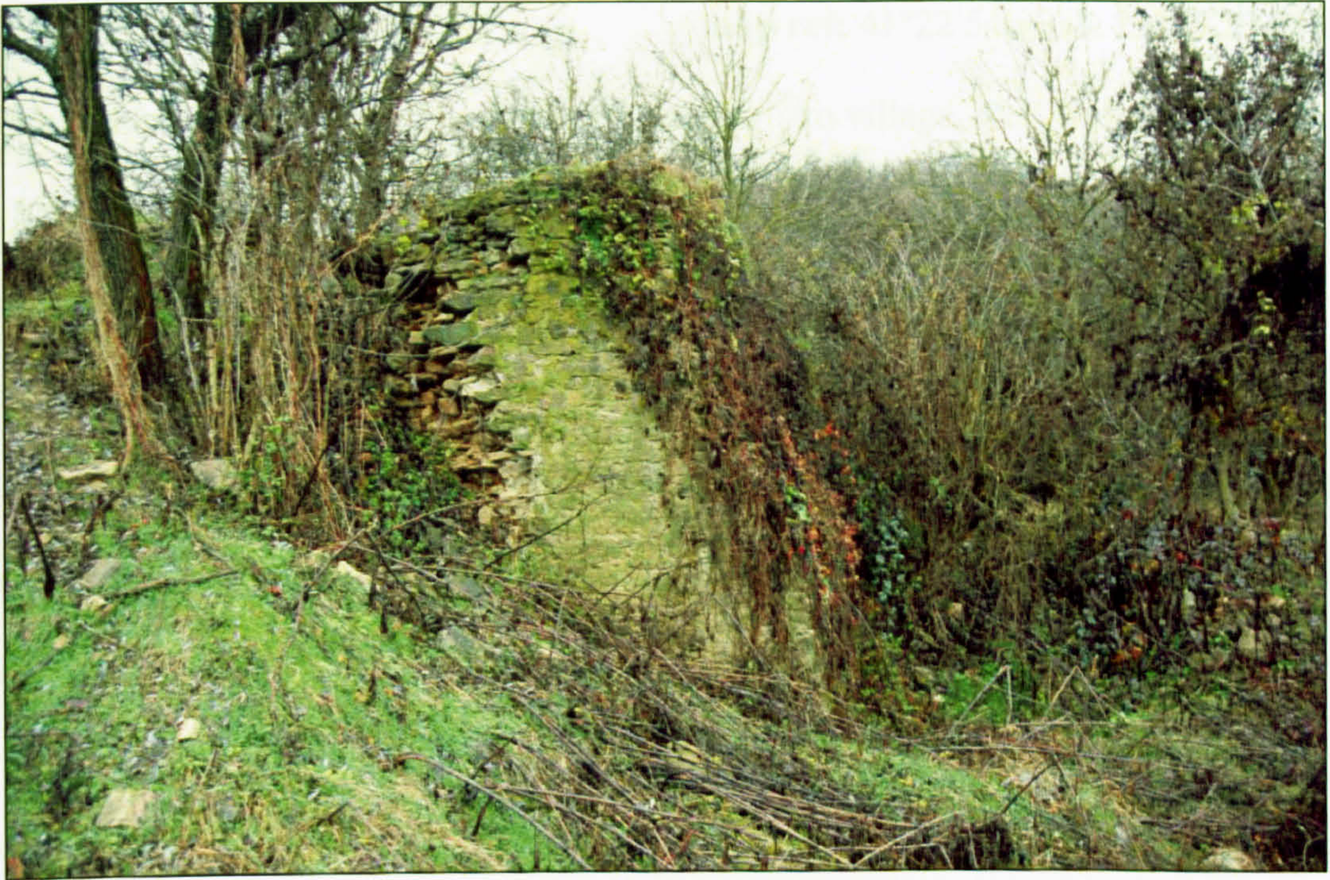
Figure 5.18 The watermill tower, view from the southeast
