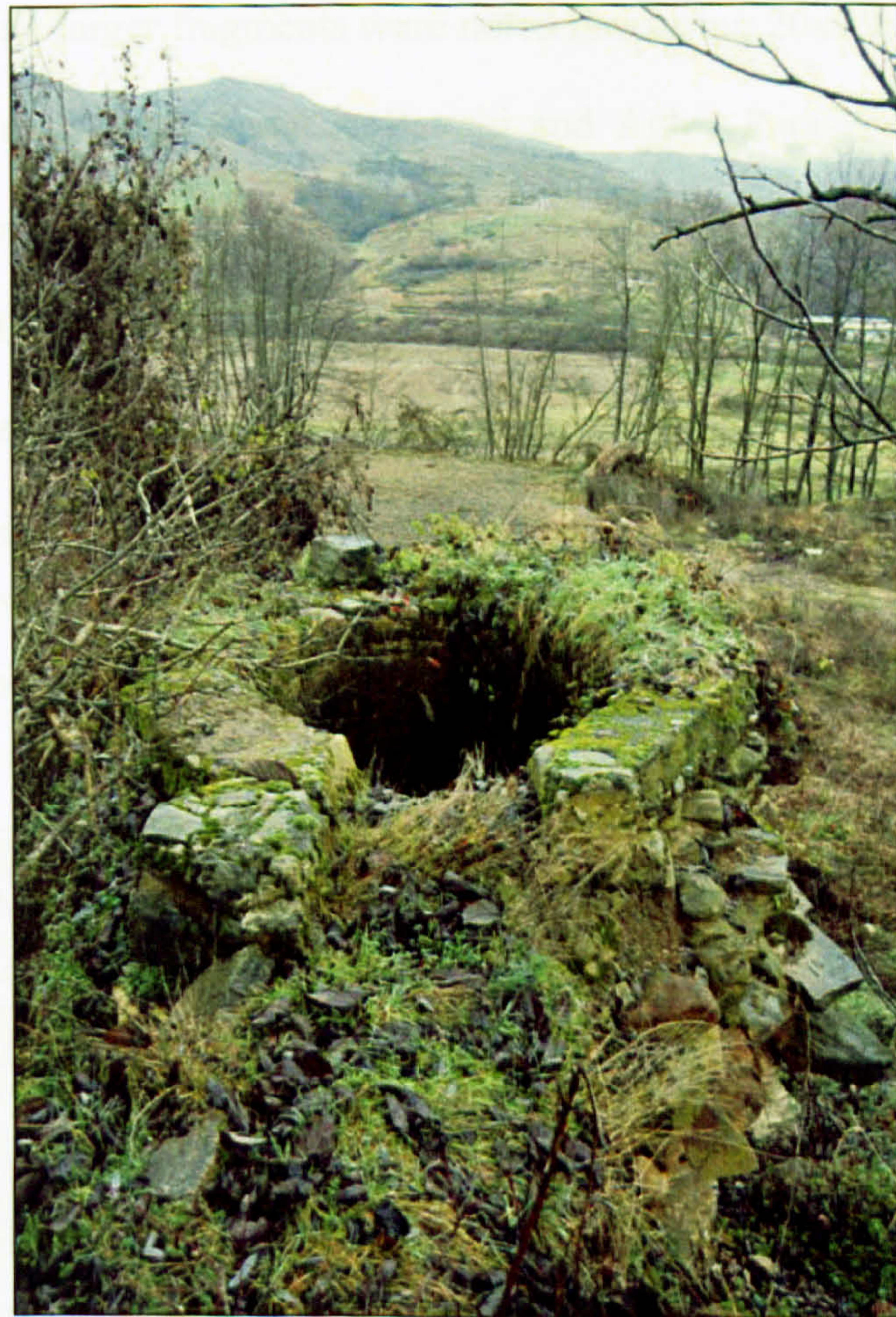
Figure 5.19 The stone-built hopper of the watermill
