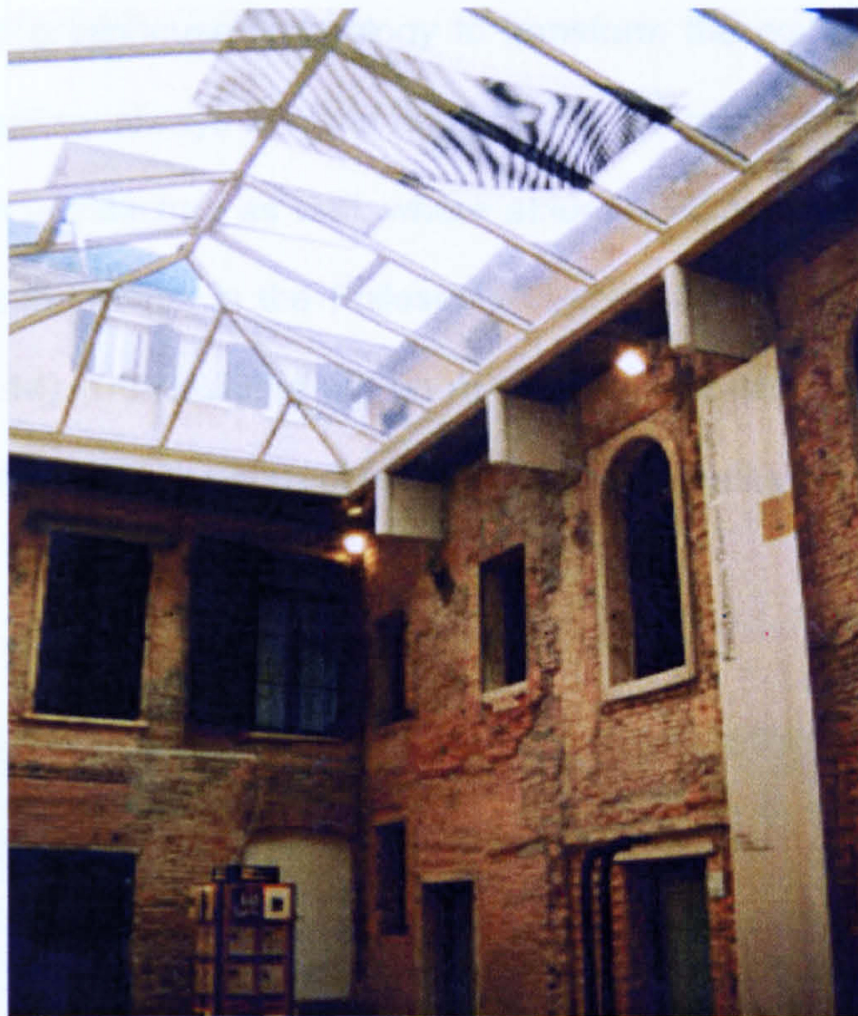
Figure 2. 43: Passive solar retrofit in the building of Fondazione Querini Stampalia, in Venice.
