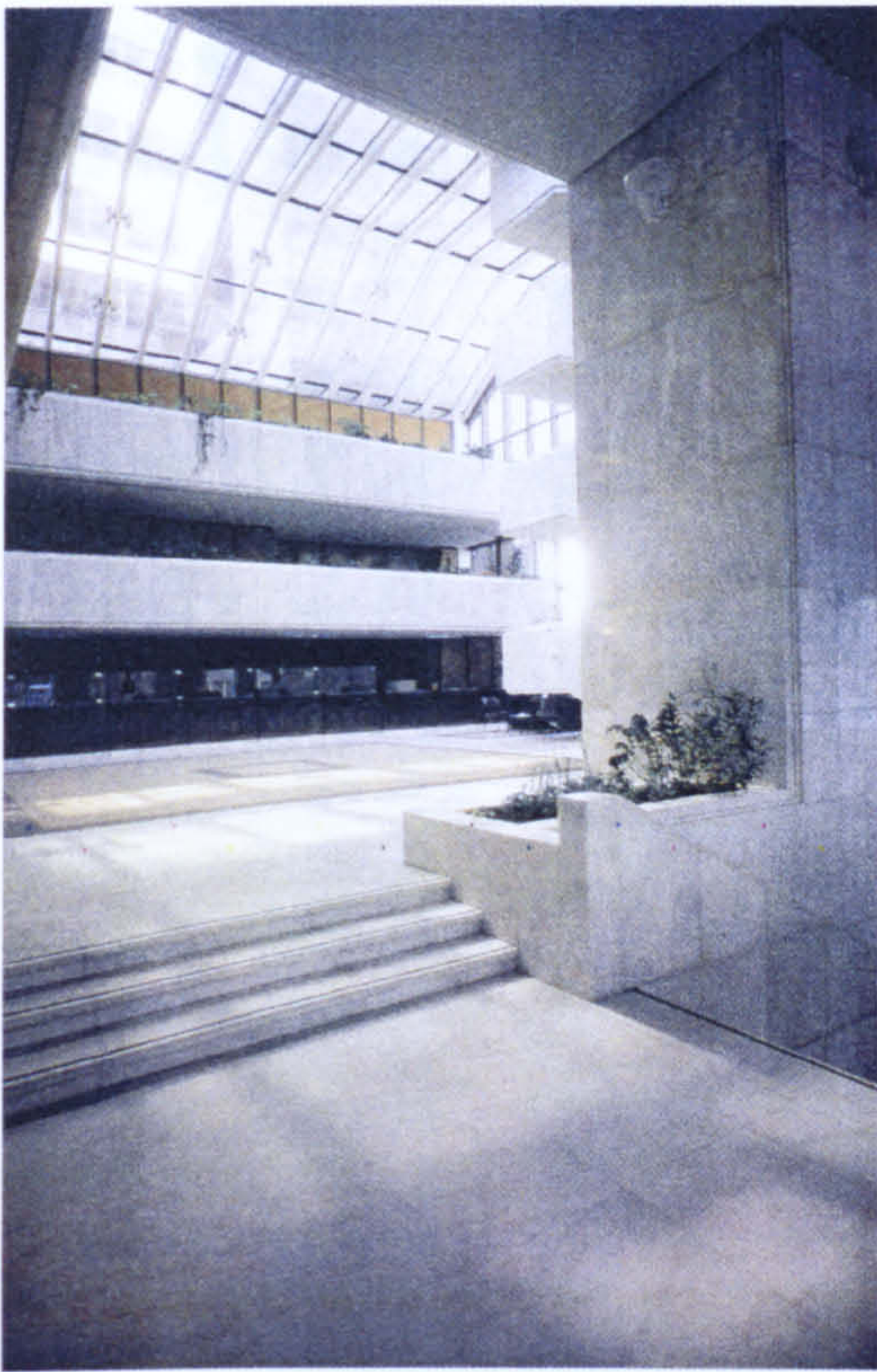
Figure 2. 32: An example of an attached glazed space. Administration headquarters building of the Credit Bank in Athens
