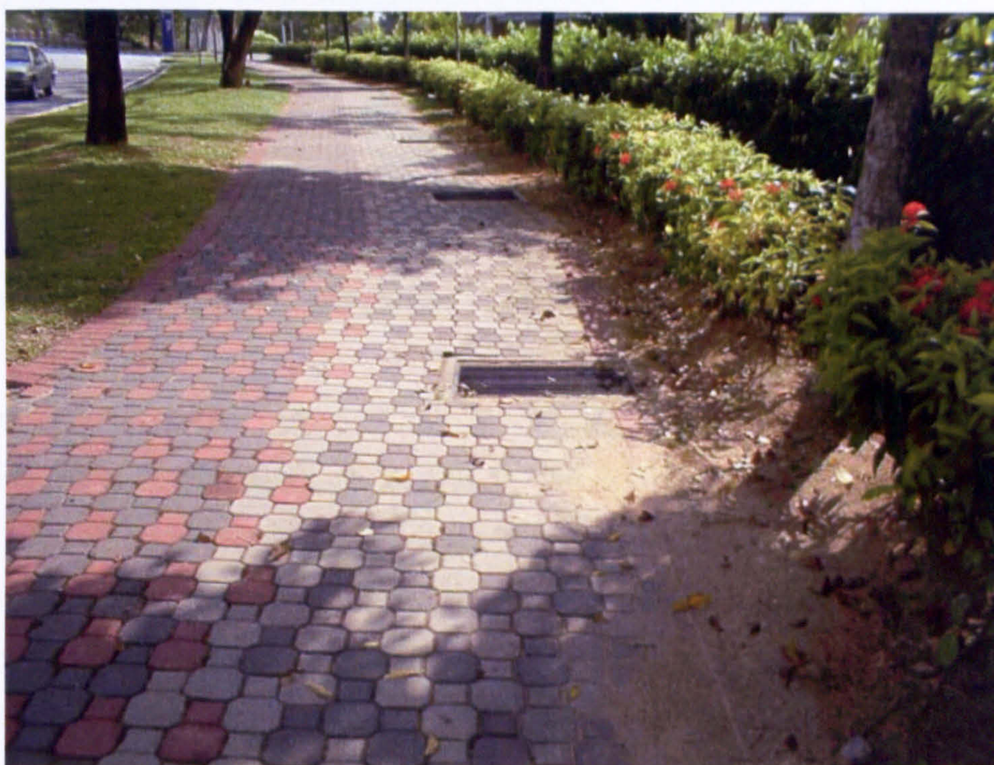
Figure 5.2.12: Porous pavement used on the pedestrian walkway.
