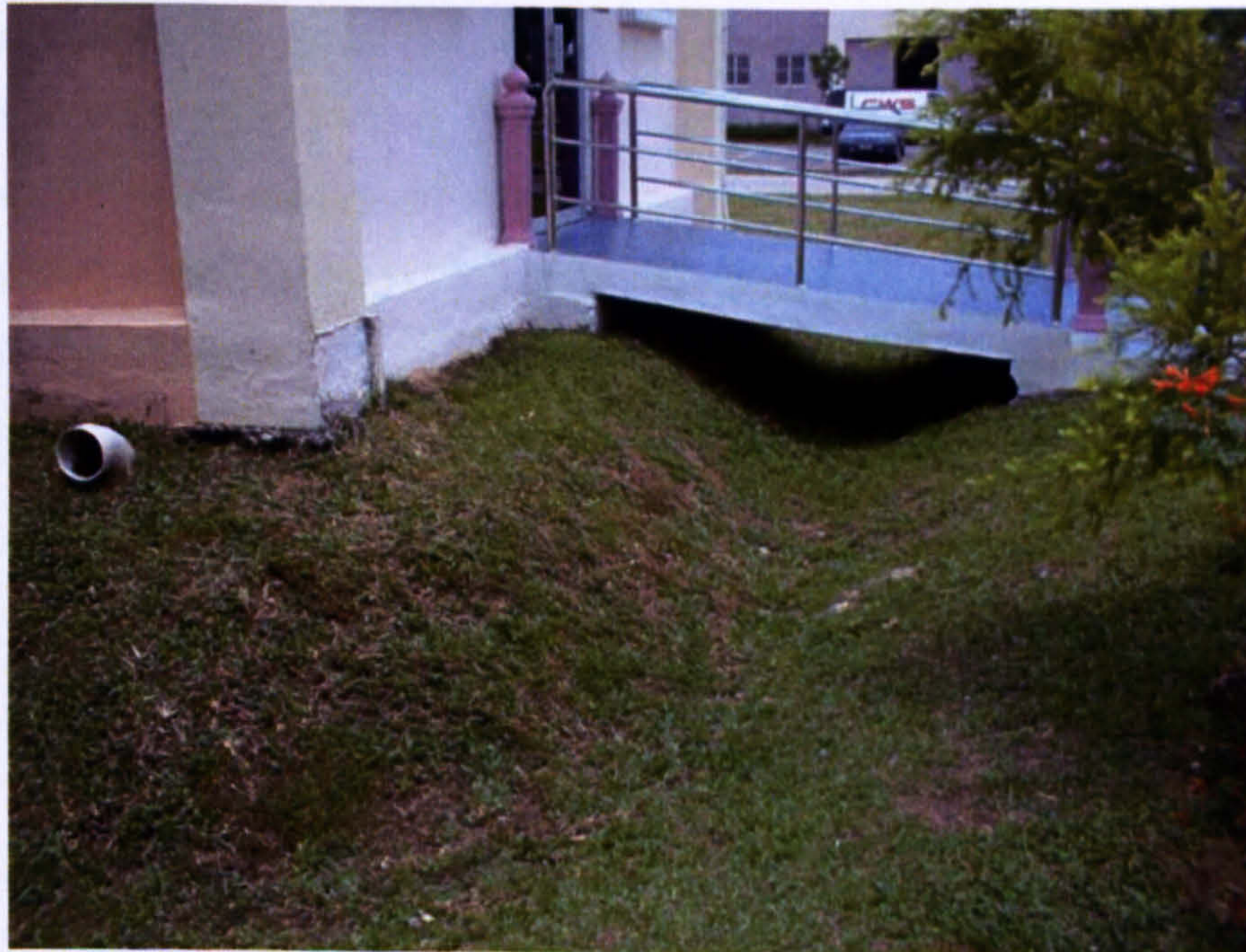
Figure 5.3.6: The perimeter swale surrounding the REDAC office in the USM campus
