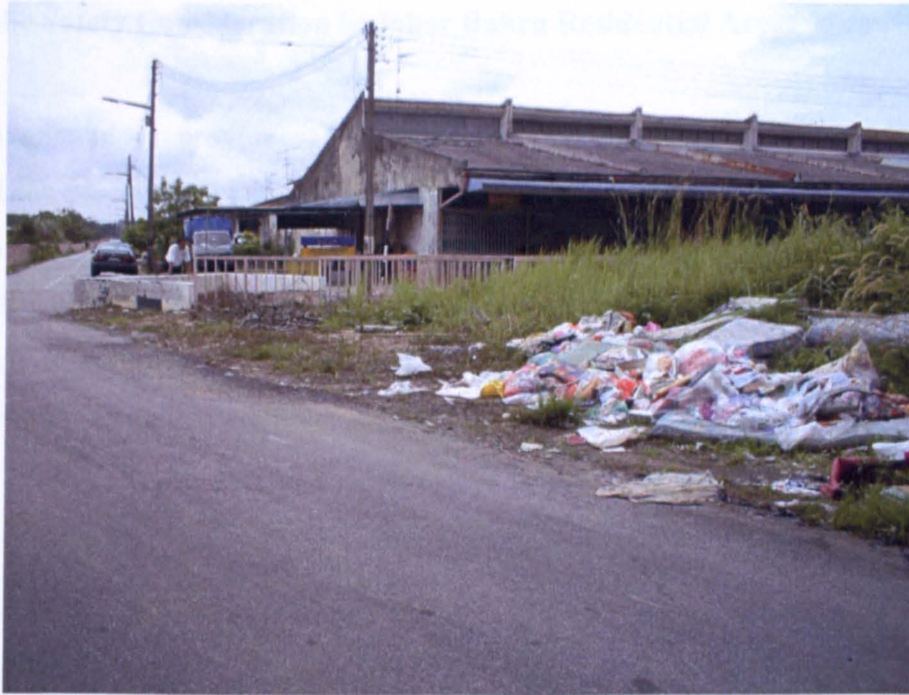
Figure 5.1.10: Waste dumping by irresponsible residents in drainage reserves in a residential area in JB
