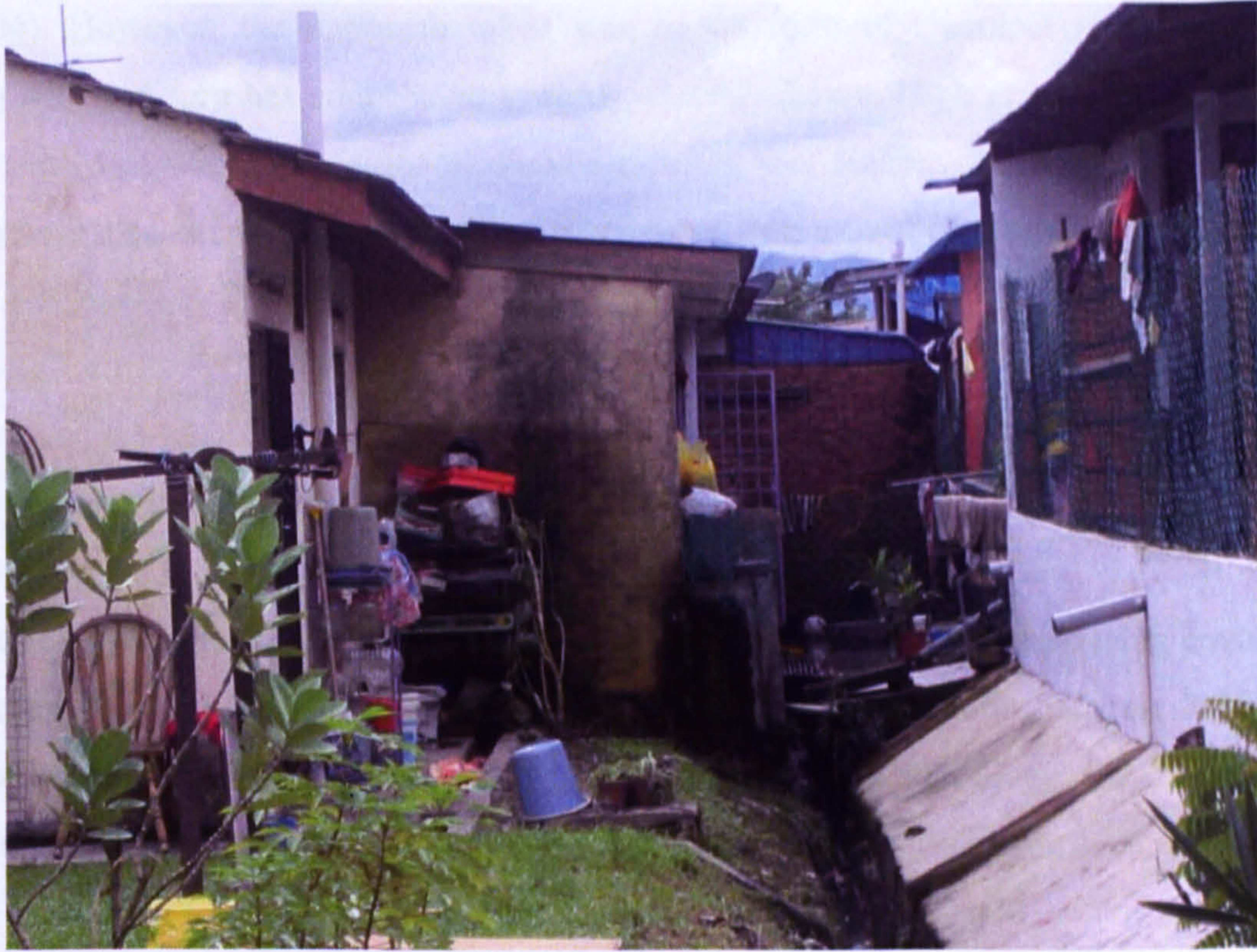
Figure 2.1.5: These two blocks of terrace houses were not provided with a back-lane and, to make matters worse, some renovation over the drainage systems.
