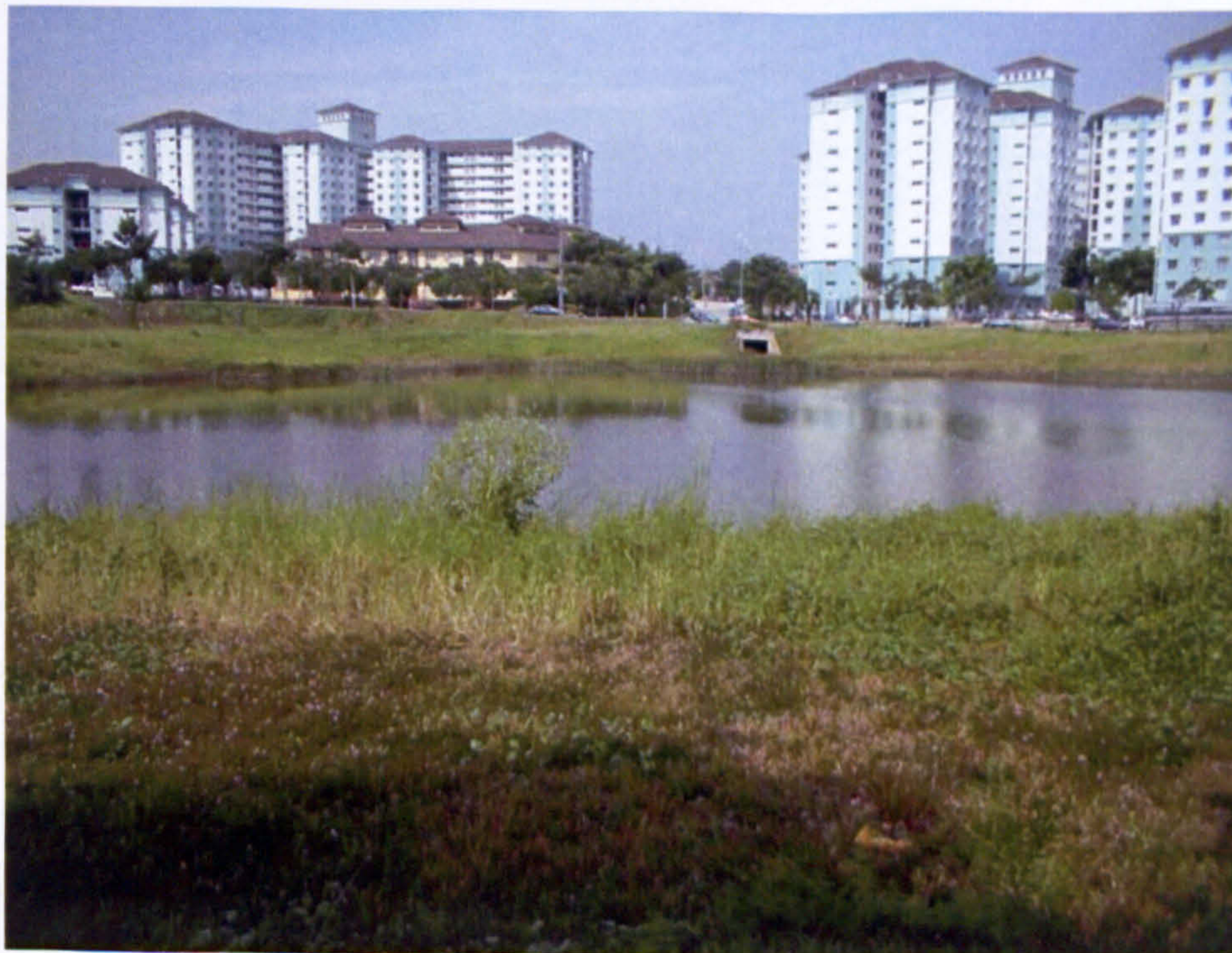
Figure 5.2.11: Wet pond in Putrajaya residential area.
