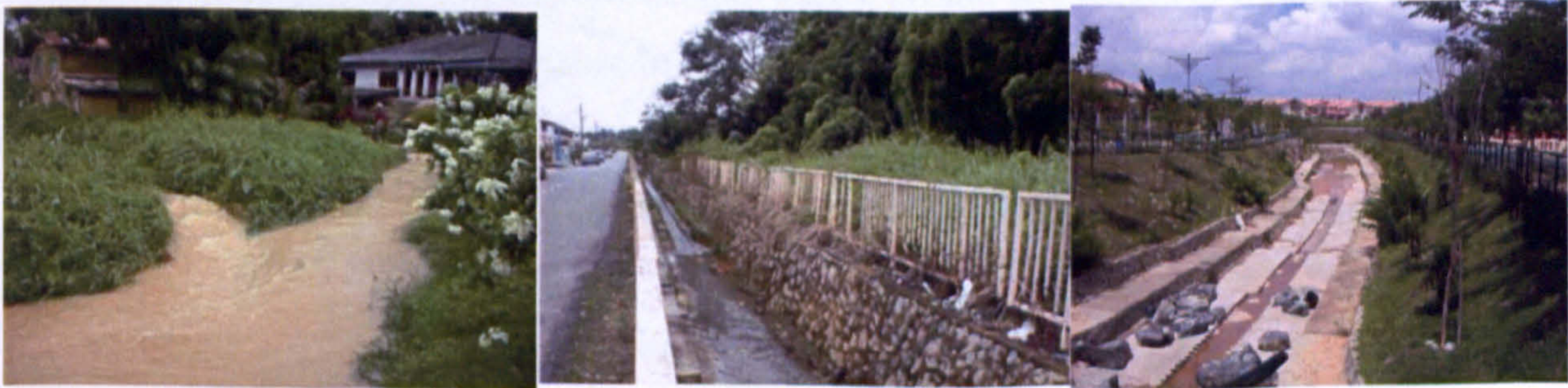
Figure 4.7.2: Drainage models in Malaysia – Natural swale (left), a conventional drainage (middle) and a drain in Putrajaya (right).
