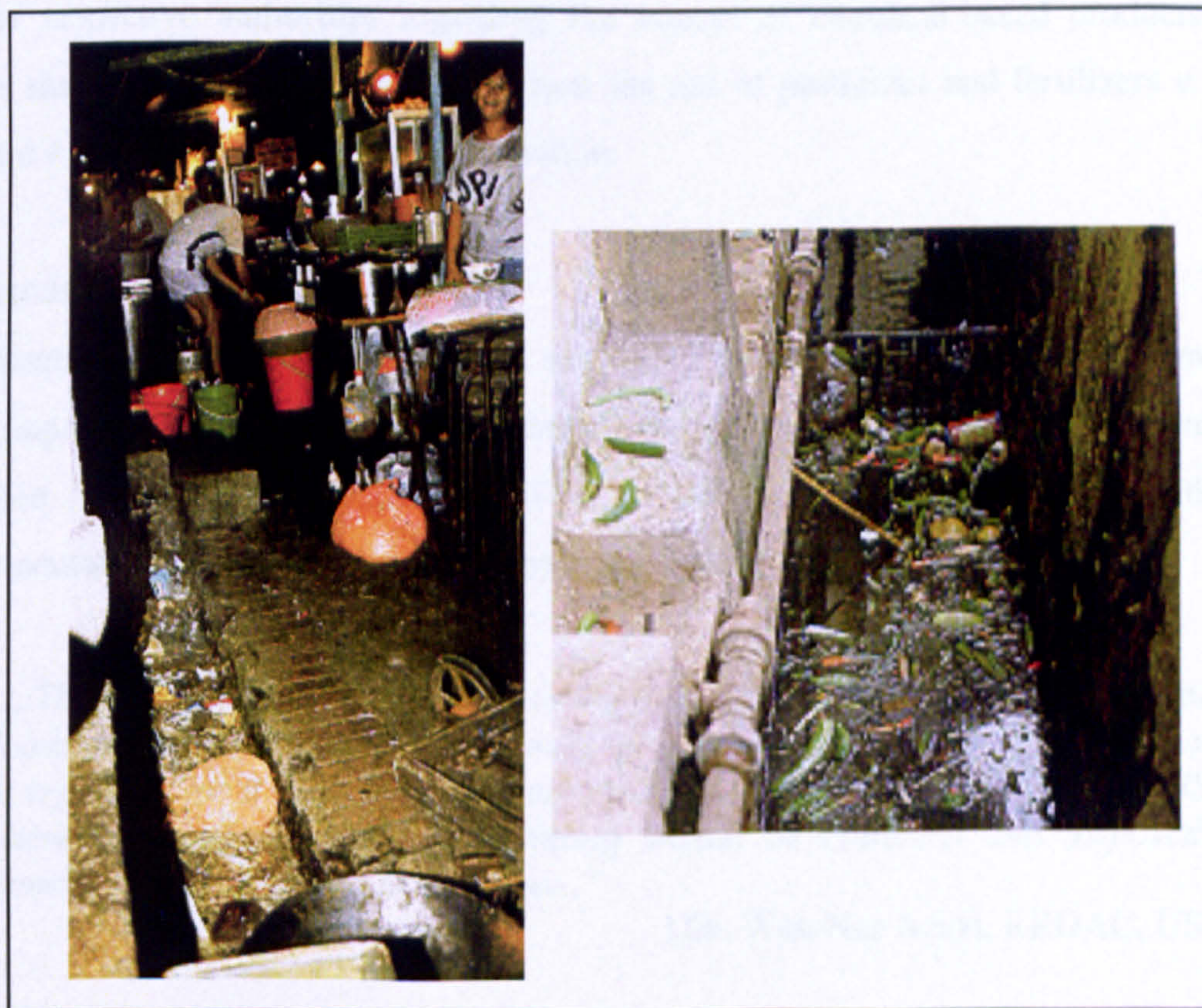
Figure 6.12.1: Waste from food stalls are dumped into the drainage systems (Source: DID webpage)
