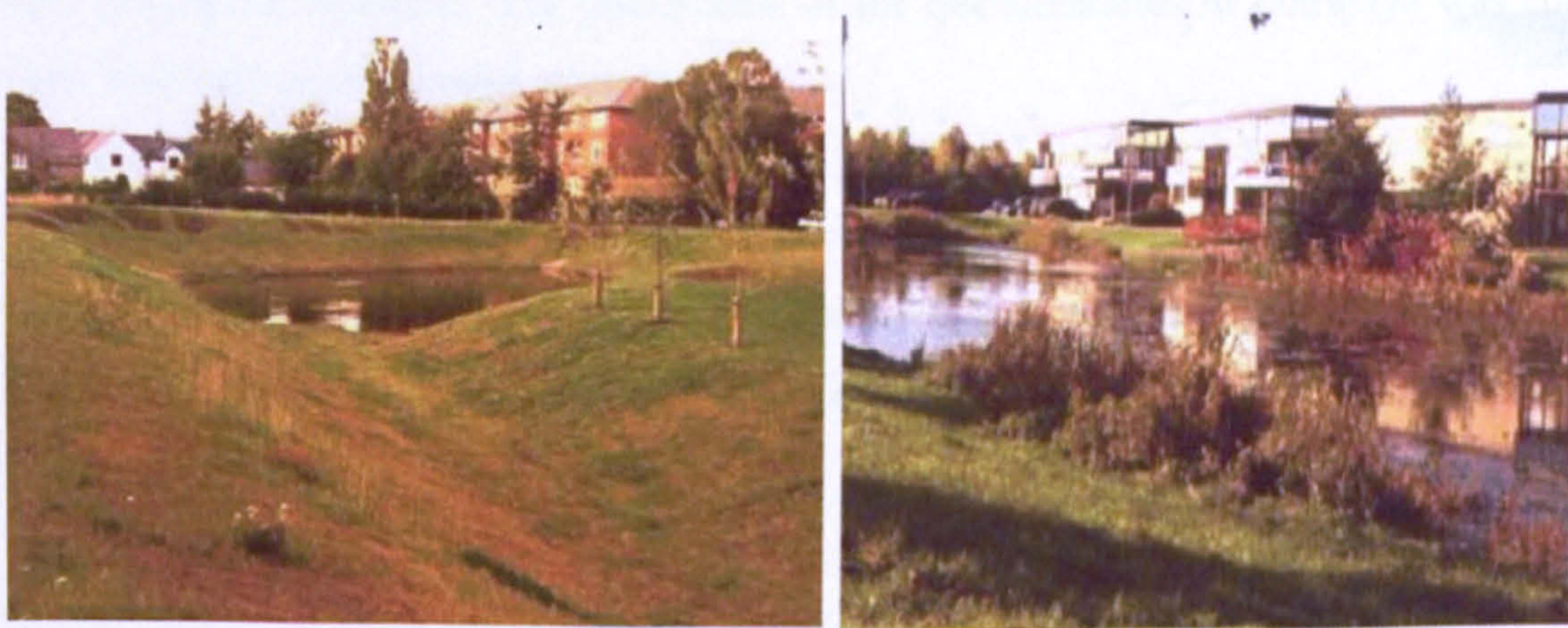
Figure 4.7.1: SUDS components as implemented in the UK – A combination used of pond and swale (left) and wetland (right)(Source: CIRIA)
