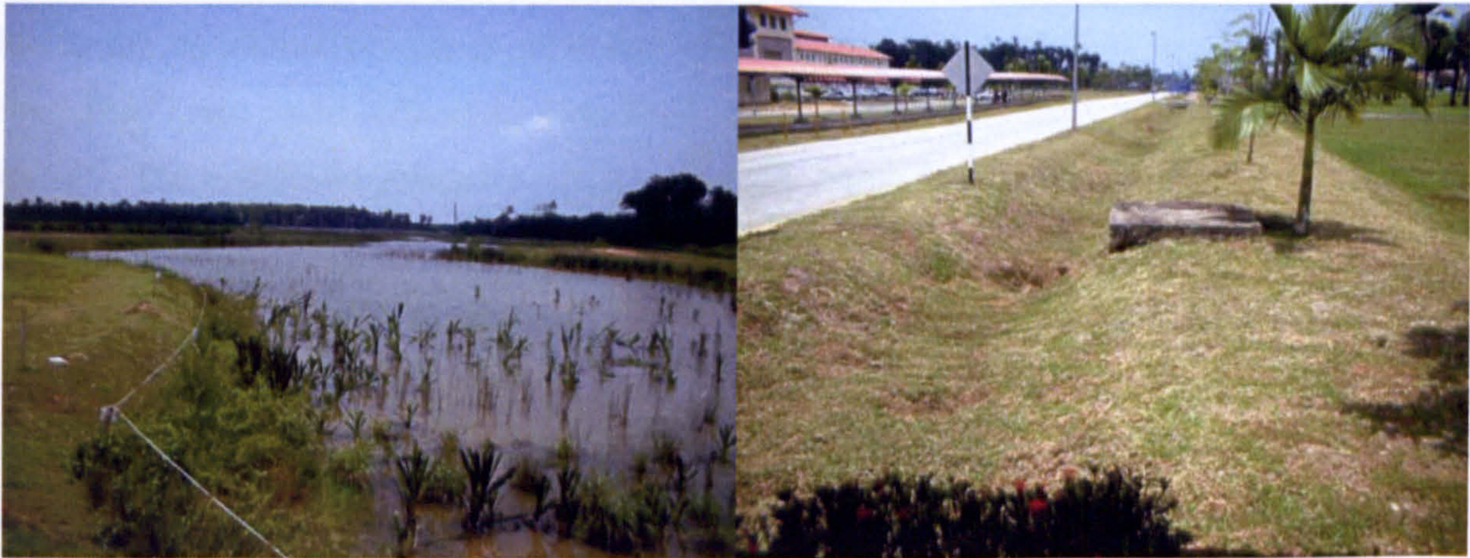
Figure 8.1.3: A constructed wetland and a swale in the USM Engineering campus.
