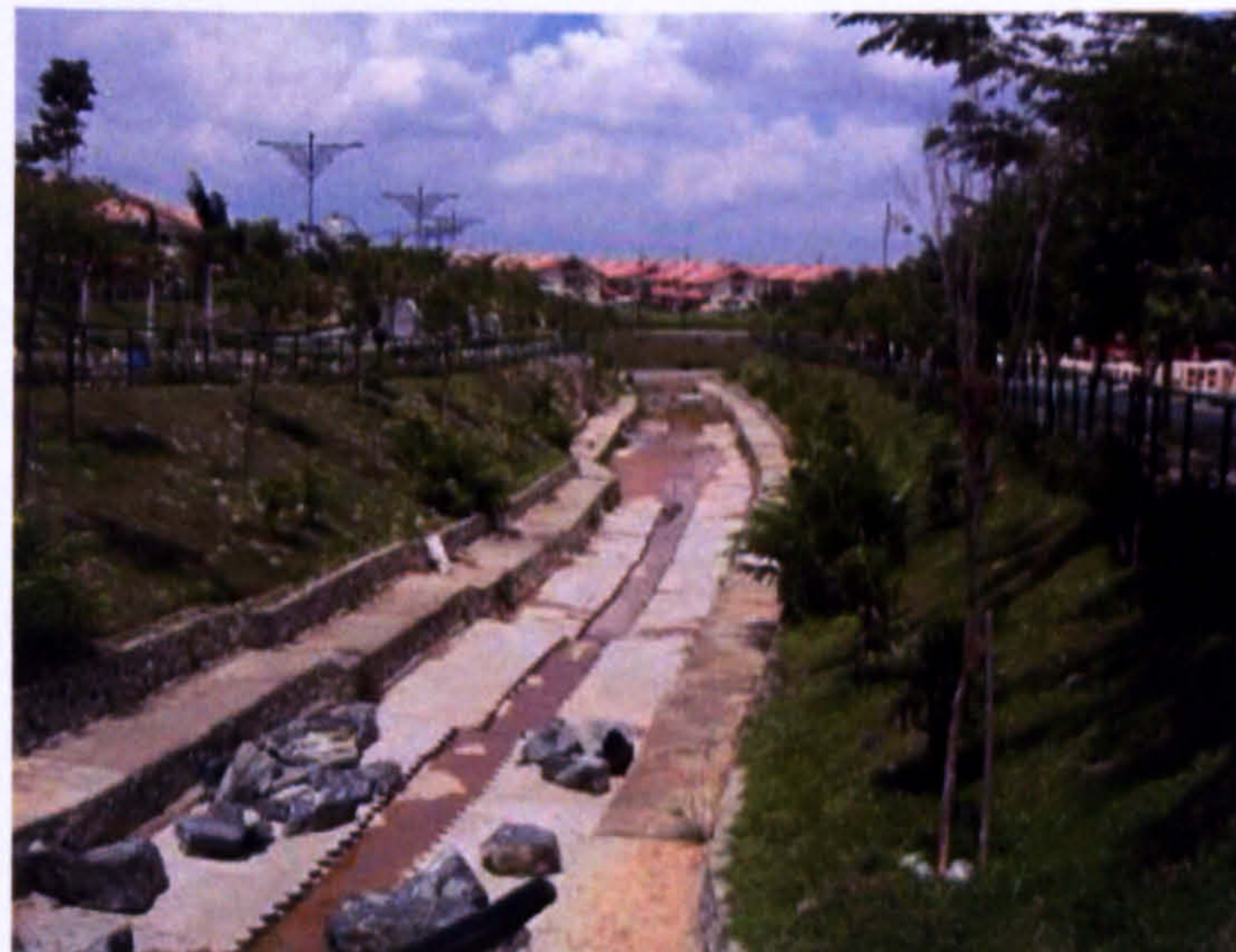
Figure 6.11.5: Image of Putrajaya Main Drain (Source: Researcher file)
