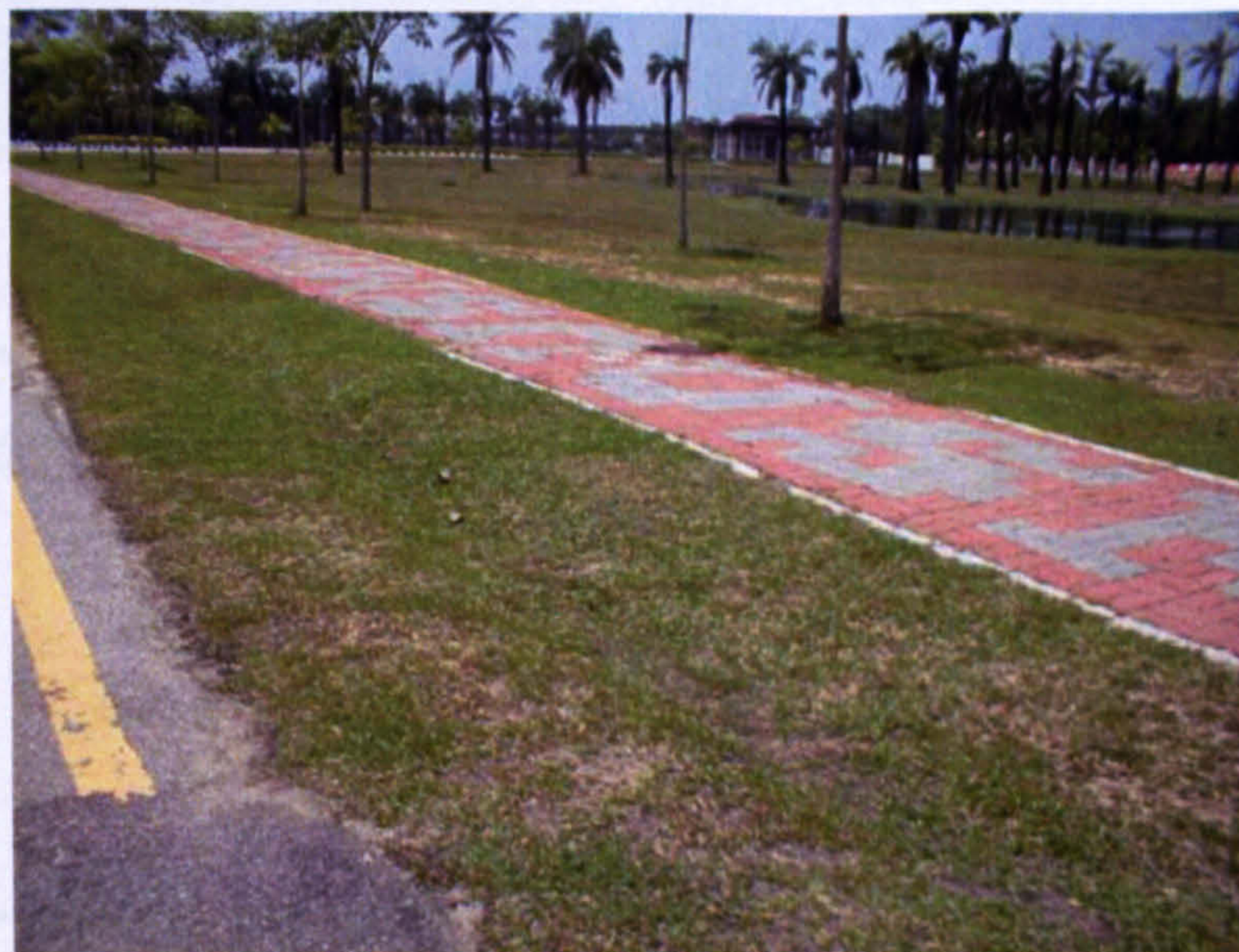
Figure 5.3.8: Ecological swale type C between the roadside and the pedestrian walkway in the USM campus
