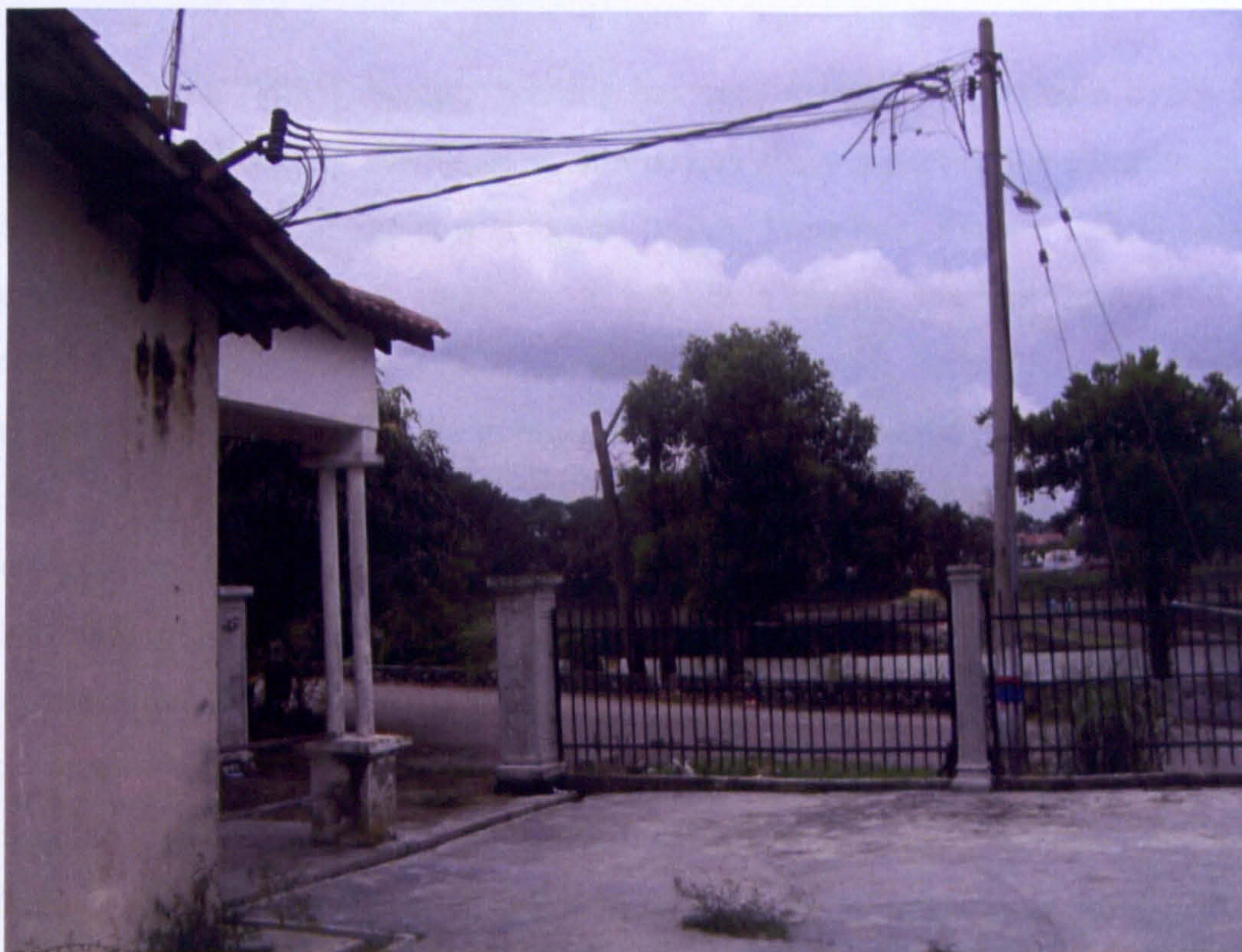
Figure 2.1.4: The whole yard area in this house unit in JB has been paved with concrete.
