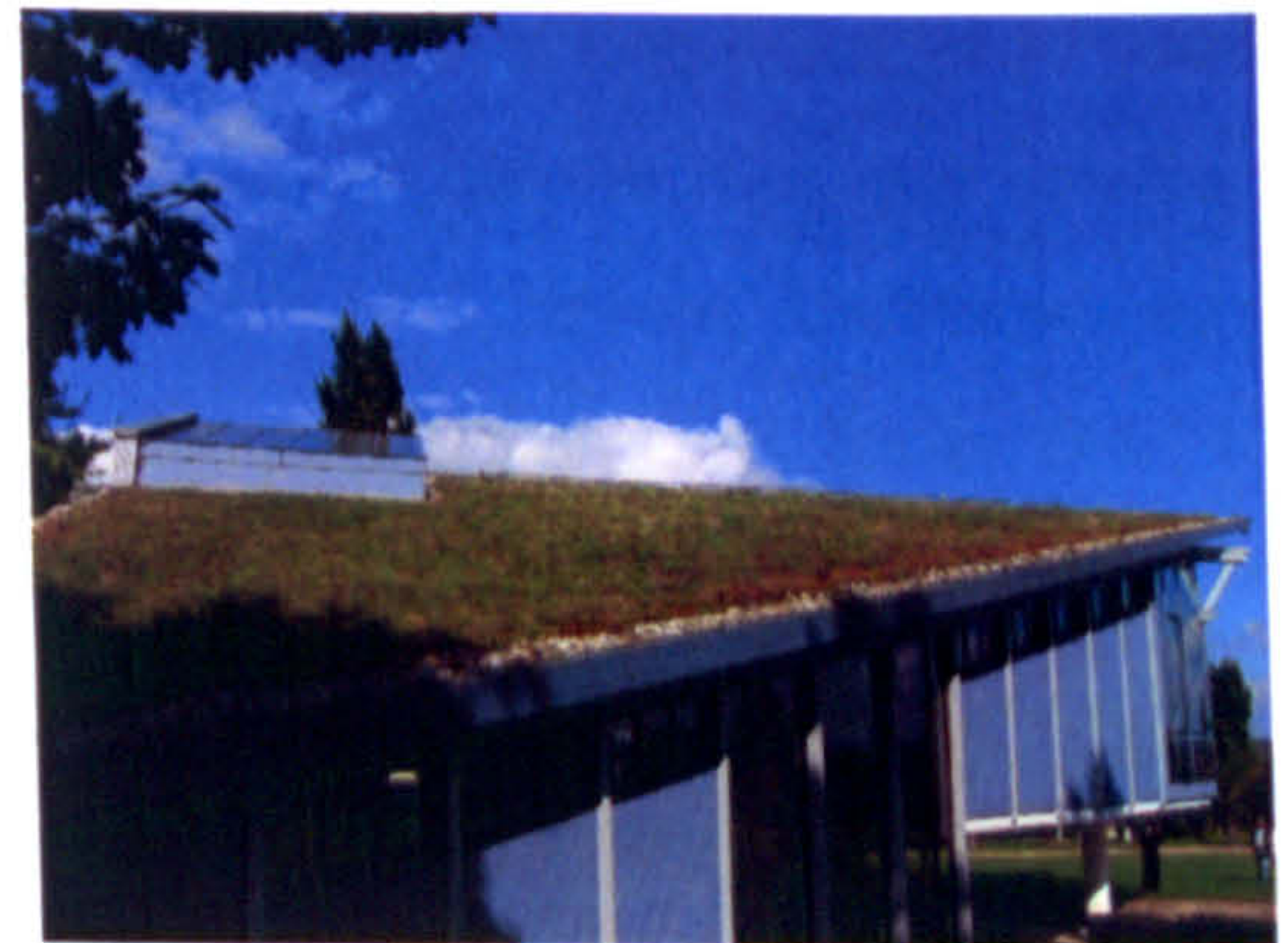
Fig.2.2 Using the gravel at the edge and corner of extensive green roofs
