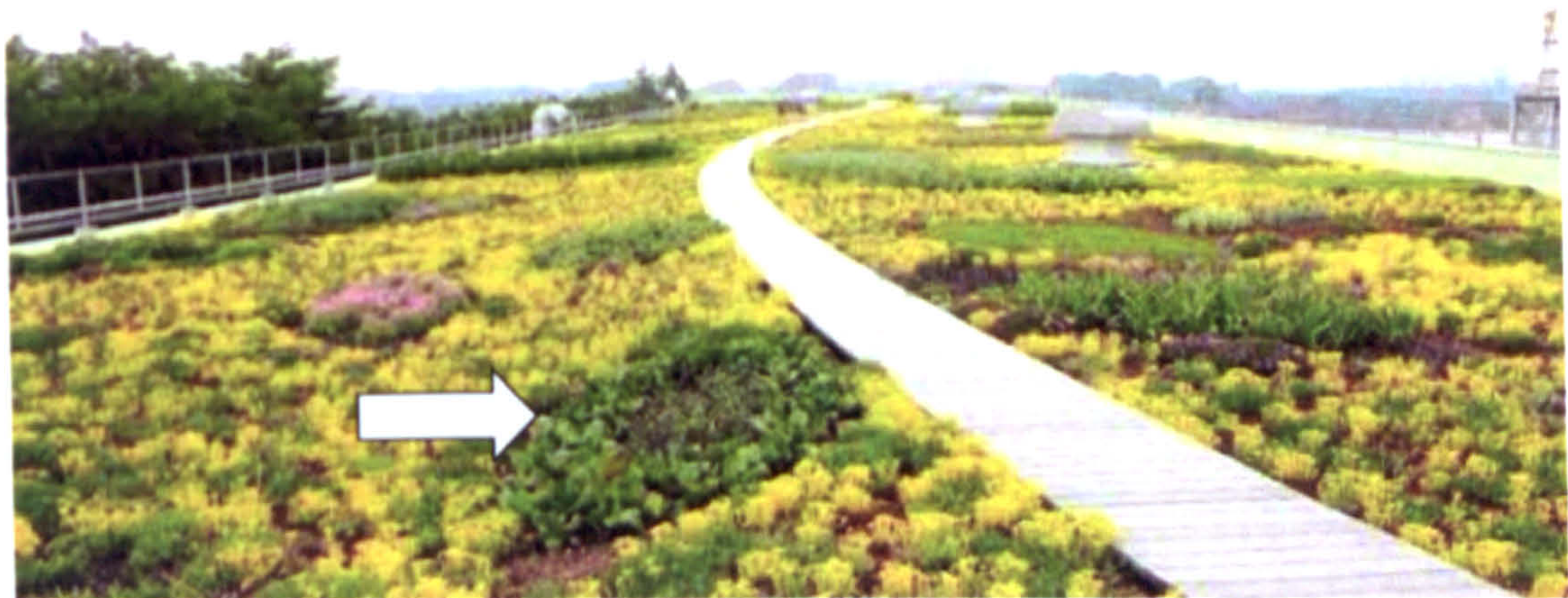
Fig.1. 49 Tajima Saitama Factory in Saitama, Japan (Source: Tajima-roofing, 2008)
