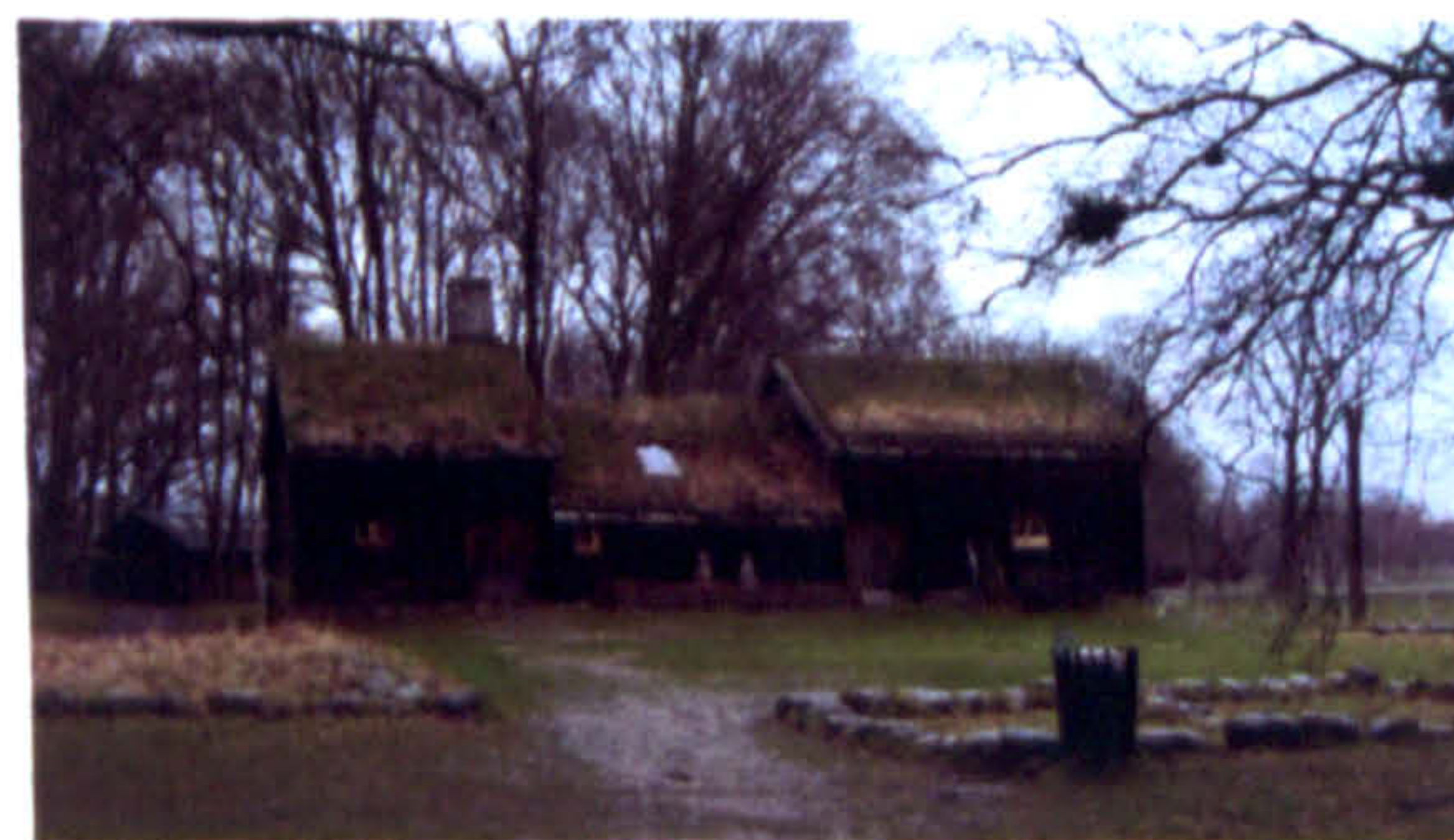
Fig.1.34 Traditional extensive green roof in Fredriksdal garden in Helsingborg, Sweden
