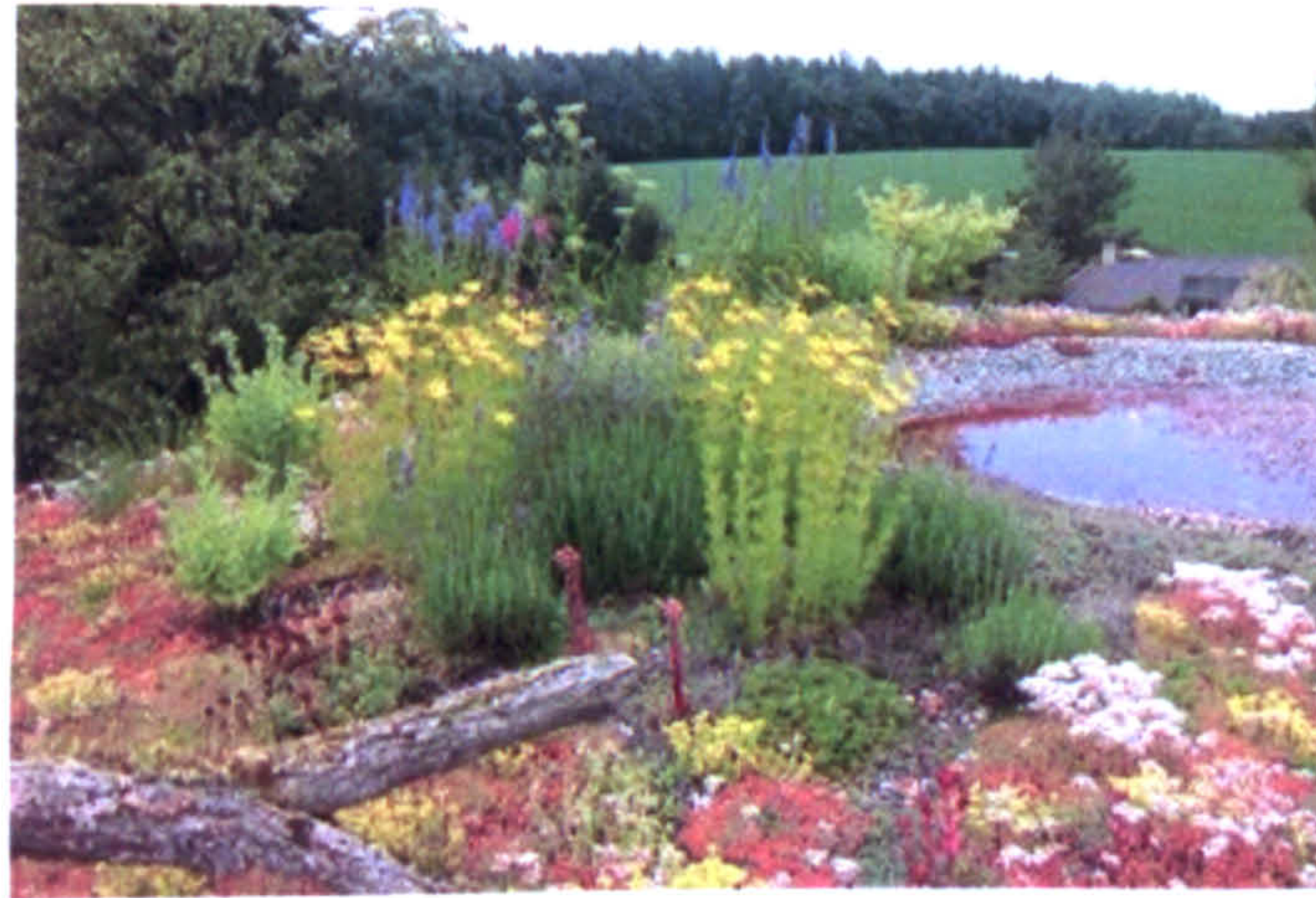
Fig.1.19 Sedum-herbaceous-grass extensive green roof (Source: Optigrün)
