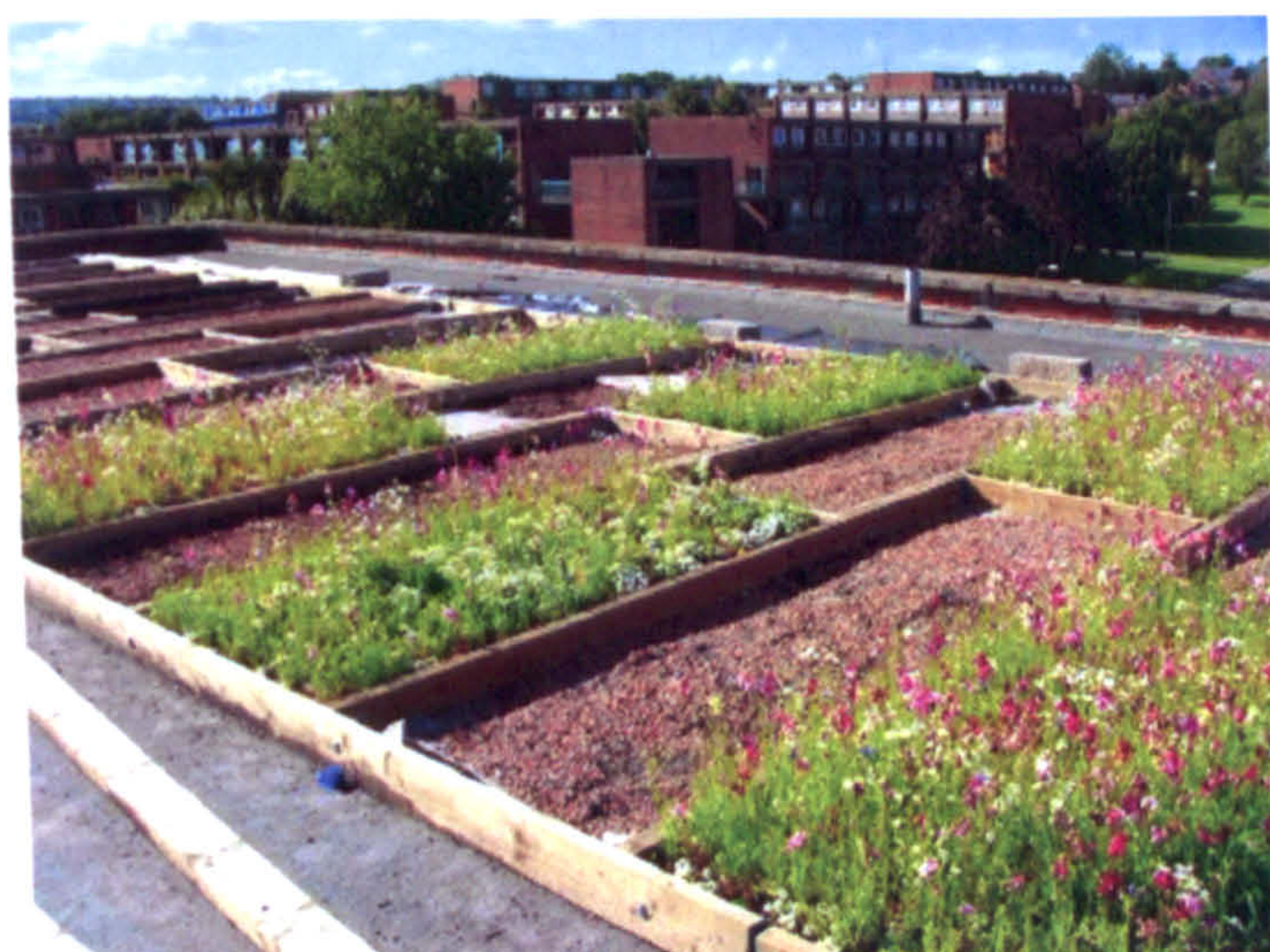
Fig.3.2.3 Overview of experimental plot on the extensive green roof
