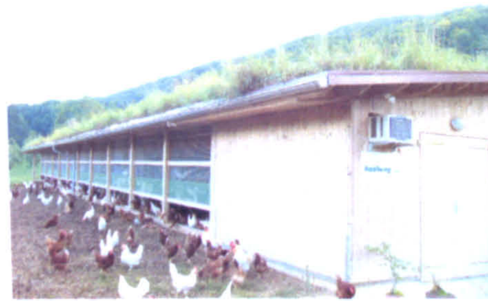
Fig. 1.12 Asphof green roof in Switzerland
