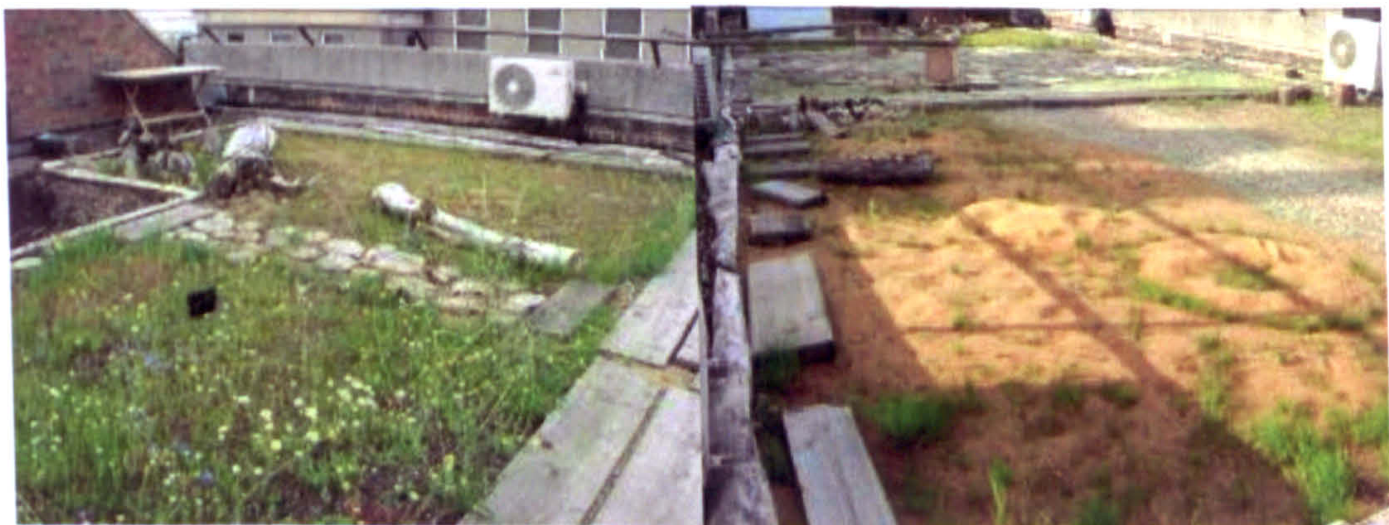
Figs. 1.29-1.30 The Office Group building in King's Cross, London
