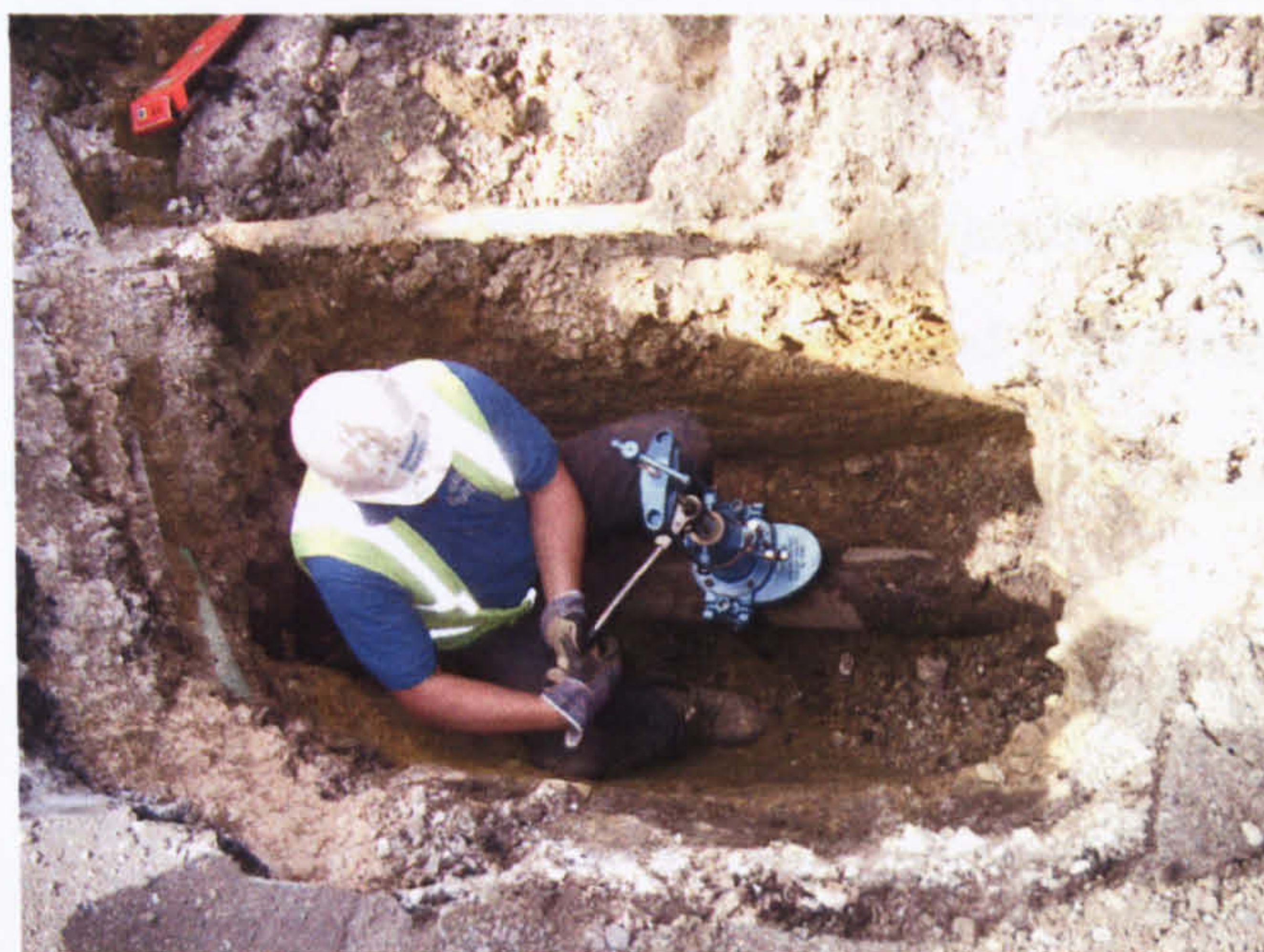
Figure 29 Installation of under pressure ferrule valve.
