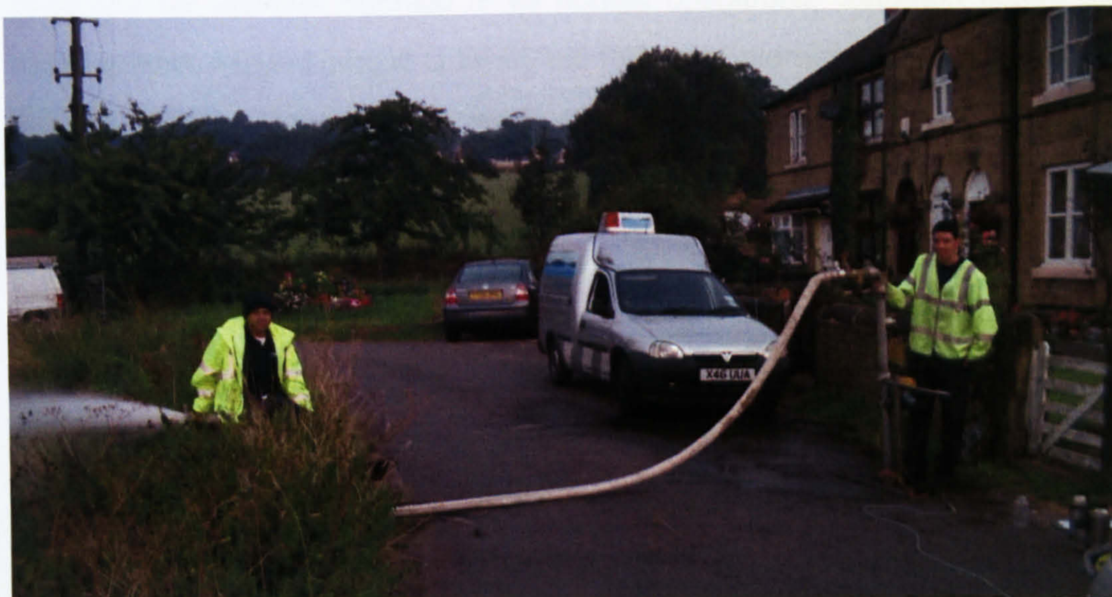
Figure 44 Use of bagging for disposal of water.
