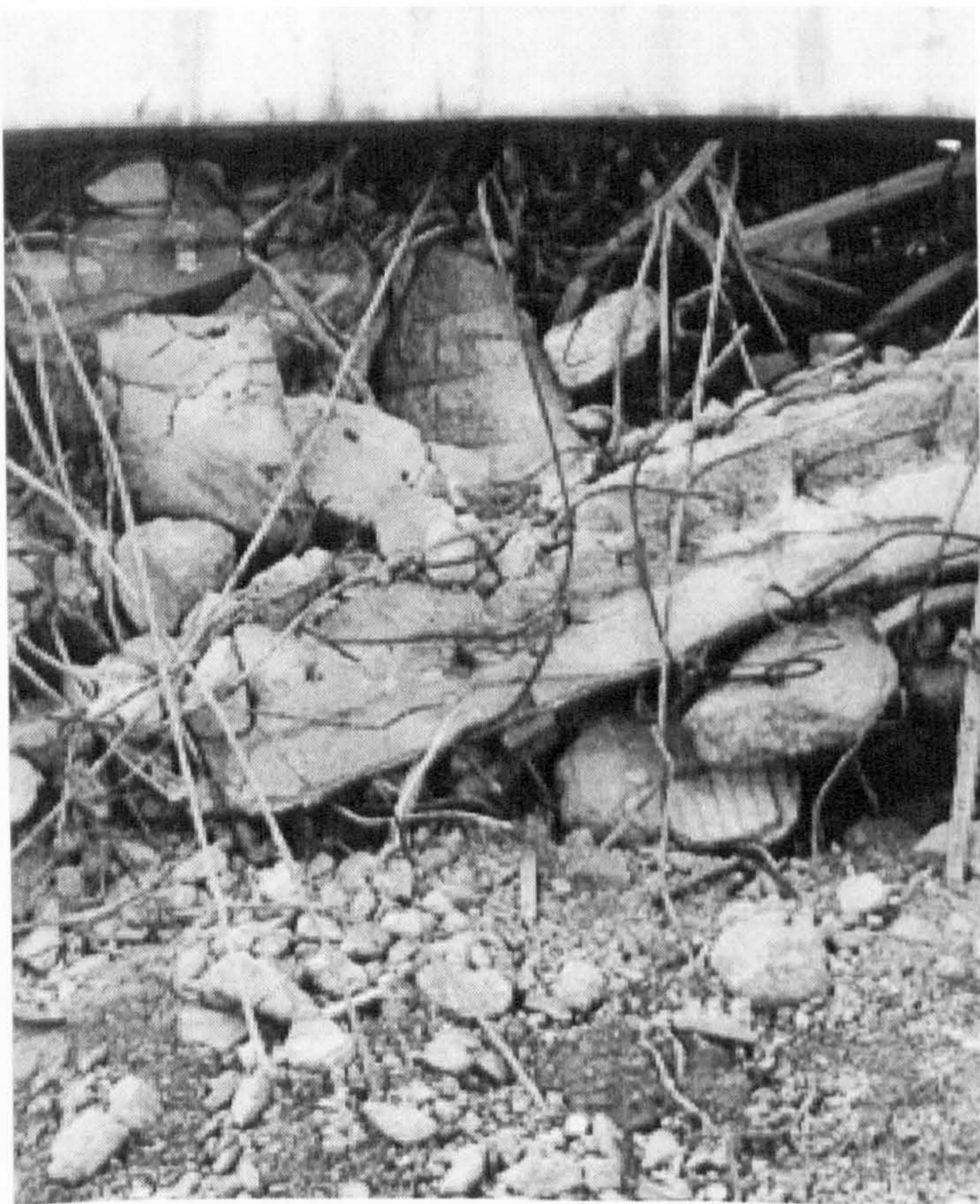
Plate 4.3 Separating Concrete and Reinforcement
