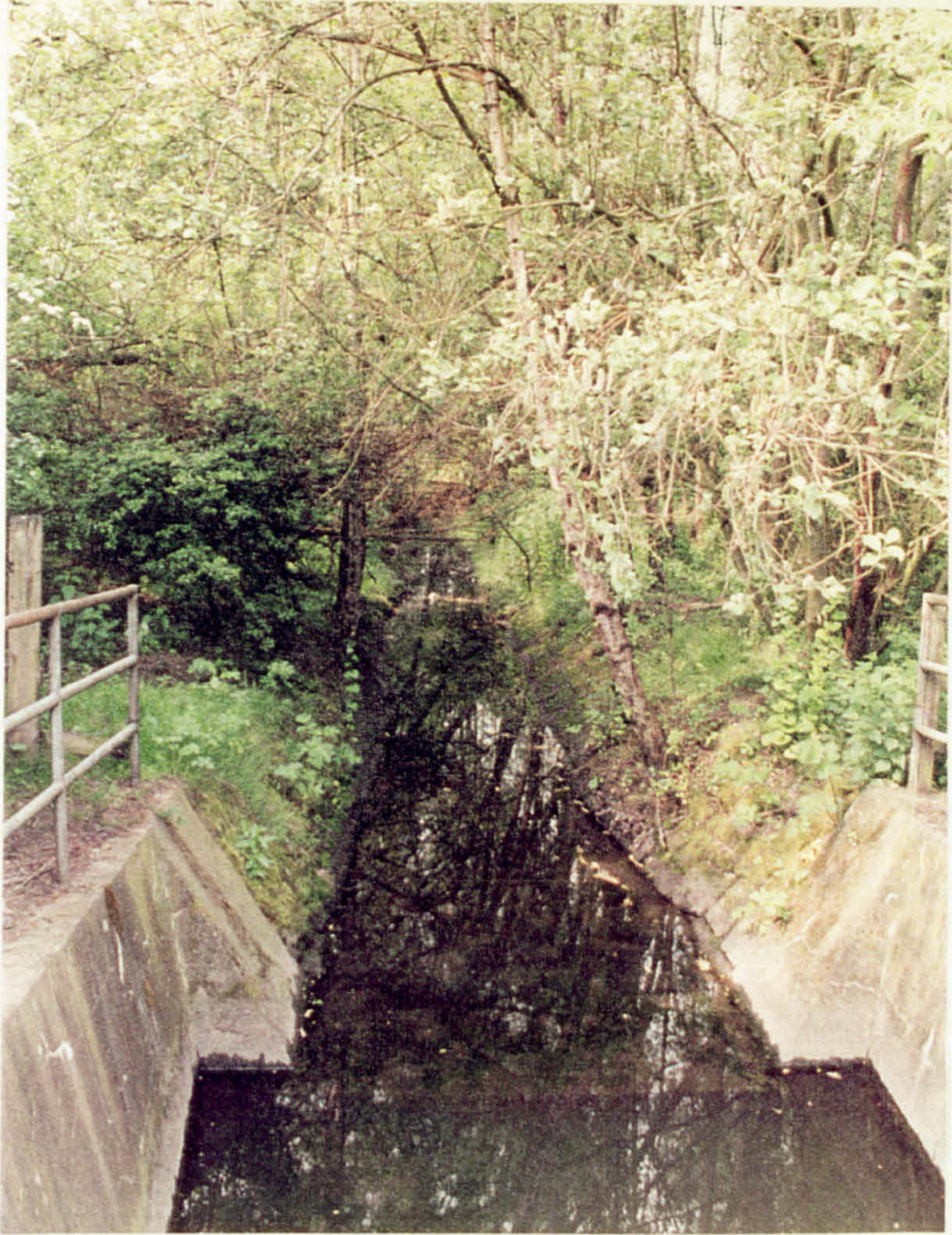
Plate 2.1.c: Pigeon Bridge Brook downstream of the motorway-discharge pipes.
