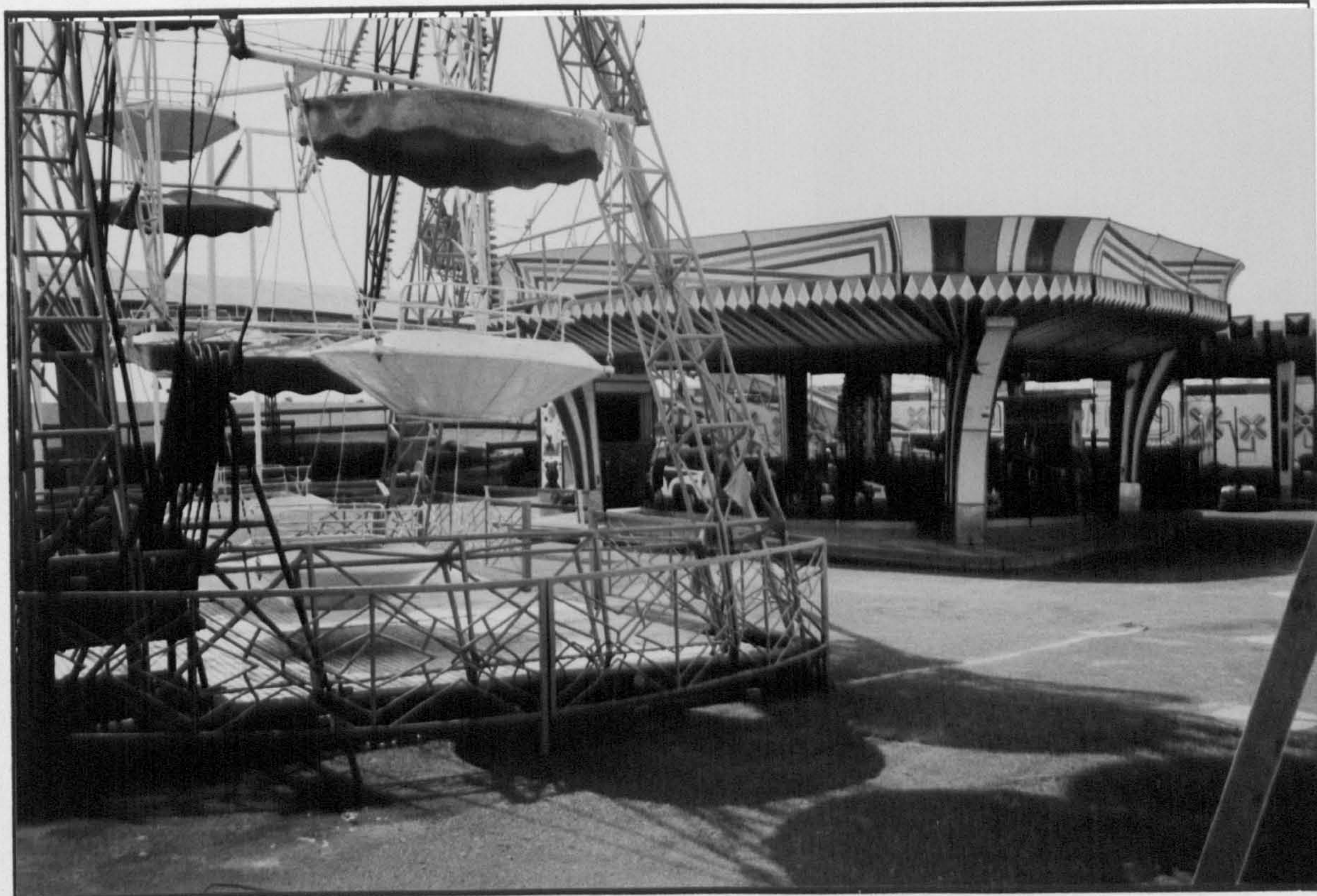
Diagram IV.D.14. Fairground Facility on The Cornice. Mechanical Equipment and Very Little Else.
