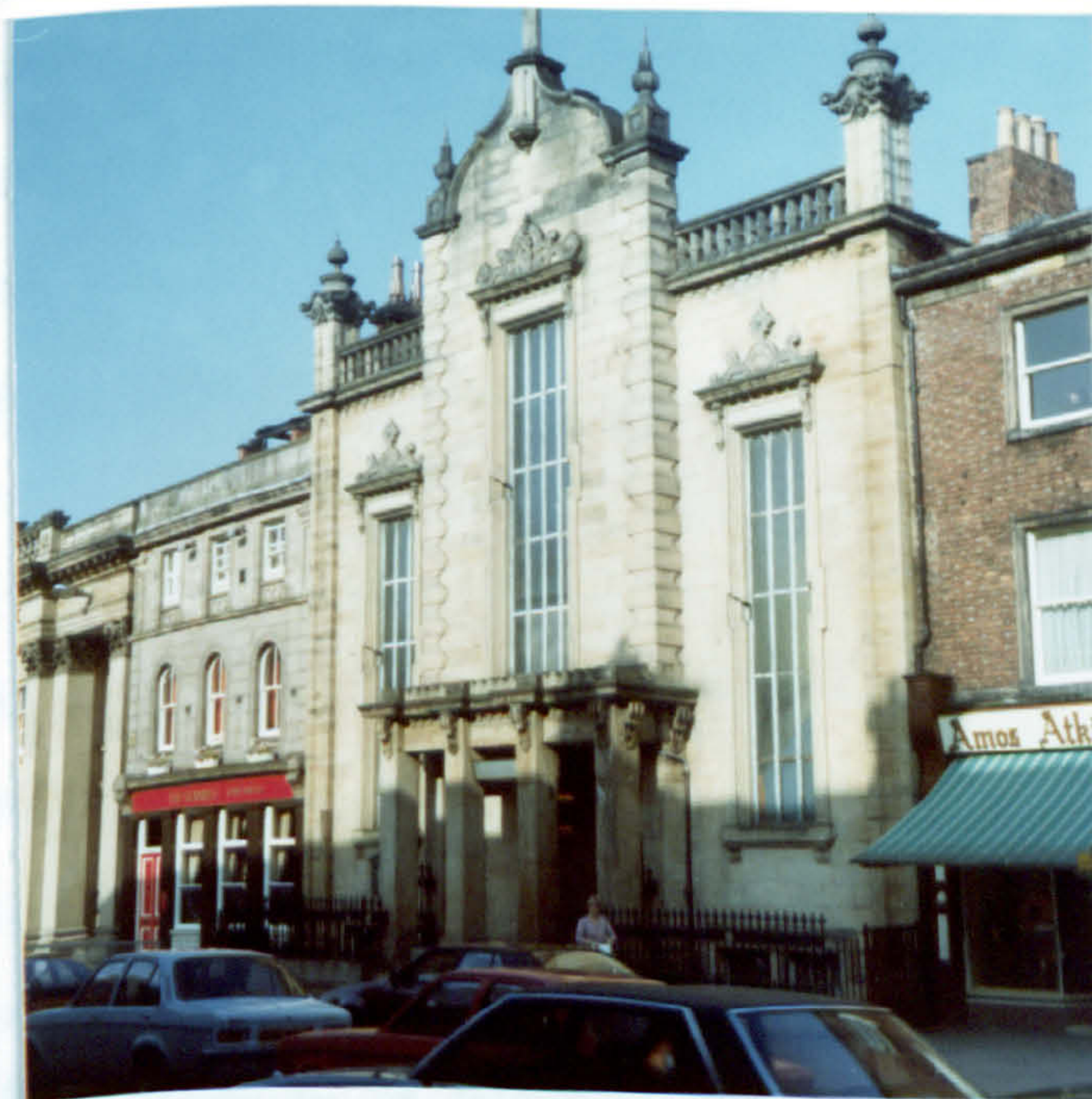
Lowther Street, Carlisle, Congregational church
