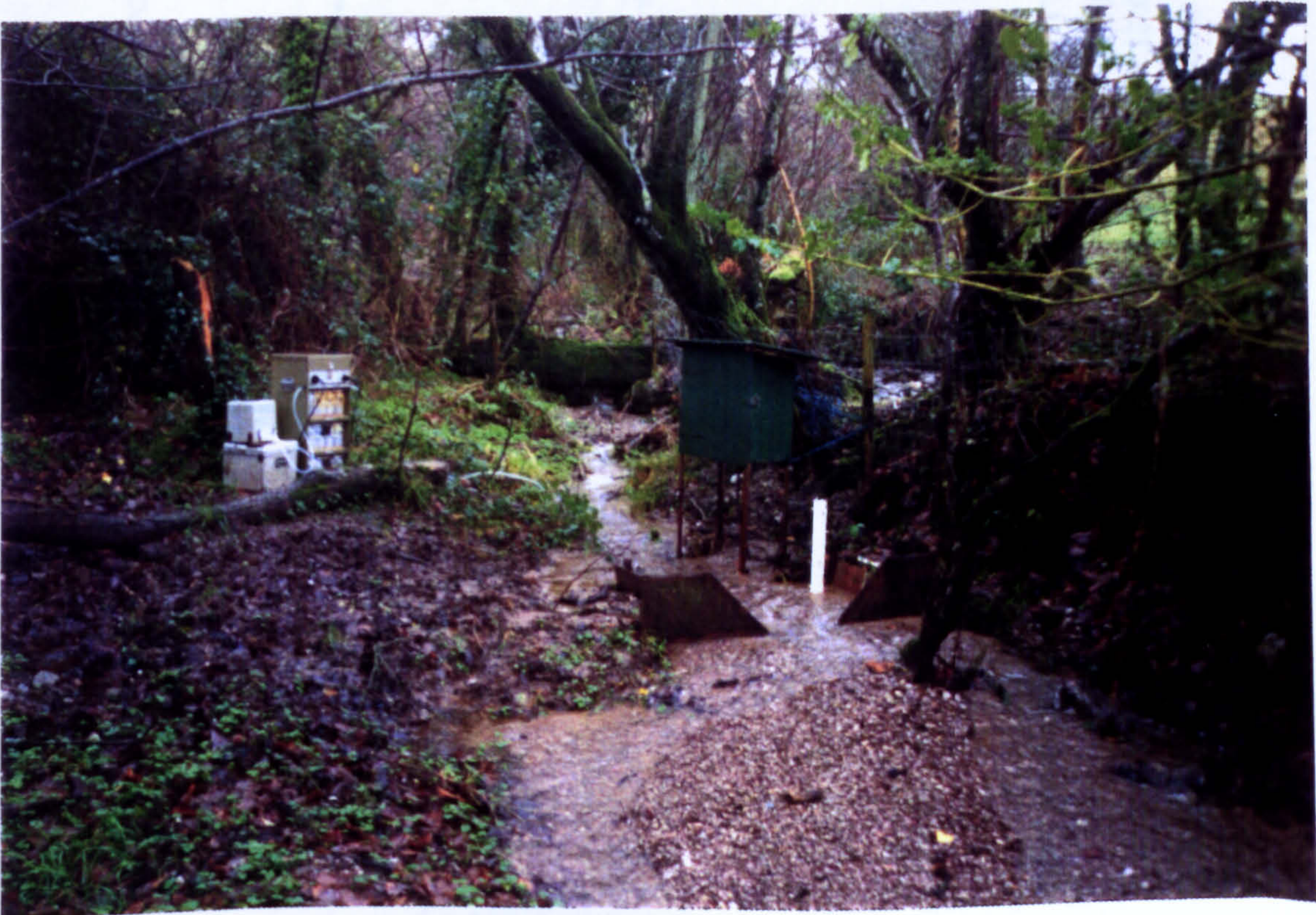
Fig.4.23. Submersion of the V-notch weir on Merrifield stream with spoil from the pond retaining bank.
