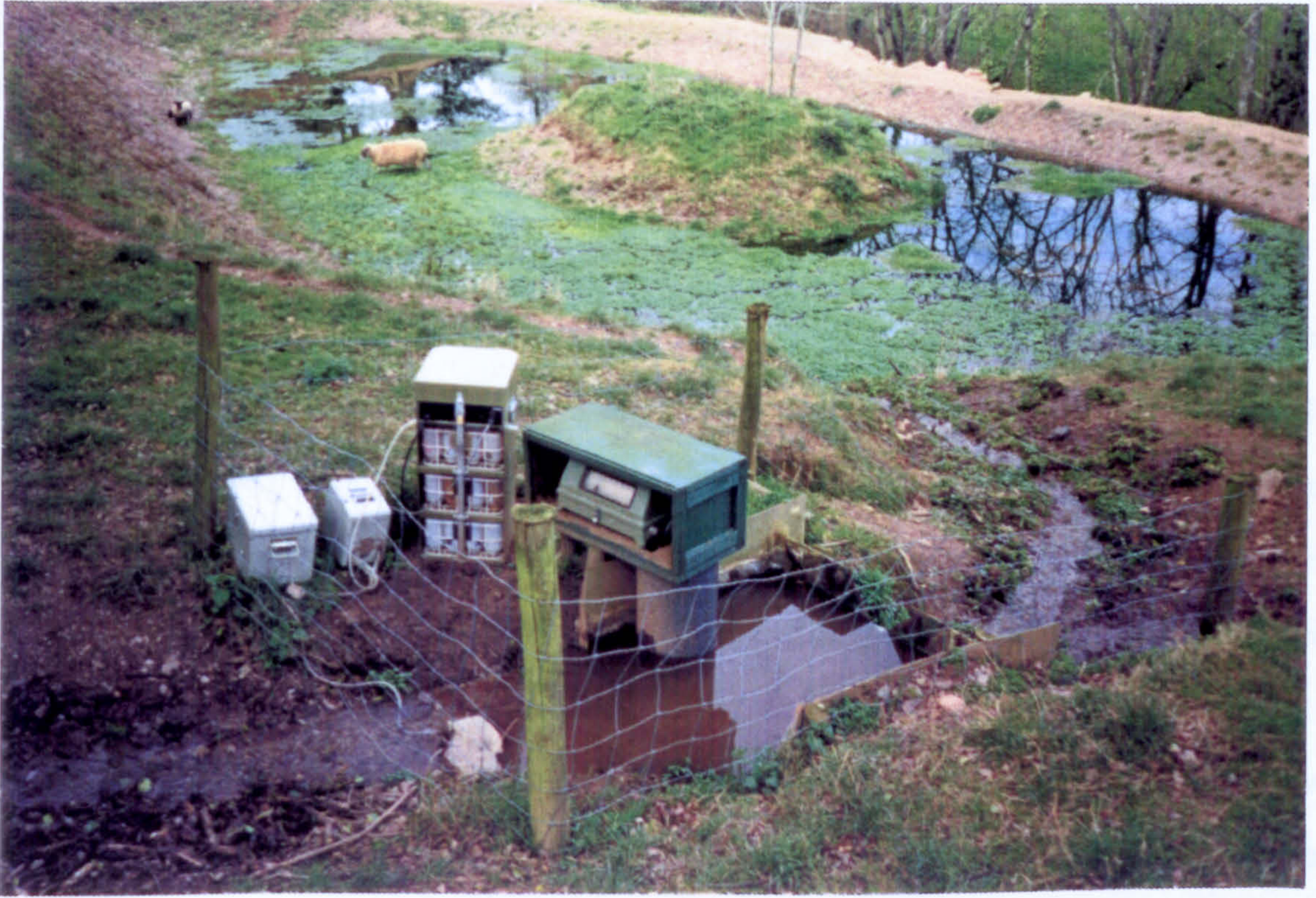
Fig.4.4. The V-notch weir on Merrifield spring, showing the stage height recorder and automatic water sampler. The pond and retaining bank is in the background.
