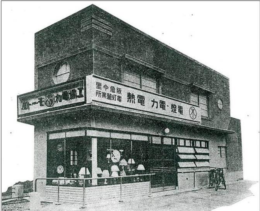
Figure 5.10 Electricity Store ( Hankyu shahō , 15 October 1935, 5) Amagasaki Municipal Archives, Amagasaki
