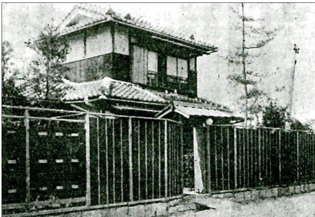
Figure 4.10 Front view of a house in Sakurai estate ( Sanyō-suitai , July 1913, 4) Ikeda Bunko Library, Ikeda
