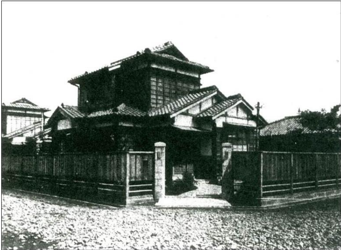
Figure 3.17 Front view of a Dōjyunkai house ( Jyūtaku , April 1931, 4) National Diet Library, Tokyo
