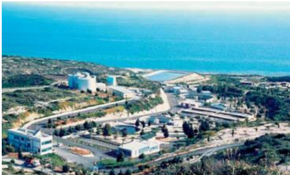
Plate 2.2 Wastewater treatment plant of Limassol, Cyprus
