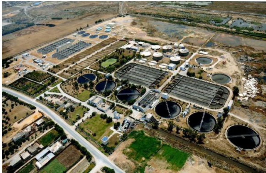
Plate 2.4 Wastewater treatment plant of Chotrana in Tunisia
