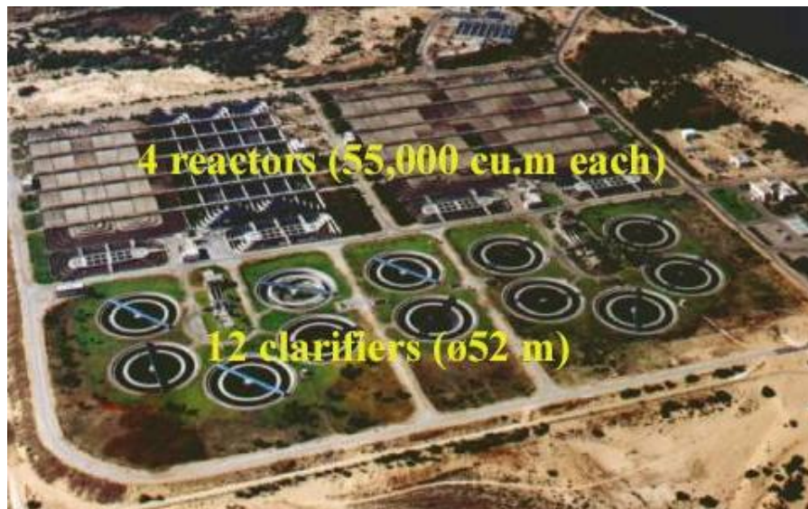
Plate 2.3 Wastewater treatment plant of Tel-Aviv in Israel
