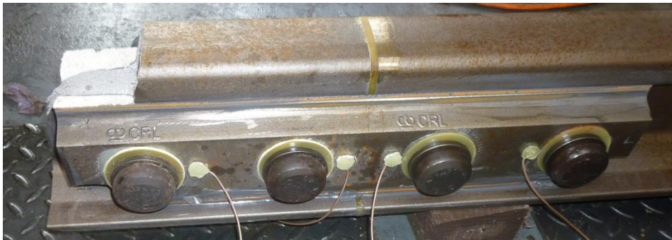
Figure 80: Failure of the full fit IBJ due to a failure of the rail
