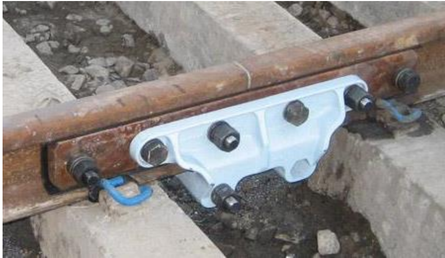
Figure 13: 'Hercules' insulated rail joint support plates (17)
