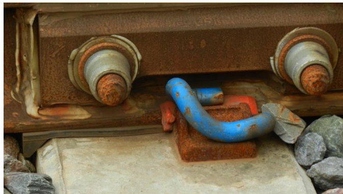
Figure 9: A six hole fishplate with material removed to allow fitment of the fastening system, in this case a Pandrol 'e-clip'
