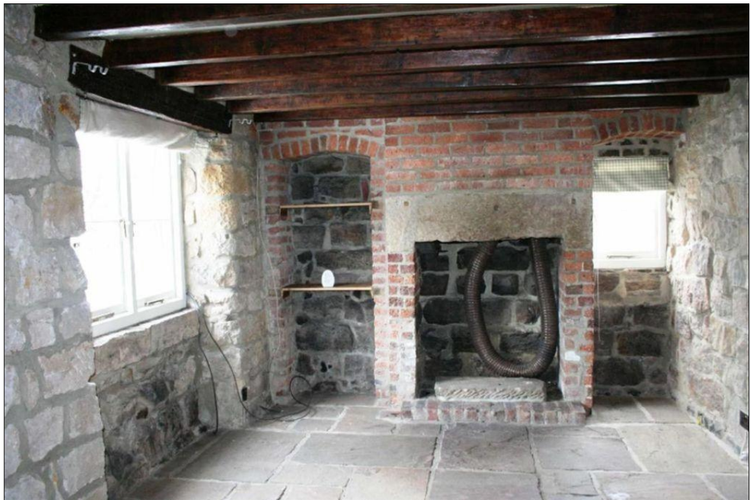
Figure 5.53: Ground floor fireplace at No. 23 East Terrace (source: Crown Copyright, Rightmove)
