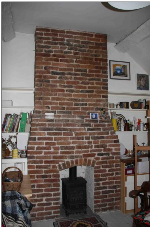
Figure 3.57: Second floor chimney breast arrangement at No.25 North Street (source: author's own photo)
