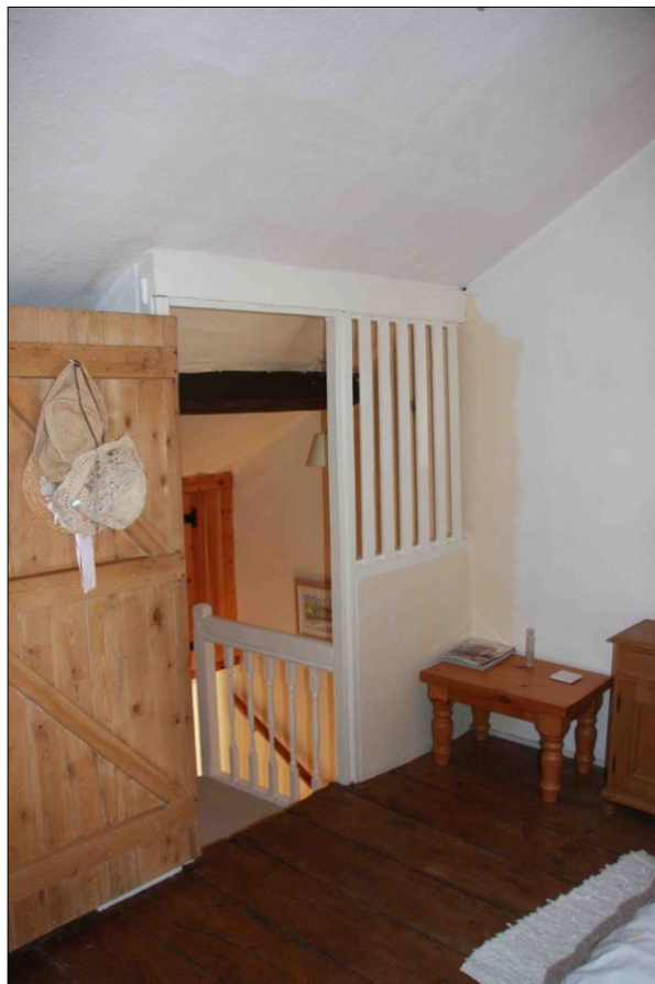
Figure 5.61: Floor boards at No. 9 Hopping Hill (source: author's own photo)
