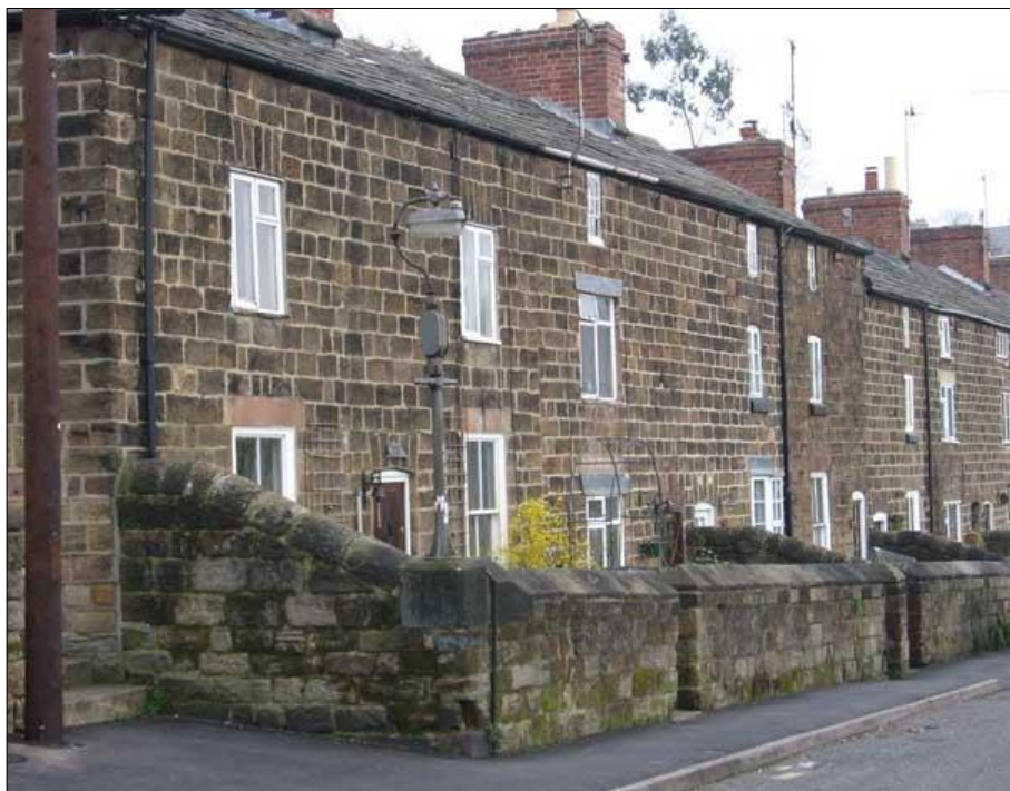
Figure 5.9: Abutment of roof-lines between Nos.8-16 and Nos.17-24 Hopping Hill (source: author's own photo)
