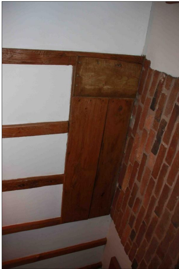
Figure 3.63: additional timber joists in the ground floor ceiling to support the first floor hearth (source: author's own photo)
