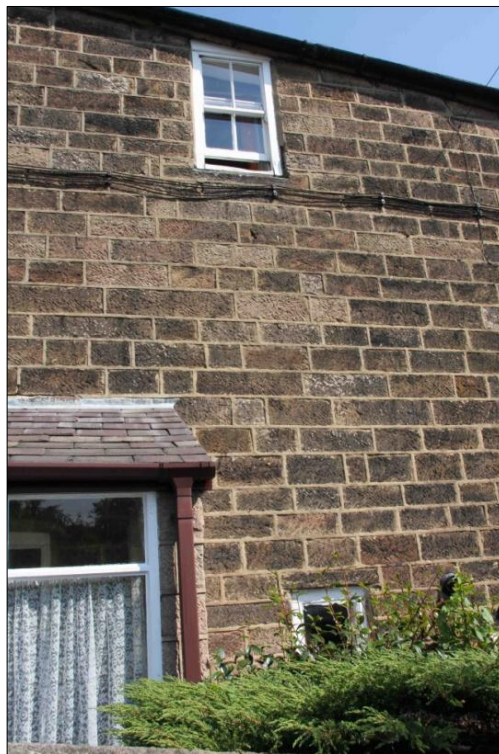
Figure 5.26: Additional windows in No. 2 (right window) and 3 (left window) Chevin Alley (source: author's own photo)
