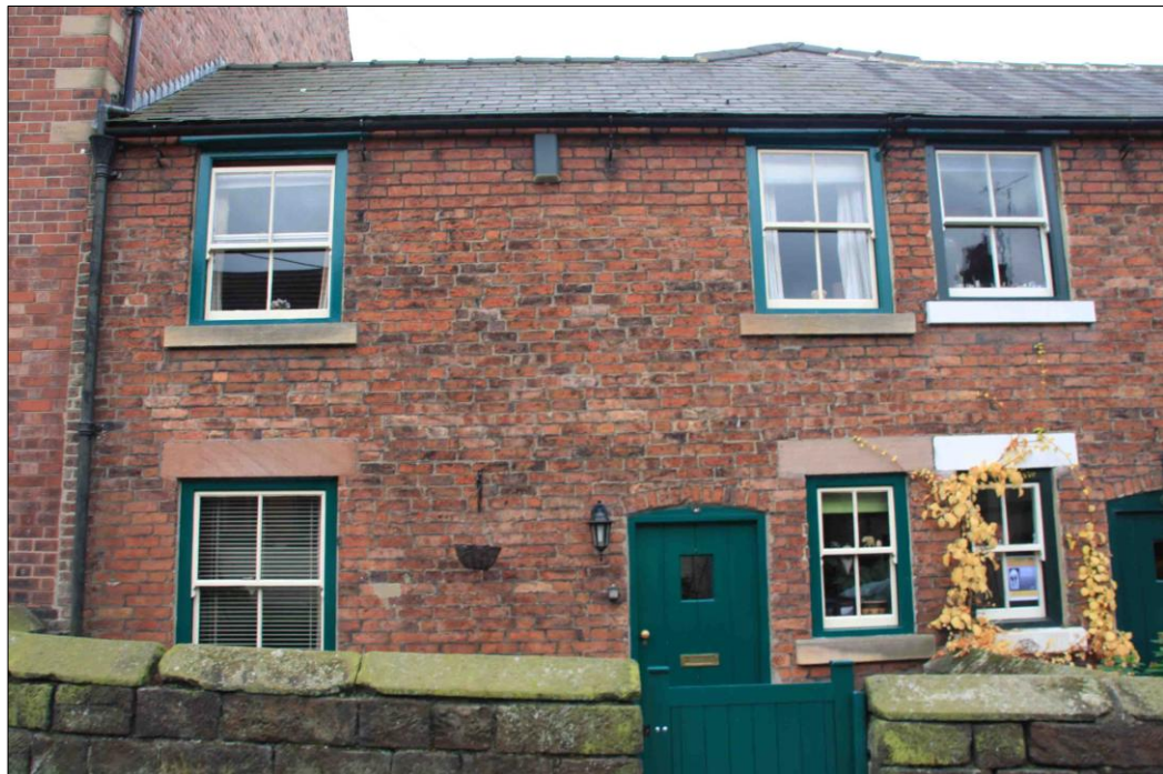
Figure 4.16: Group J property, note the arrangement of the windows and style of the forecourt area (source: author's own photo)
