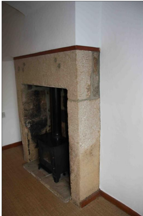
Figure 5.50: Ground floor fireplace, style used in Plans 10 and 13 properties (source: author's own photo)
