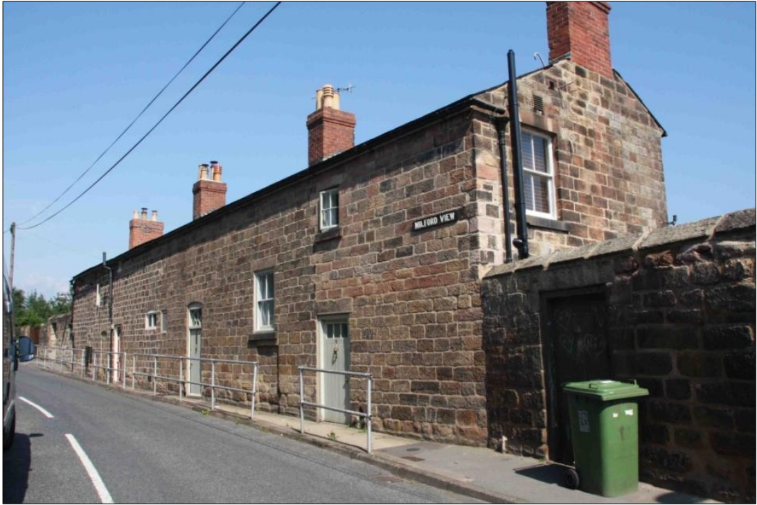
Figure 5.12: The Bleach Houses, Chevin Road (source: author's own photo)
