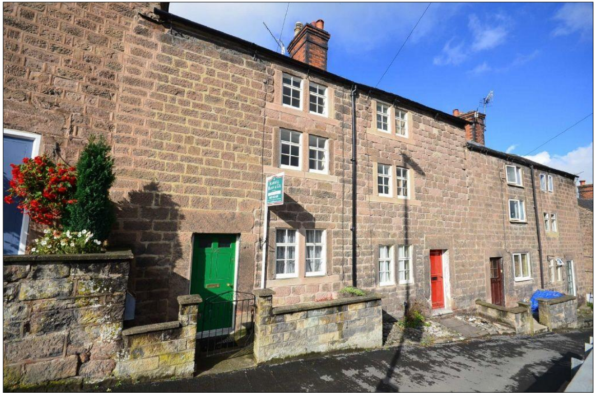
Figure 3.22: Group C properties, Cromford. Note the forecourt arrangement (source: DCC)
