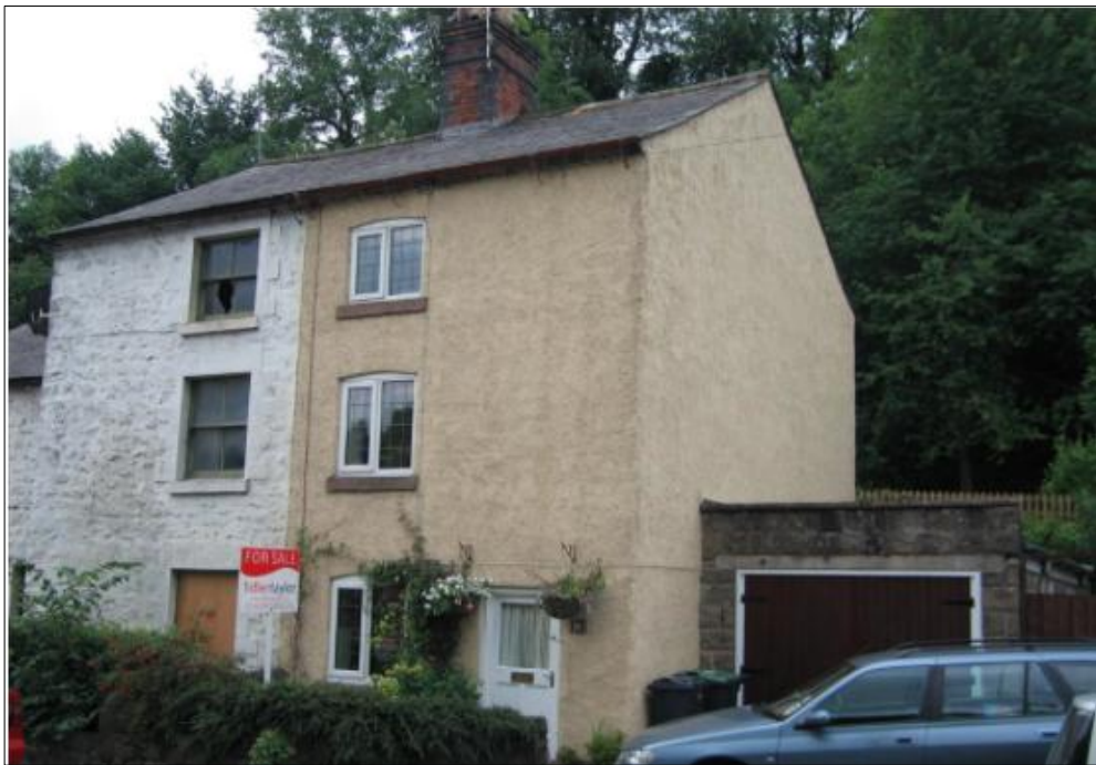
Figure 3.9: Water Lane, Cromford. Built in the 1820s ( Group F ) (source: DCC)
