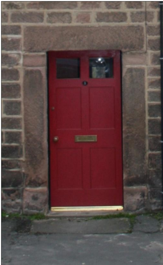
Figure 3.14: Detail of elaborate door surround of Group A properties (source: author's own photo)
