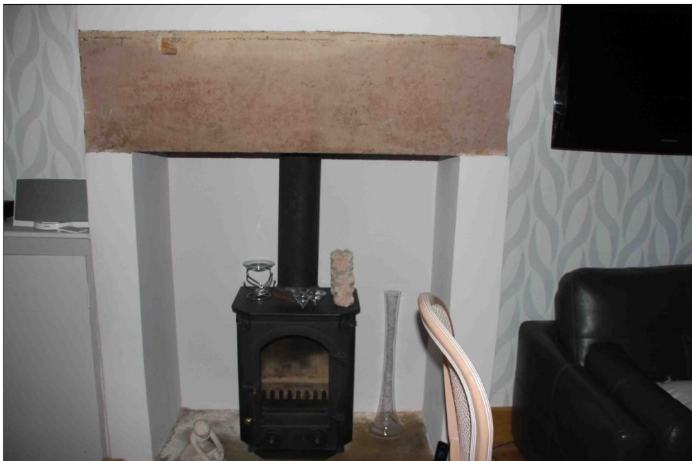
Figure 6.32: Ground floor fireplace at No. 15 Brick Row (source: author's own photo)
