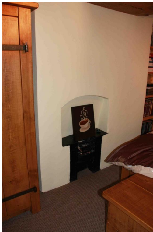
Figure 3.54: First floor chimney breast and fireplace in No.1 North Street (source: author's own photo)
