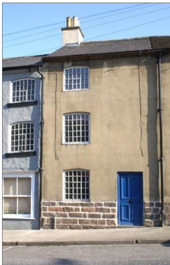
Figure 3.30: Mid-nineteenth century housing, The Hill Cromford (source: DCC)
