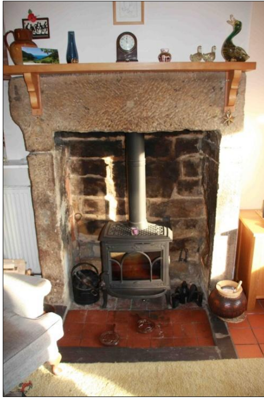
Figure 5.54: Fireplace at No. 23 Hopping Hill, note the soot pattern on the fireback (source: author's own photo)
