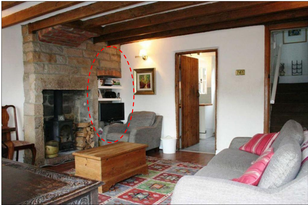
Figure 5.64: Ground floor of No. 15 Hopping Hill, note the segmental arched recess (outlined) (source: DCC)
