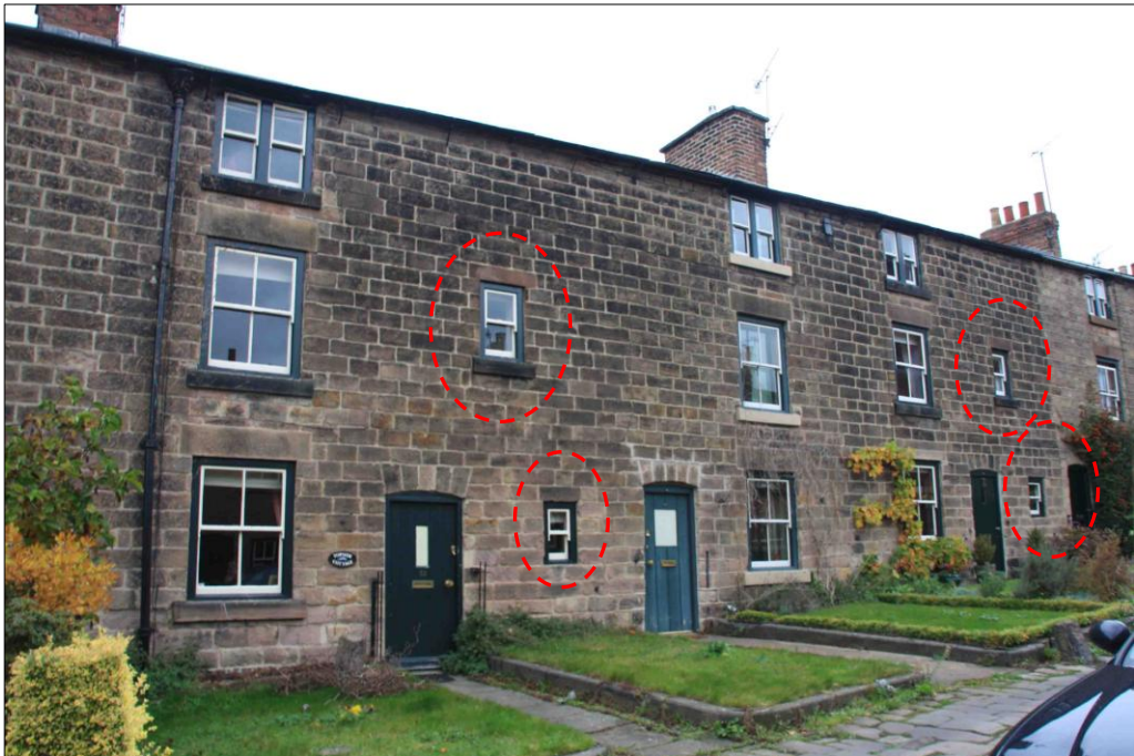
Figure 4.14: Detail of Group I properties, note the additional staircase and cellar windows (circled) (source: author's own photo)
