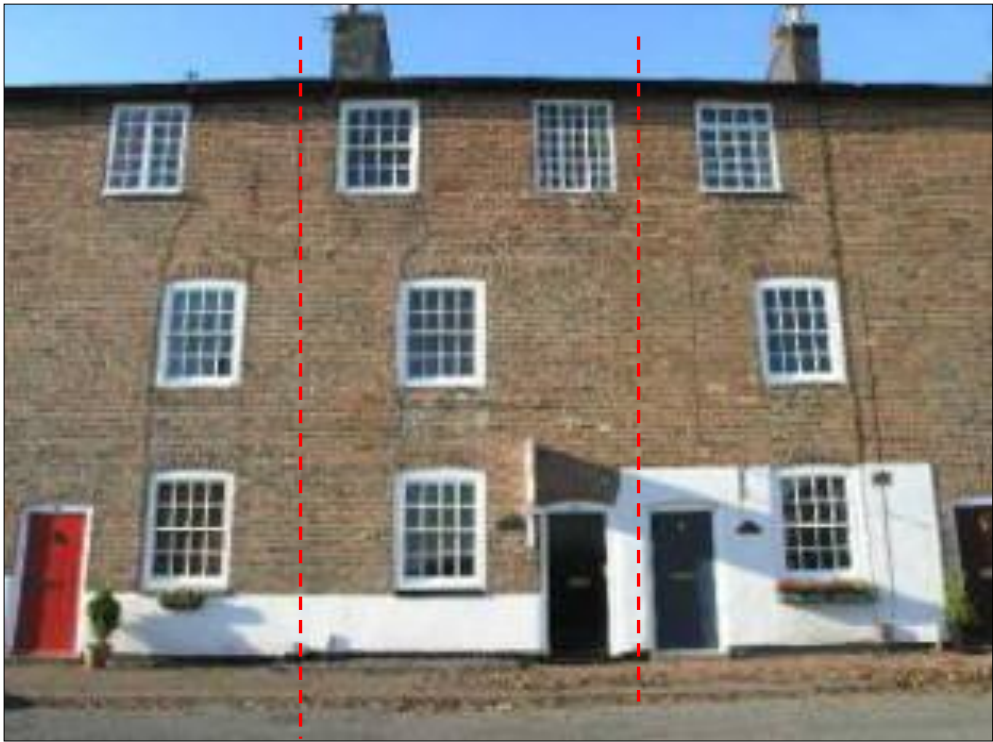
Figure 6.17: No. 11 Brick Row (source: DCC)
