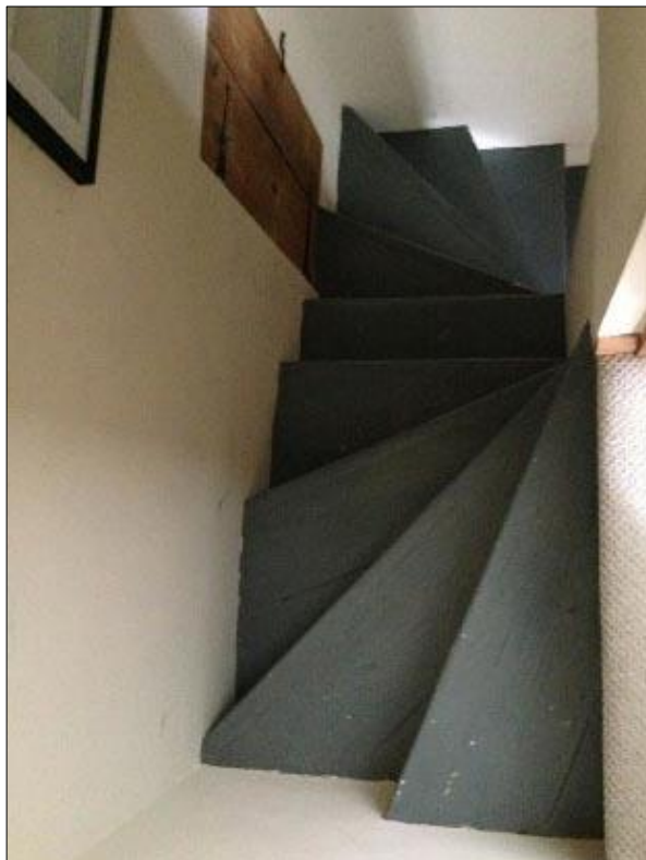
Figure 5.41: Winder staircase at No.2 Dukes Building (source: DCC)
