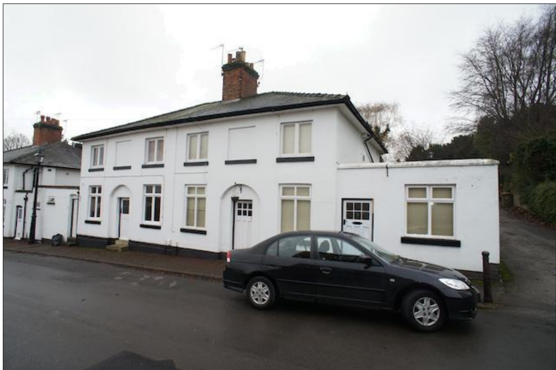
Figure 6.13: Upper New Road (source: DCC)
