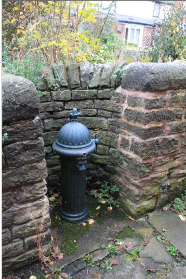
Figure 4.57: Detail of water pump at Short Row (source: author's own photo)
