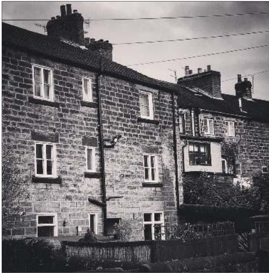
Figure 5.29: No. 2 Dukes Buildings (source: DRO)
