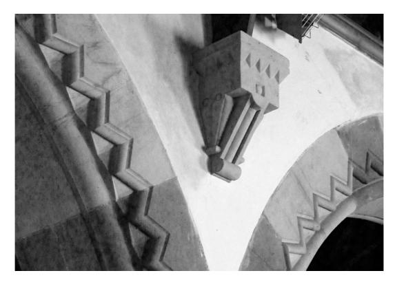
Figure 8.20 Neo-Romanesque corbel supporting the wall plate of a principal rafter
