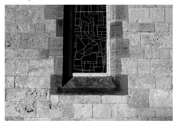
Figure 8.9 Detail of the disturbed stonework surrounding the nave windows – note that the window quoins do not course within the masonry and some stones have been cut to fit the quoins
