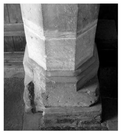
Figure 7.8 Detail of a parclose screen scar in the south-eastern face of the south aisle pier base
