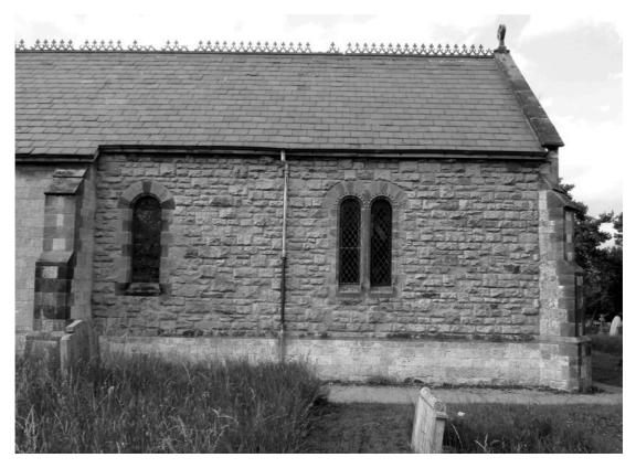
Figure 8.28 South elevation of the chancel (exterior) - note the limestone ashlar of the nave and chancel plinth versus the rock-faced sandstone masonry of the chancel wall
