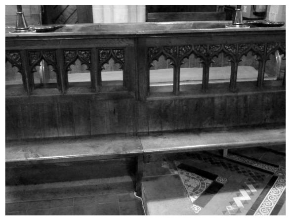
Figure 5.42 Detail of the choir stalls (north side), showing a straight join level with the step, and the quarry tiles marking the possible location of the stored choir desks
