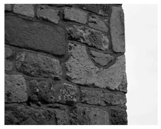
Figure 4.32 Detail of a window head (inverted) reused as a quoin in the tower
