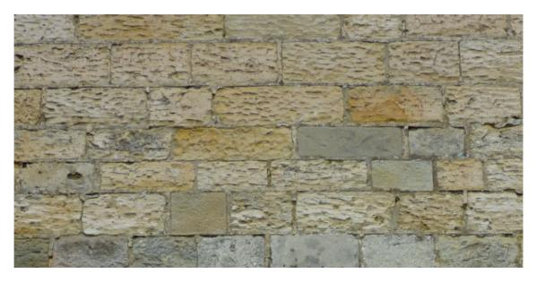
Figure 4.37 Detail of exterior wall showing the 19th-century tooling and masonry
