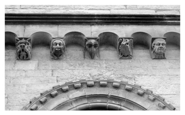
Figure 6.7 Detail of the Victorian exterior corbel table
