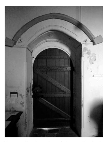
Figure 8.14 Interior of the south doorway, showing the moulded arch and blank label-stops
