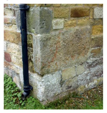
Figure 4.18 Detail of large quoins employed at the north-west angle of the north aisle
