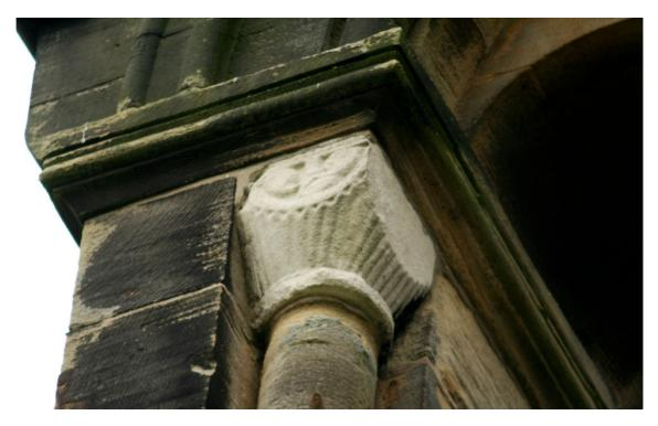
Figure 6.11 Detail of one of a limestone bellcote capital
