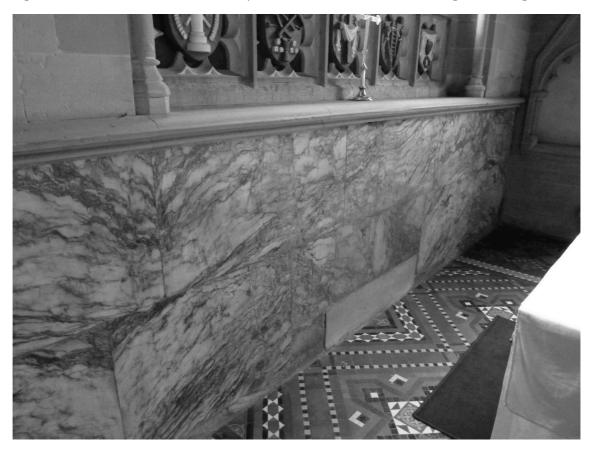
Figure 5.26 Detail of the interior east wall of the chancel, showing the plain foundation stone within the Alabaster reredos
