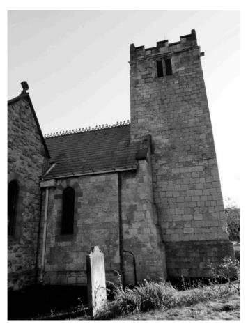
Figure 8.39 The nave west wall & its shallow buttress project across the north face of the tower
