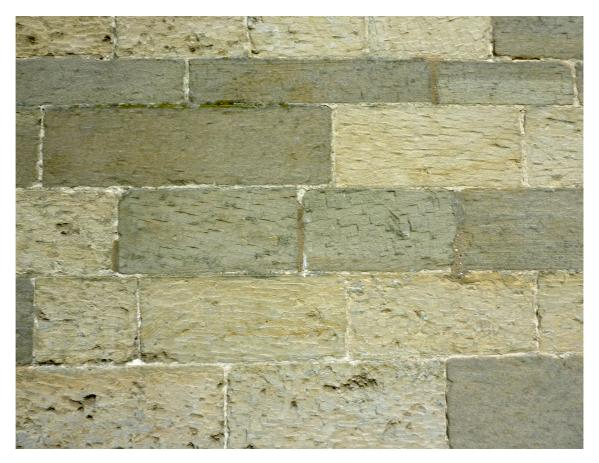
Figure 5.59 Detail of the exterior masonry, showing the variation in geology but consistent tooling
