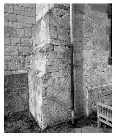
Figure 8.11 Detail of the shallow buttress at the south-west corner of the nave, showing the interrupted plinth and disturbed stonework coursing
