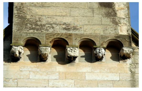
Figure 6.10 Bellcote corbels on the western elevation – note the pale limestone
