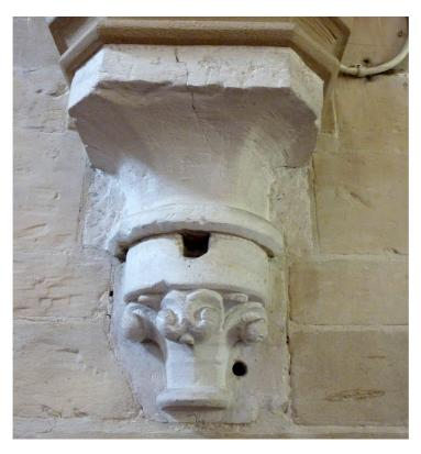
Figure 5.47 Detail of the western respond of the north aisle arcade, showing wear and alteration
