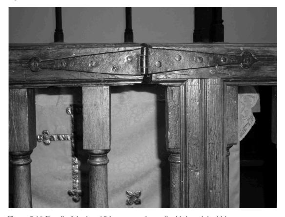
Figure 7.10 Detail of the late 17th-century altar rail with its original hinges
