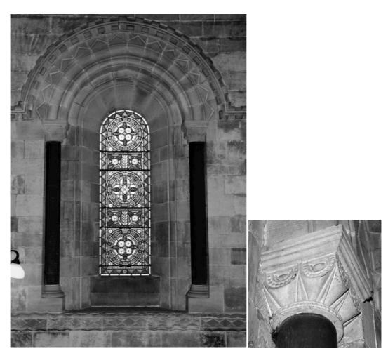
Figure 6.31 Chancel window (interior) showing the increased level of decoration, including the treatment of the nook shaft capitals (inset)
