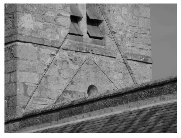
Figure 7.6 Earlier roof lines (highlighted) visible on the east elevation of the tower
