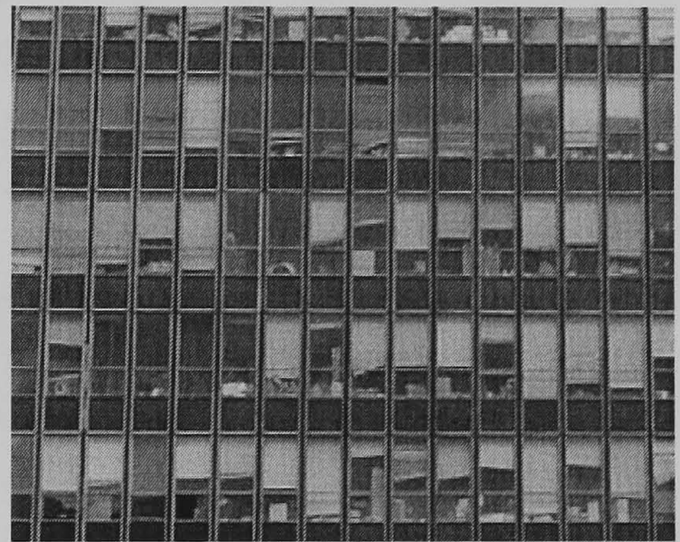
Figure 4.8 Window and blind in the Arts Tower
