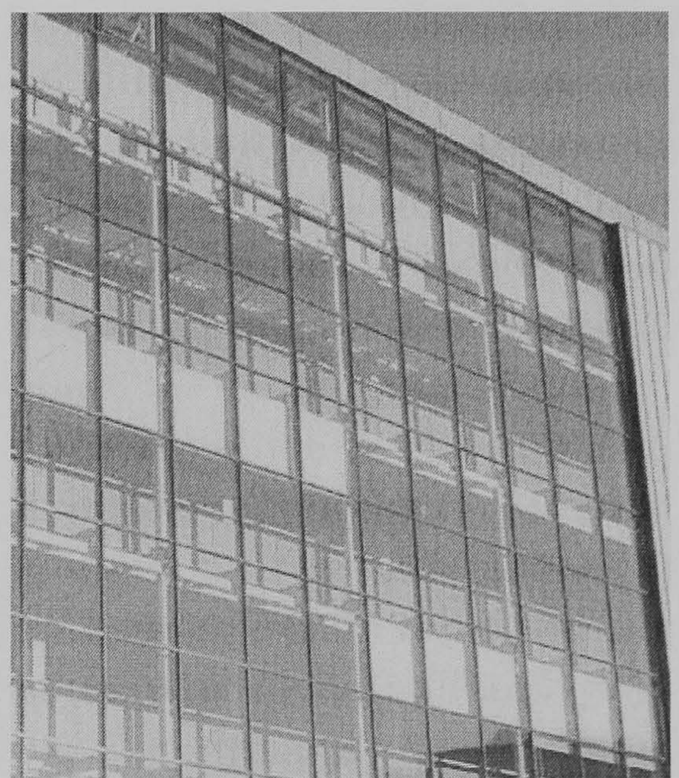
Figure 4.9 Window and shading roll in the ICOSS Building
