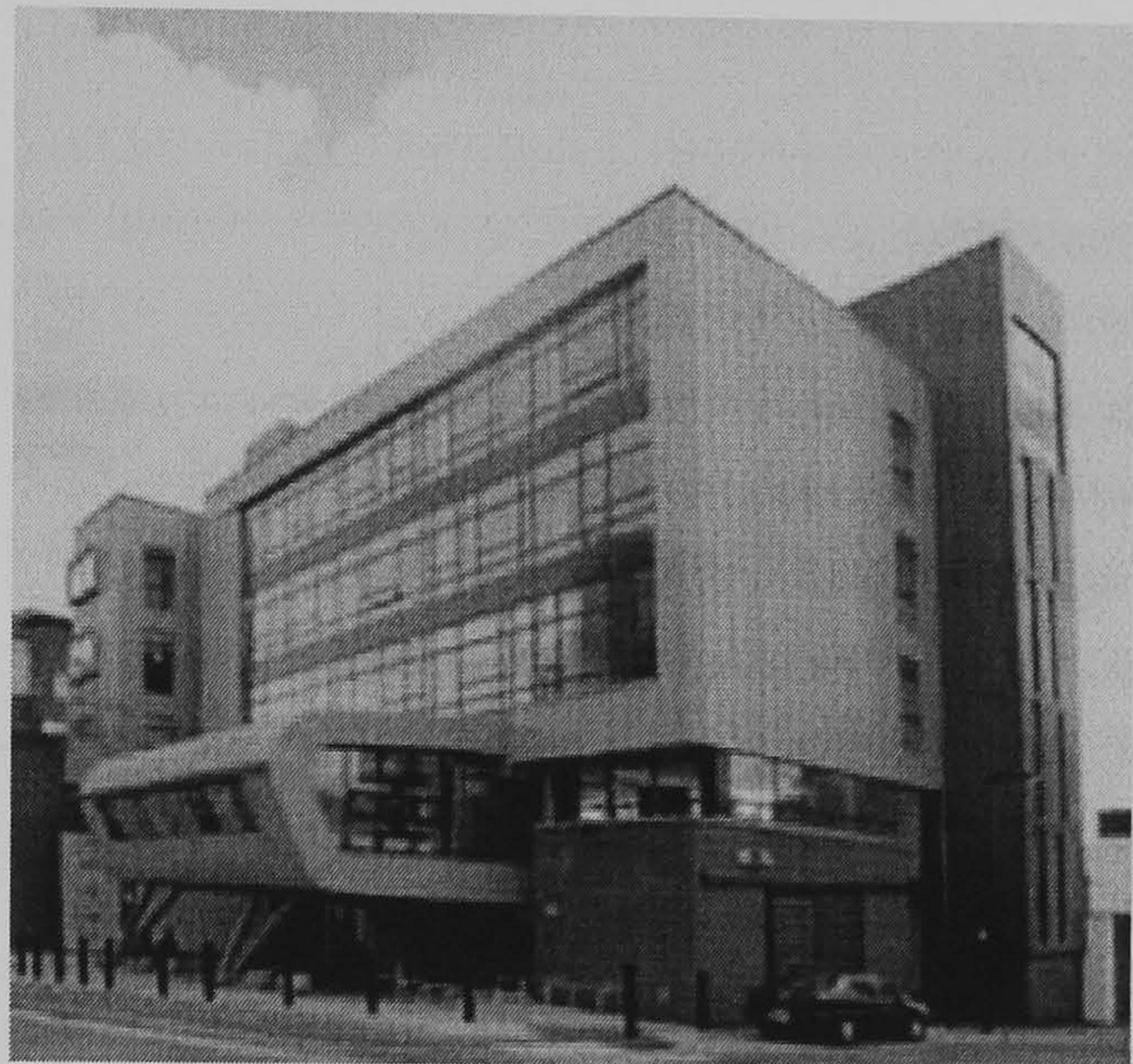
Figure 5.24 Northwest view of the ICOSS Building
