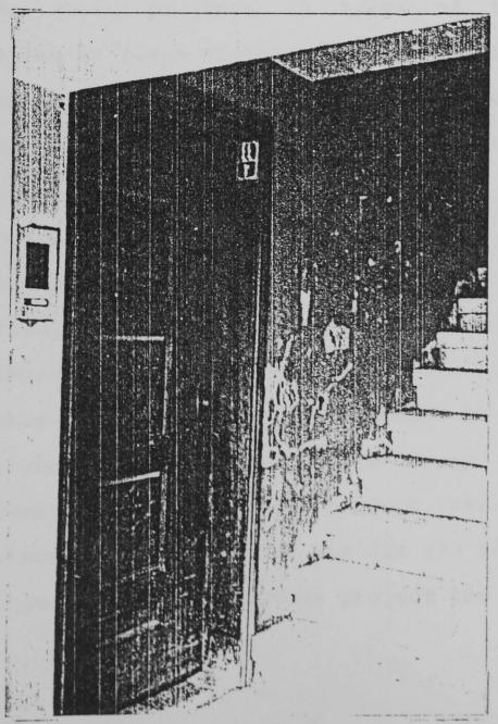
FIG.8.14 The awkward location the staircase in close proximity to the flats' entrance door.
