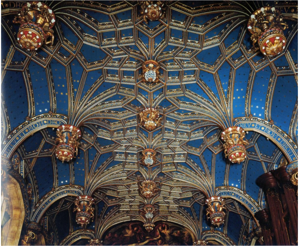
Figure 17:- Wooden ceiling vault of Hampton Court Chapel, erected c.1533-36, looking east.
