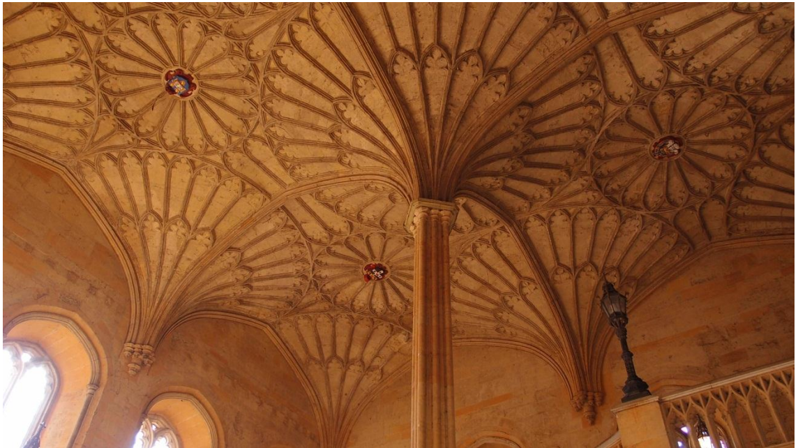
Figure 97:- Christ Church, Oxford. Fan vault over the hall stairs, attributed to Robert Smith, dated c.1636-38.
