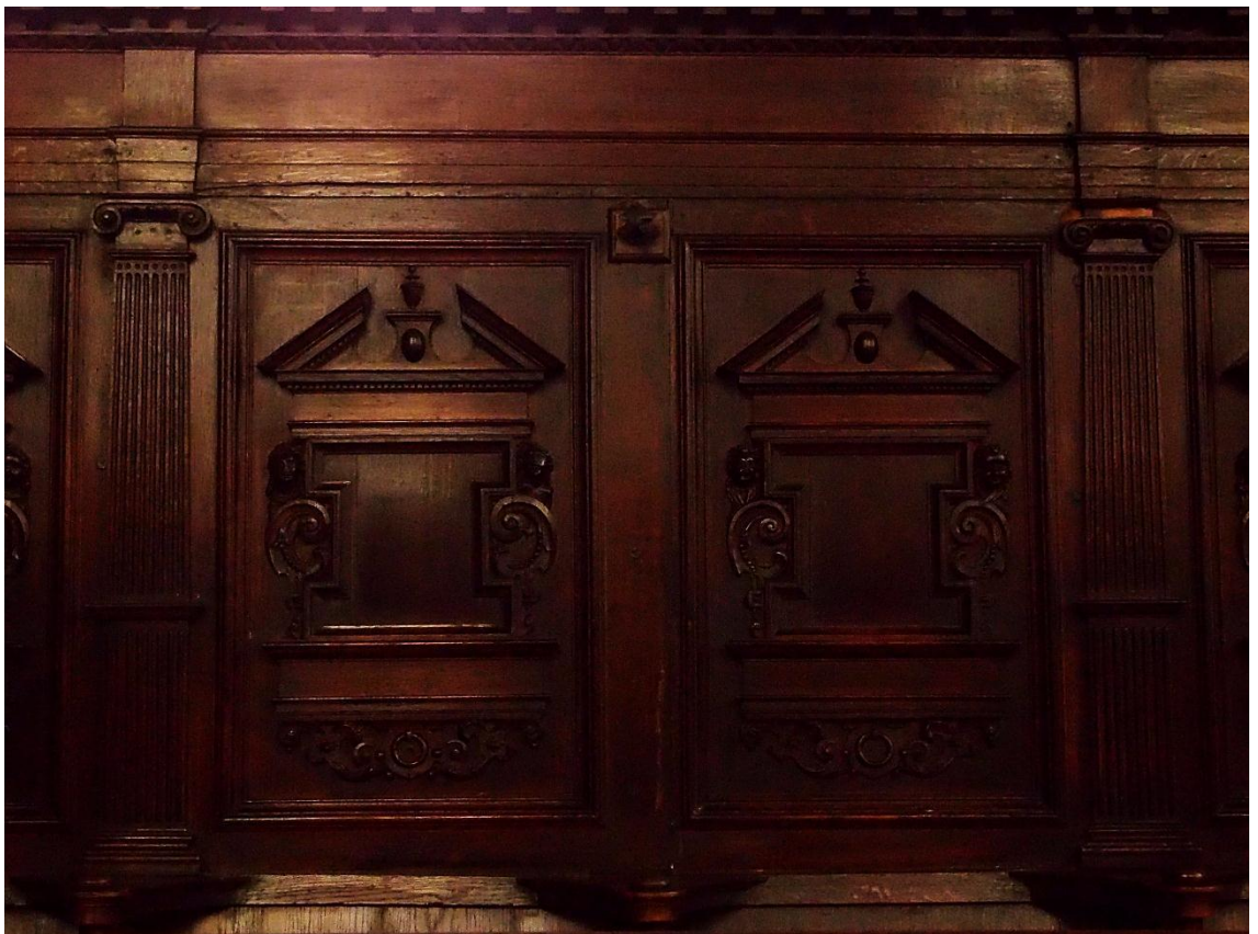
Figure 83:- Lincoln College Chapel, Oxford. Detail of wainscot panelling behind stalls, dated c.1629-32.
