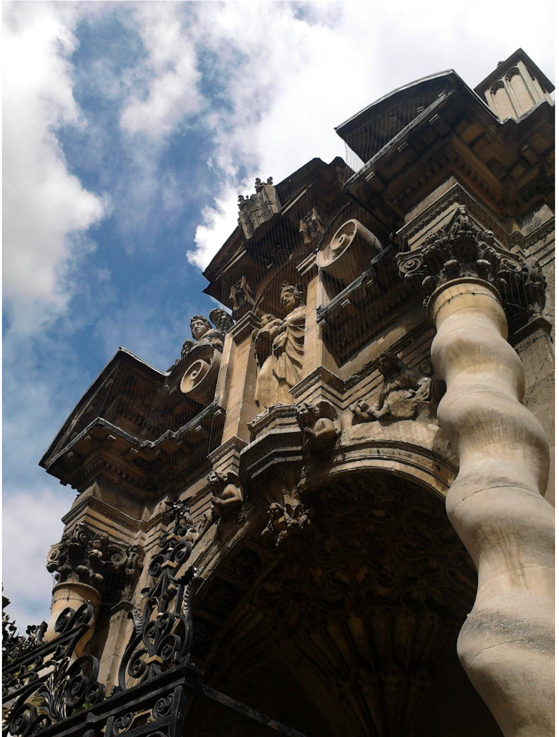
Figure 100:- Porch of the University Church, Oxford, design attributed to Nicholas Stone, executed by John Jackson, dated 1637.
