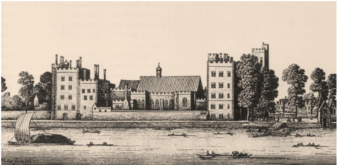
Figure 28:- Wenceslaus Hollar. Palatium Archiepiscopi Cantuariensis propæ Londinium vulgo Lambeth House , prior to the demolition of the mediaeval Great Hall, 1647. Engraving, 5¾"×12½".
