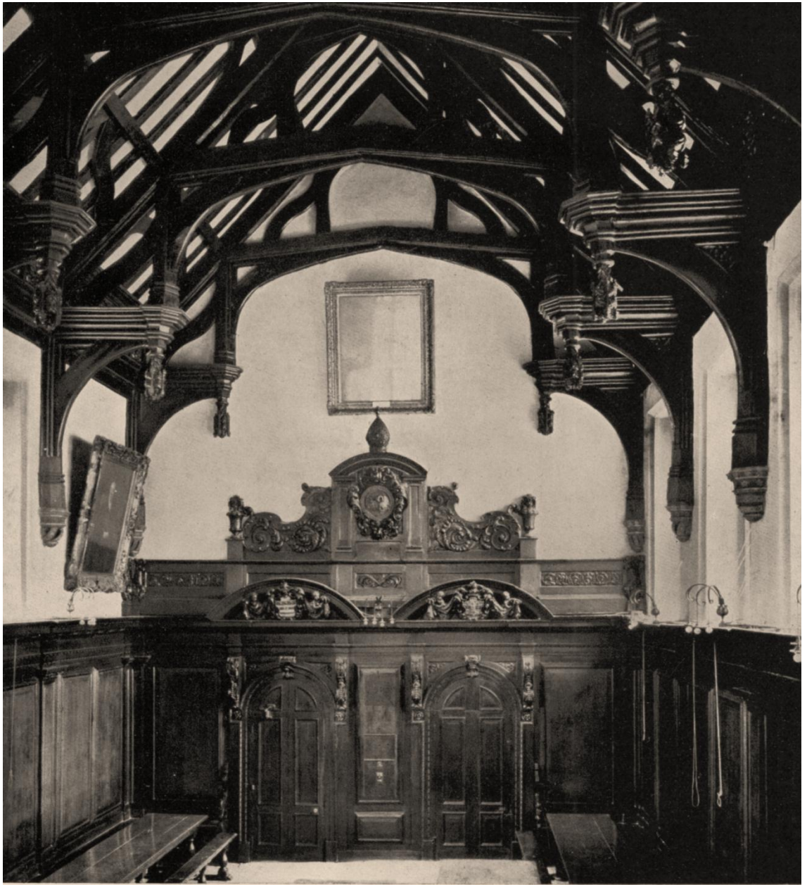
Figure 90:- Corpus Christi College, Oxford. Roof of the hall, attributed to Humphrey Coke, second decade of the sixteenth century.
