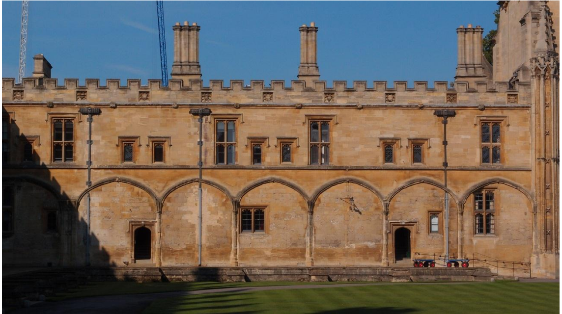
Figure 96:- Christ Church, Oxford. Tom Quadrange, showing the responds for the projected cloister, as left in 1529.
