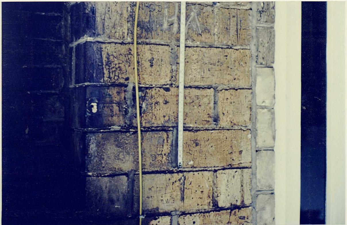
Figure 10.10. (top) and 10.11. (bottom) Porch constructed of hollow bricks in building at Banham, Norfolk (top). Close-up (bottom). [Photographs by author]
