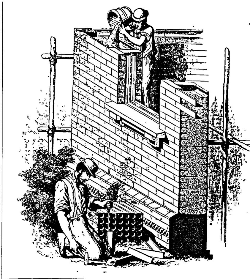
Figure 11.13. Construction of a concrete wall in stables and coach house at Hershams Lodge, Walton, Surrey using facing bricks manufactured by the Broomhall Tile Company.
