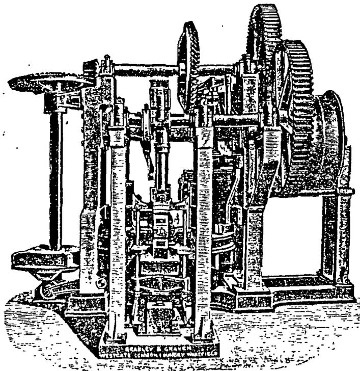
Figure 7.19. Stiff-plastic brickmaking machine by Bradley and Craven of Wakefield, c. 1890.
