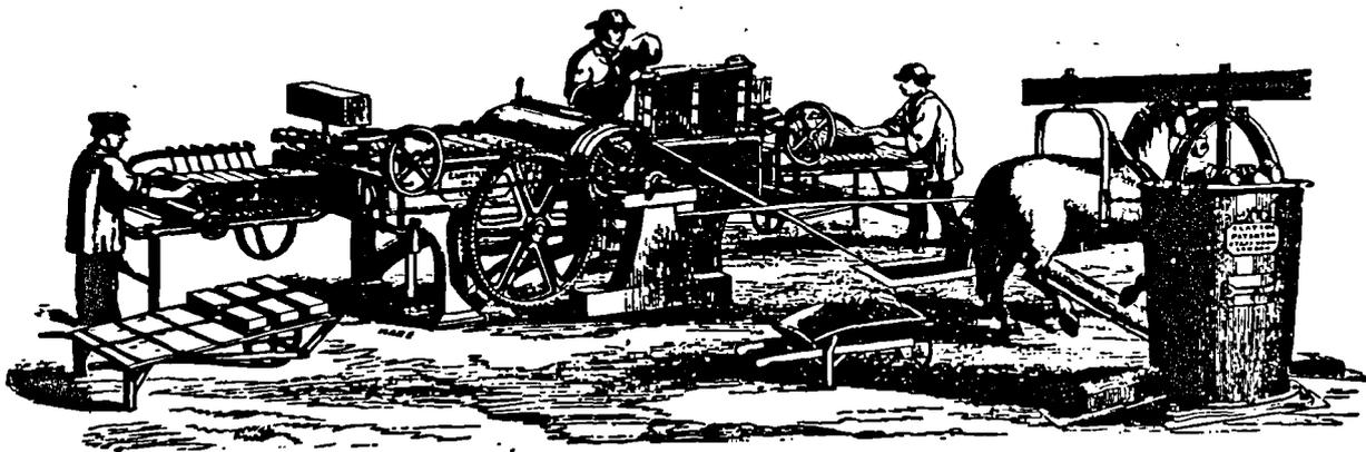
Figure 7.8. Henry Clayton's General Purpose "No. D" Brick and Tile Machine.
