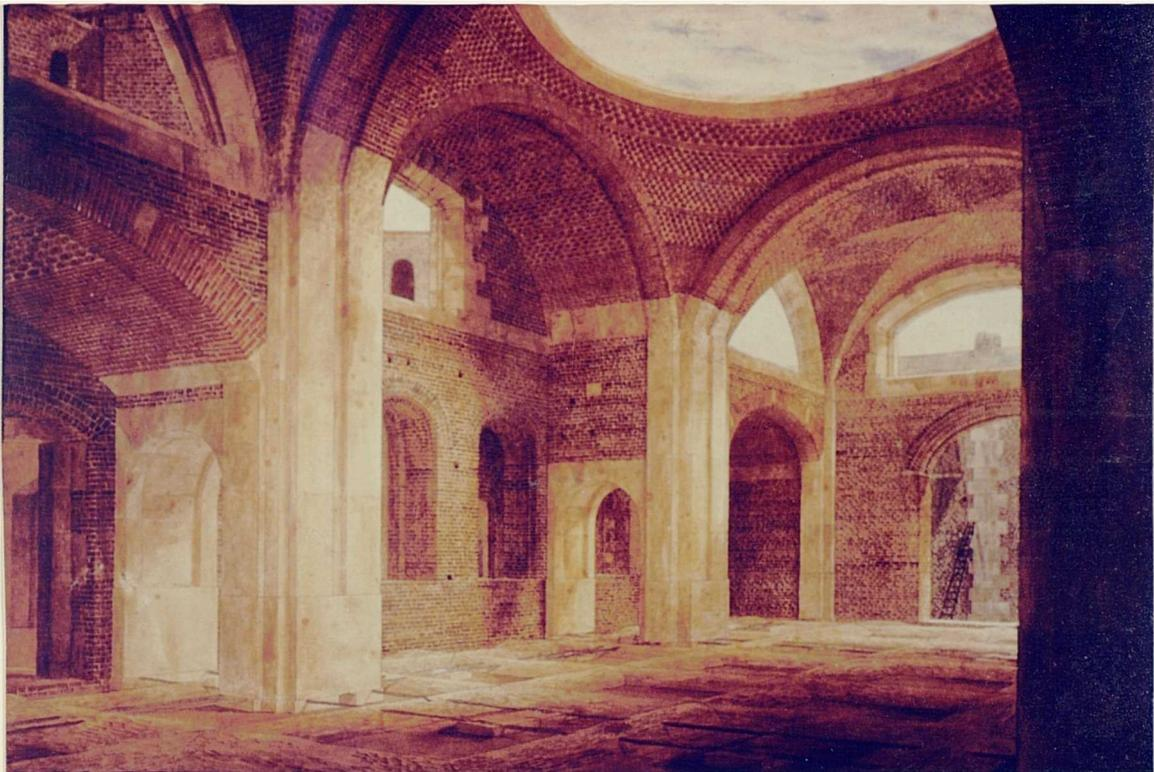
Figure 9.2. The Bank of England by John Soane; the Consol's Office before plastering, progress drawing by J. Gandy, 1799. [From John Summerson, John Soane (1983) p. 72]
