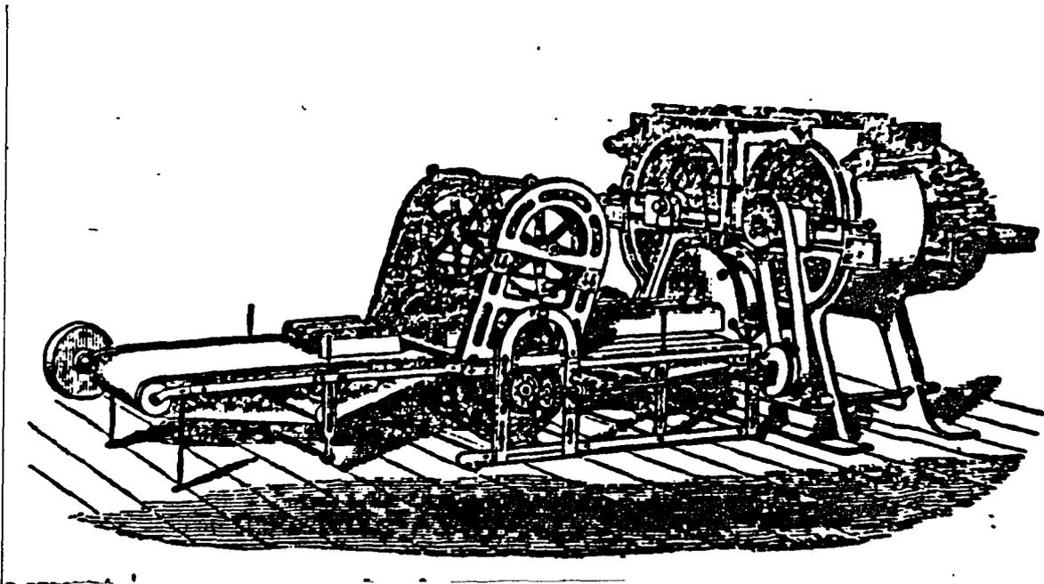
Figure 5.6. Brick and tile machine patented by John Ainslie, British Patent No.8965, 1841.
