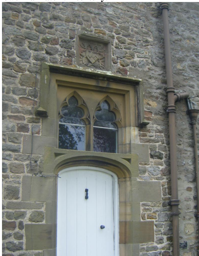
Figure 25 The Conyers-Wycliffe heraldry inserted above a door on the east side of the house, no longer used but which once would have led directly into the lower hall late 15 th century.
