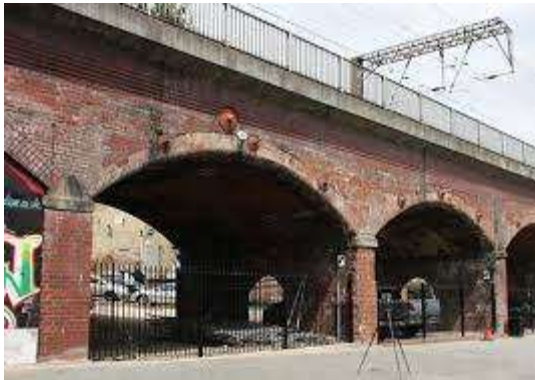
a) Marsh Lane Viaduct
