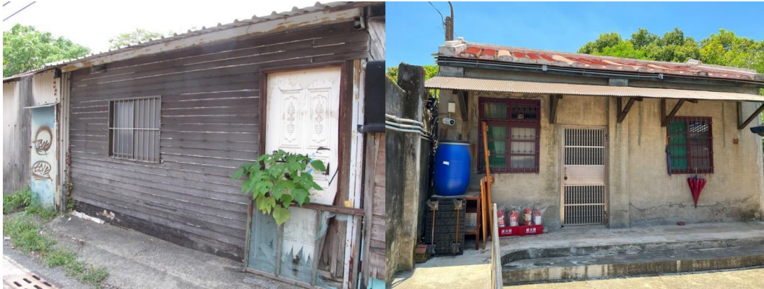
Figure 5.1: Un-demolished old MDV dwellings (Source: Author's own)
