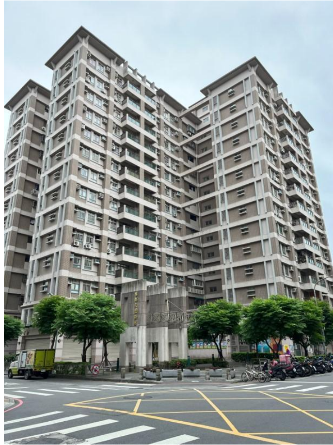
Figure 5.10: Reconstructed MDV housing of the second phase (Source: Author's own)
