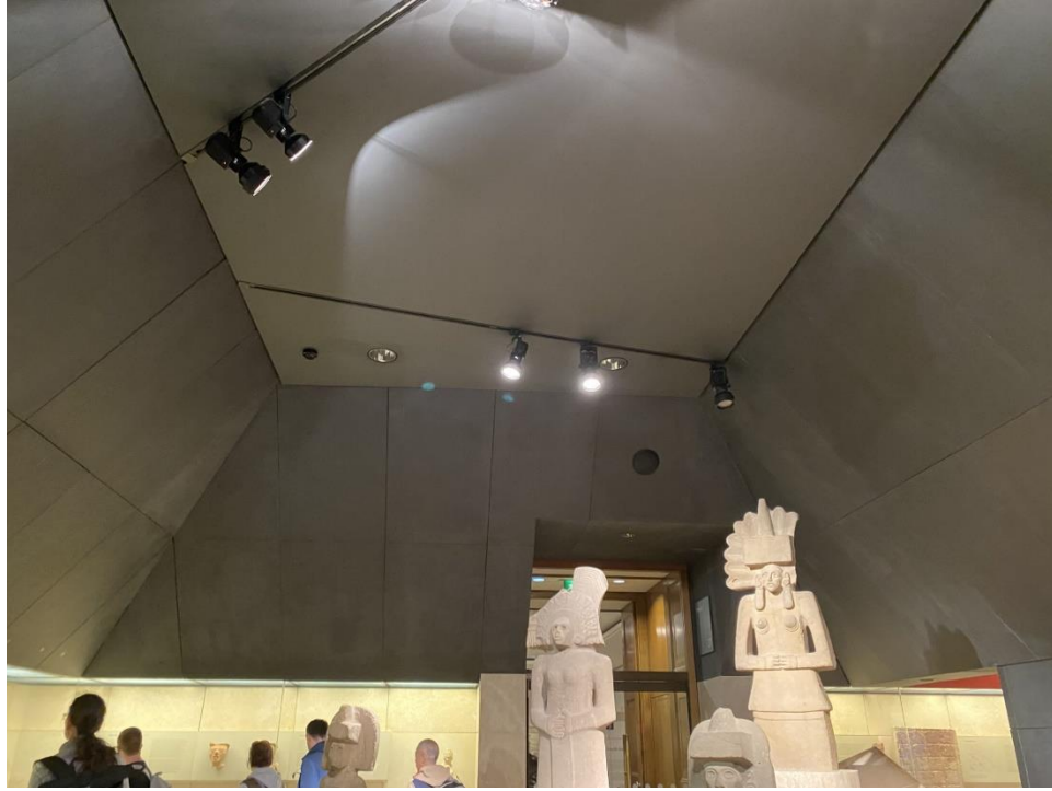
Figure 8: View of corbelled roof.
