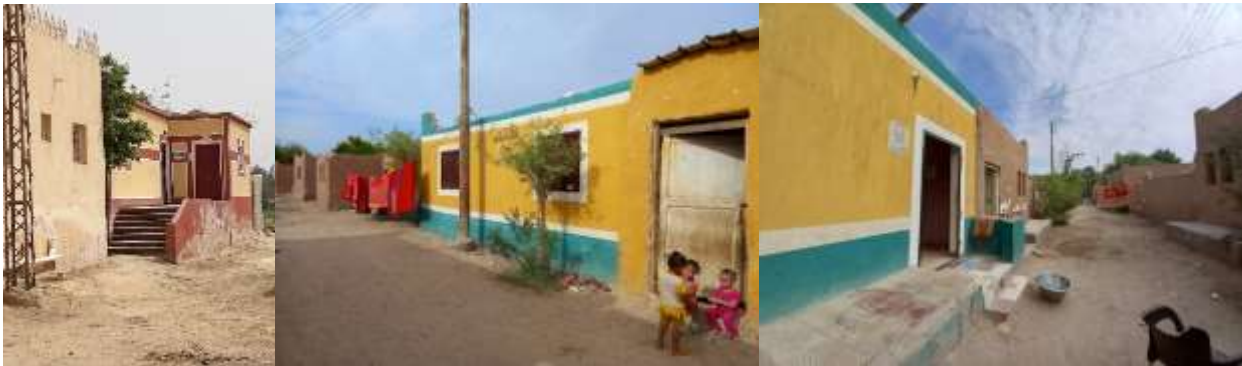
Figure 5-3: Left: House restored by Alorman in Benisuef. Right: House restored by LMF for Hayah kareema house in Sohag
