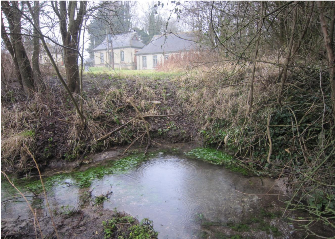
Figure 9.3a: The current 'issue' at Wellhead, with Connington Pumping Station in the background, photographed in mid-March. Prior to the construction of the pumping station in the early 1930s, the stream was fed by two springs issuing from adjacent deeply-eroded depressions, c.100m further north.
