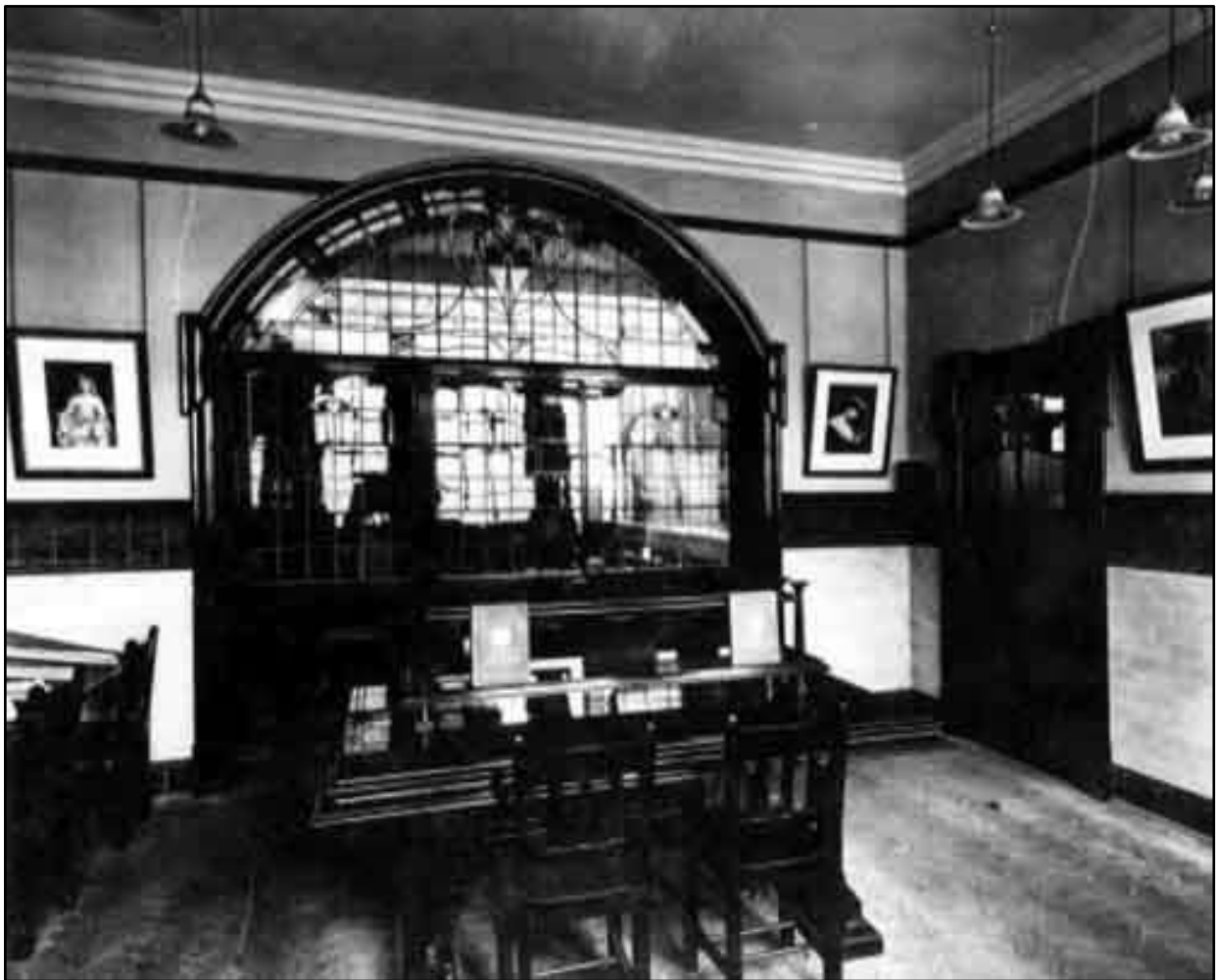
Image 7.48. (1902). Ladies’ Reading Room. Dewsbury Branch Library. Leeds Library. Leodis.
