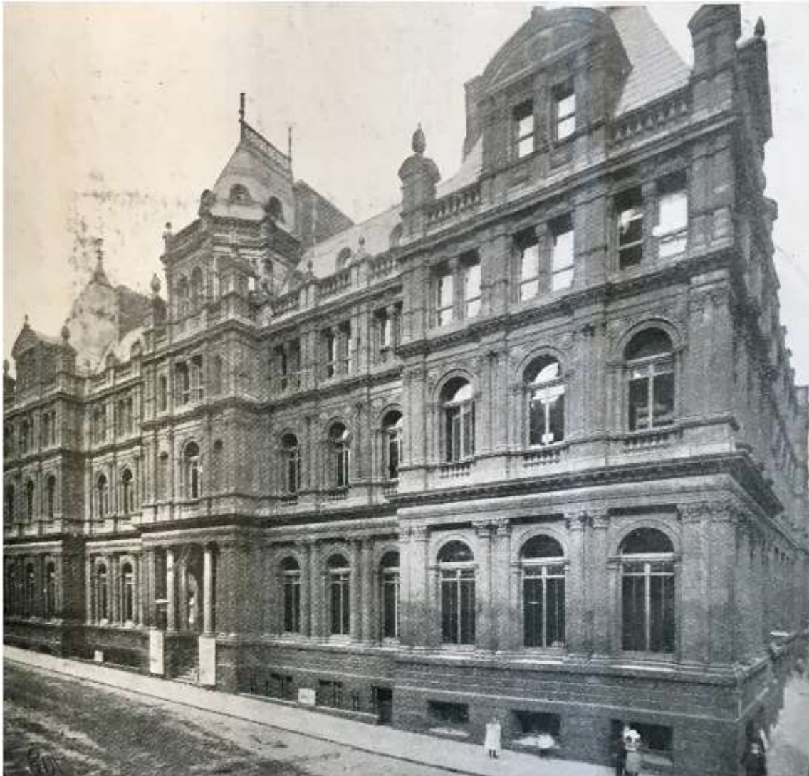
Image 7.43. Leeds. The Municipal Building. (1909). A History of Leeds Central Library . Leeds Library and Information Service. Leeds, Yorkshire, England.
