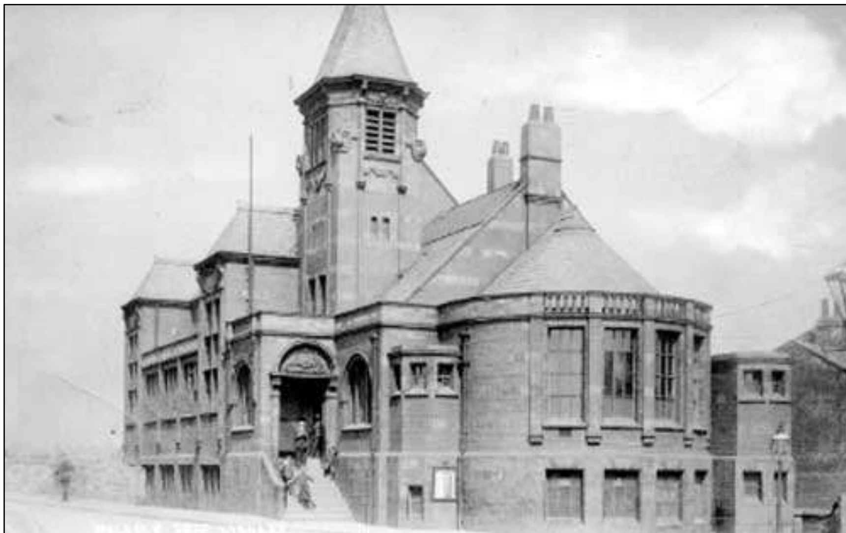
Image 7.52. (1903). Exterior. Holbeck Branch Library. Leeds Library. Leodis.
