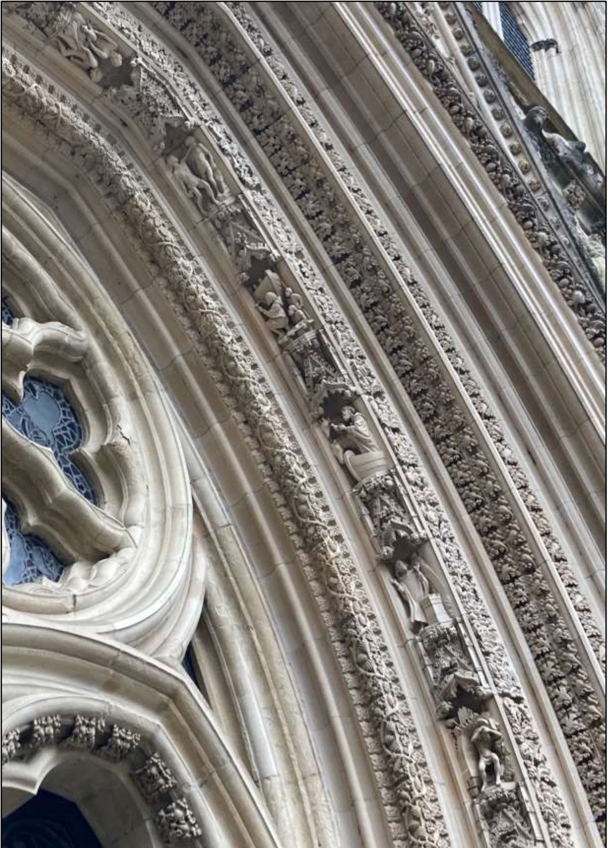
Image 7.99. (2023). Entrance Arch Detail. Exterior of York Minster: West Facing Narthex. Detail(s) of Entrance Arch 1230-1472. York, England. Authors' Own Image
