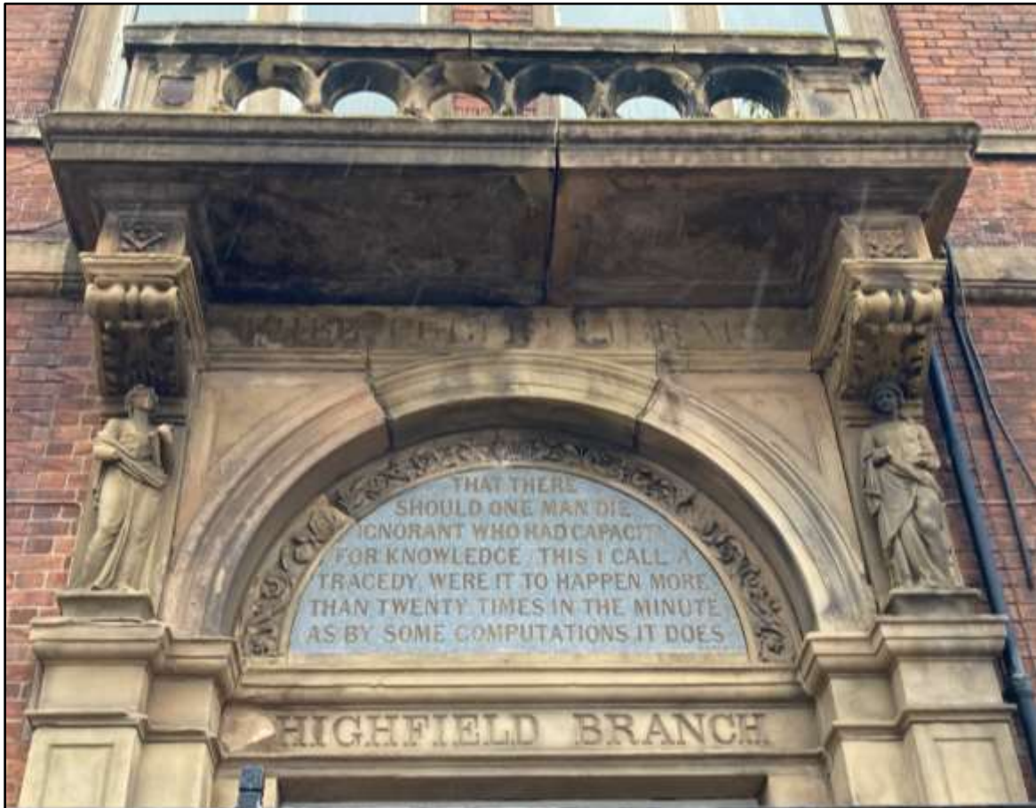
Image 7.74. (2023). Detail of Entranceway. Highfield Branch Library. Author’s Own Photo
