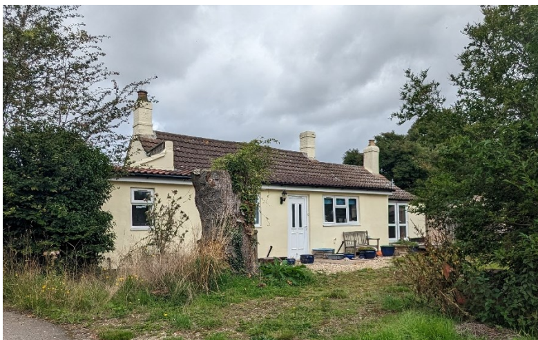
Fig. 88. Toll Bar Cottage from the south-west
