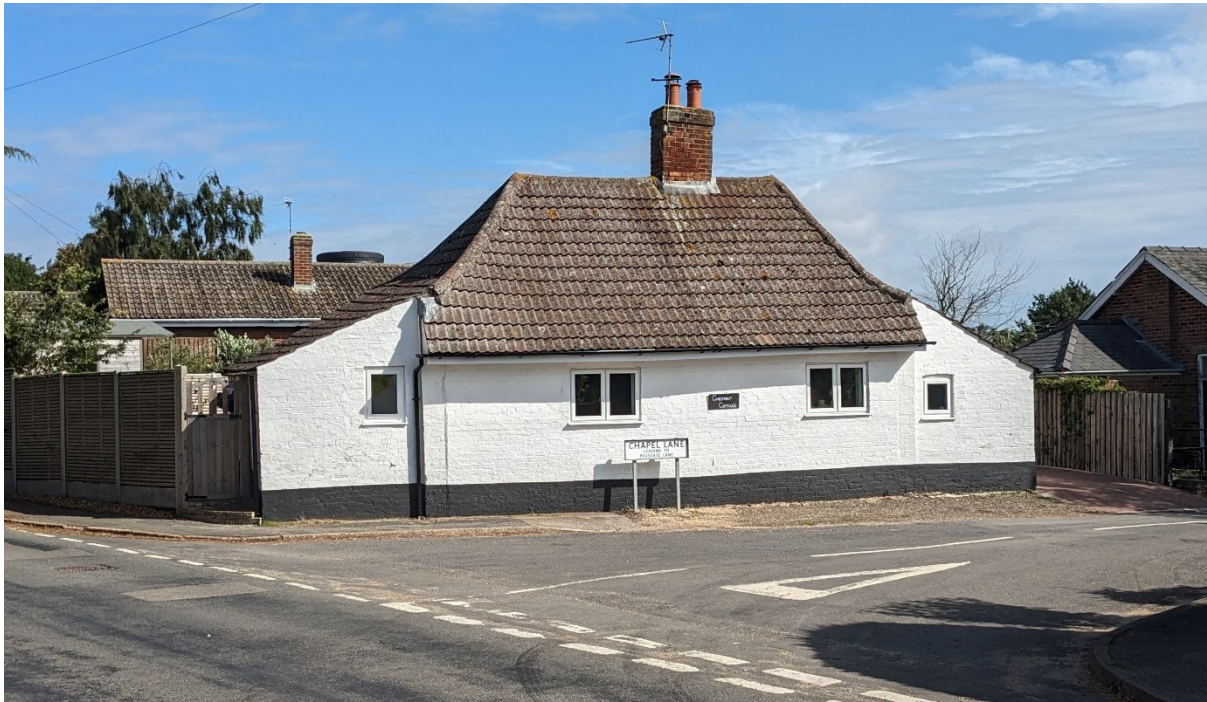
Fig. 94. Chestnut Cottage from the south-west
