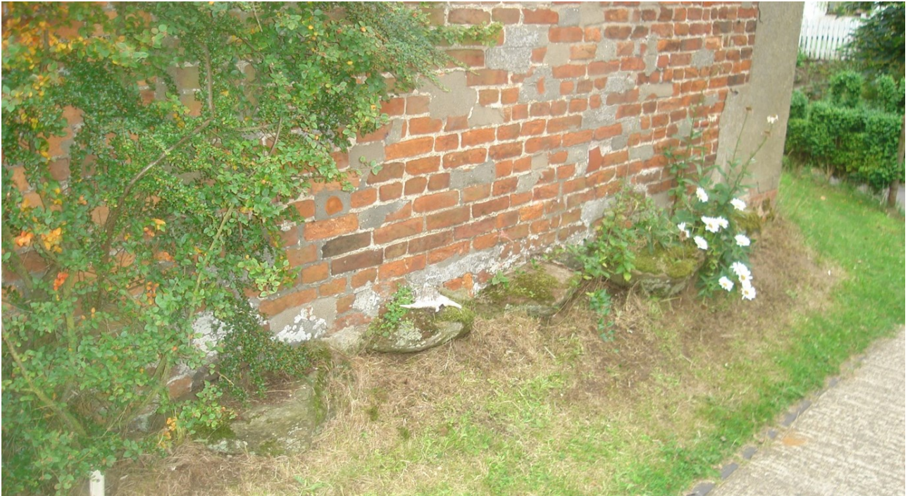
Fig. 30. Row of padstones/plinth below western gable wall
