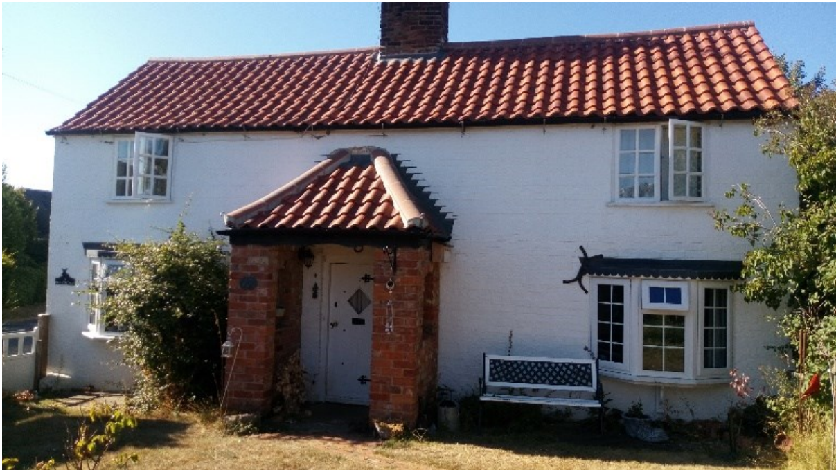
Fig. 92. Mill Cottage from the south
