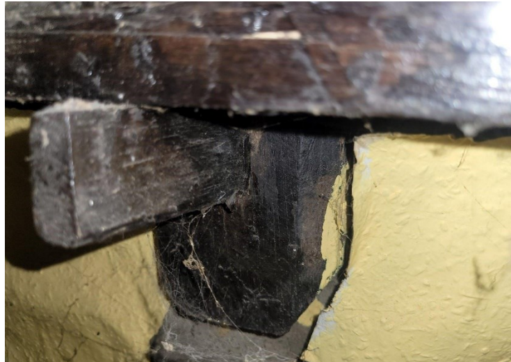
Fig. 63. Joint in the southern wallplate (courtesy of Richard Locke-Wheaton)
