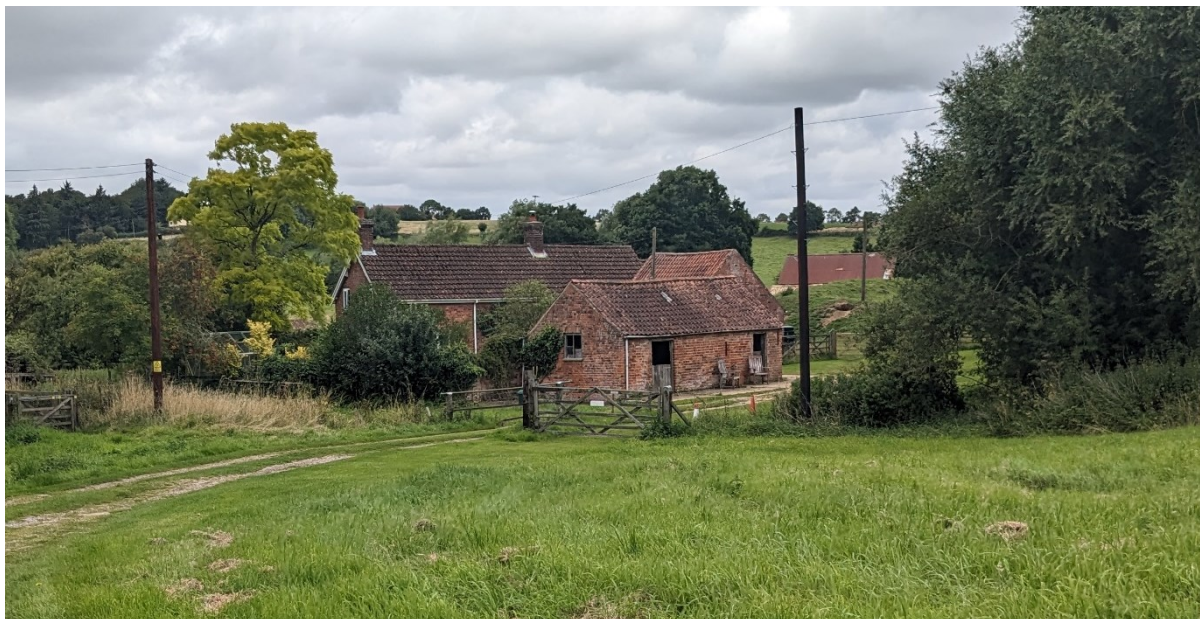
Fig. 107. The Watermill from the south-east. The mill building is the short pan-tiled building behind the stable, with the mud and stud mill cottage to the left (with modern roof)
