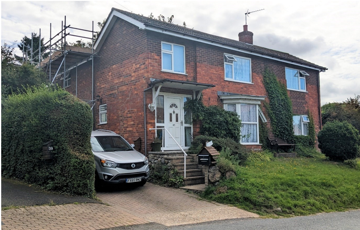
Fig. 126. Harboro House from the north-west
