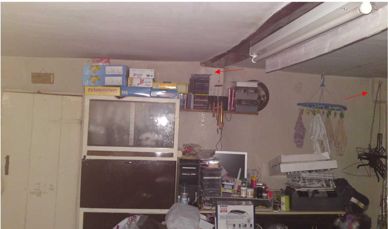
Fig. 31. Northern wall of the former hall. Note the undercut 'corbel-like' post in the top right corner, and visible mid-post, centre, supporting the binder. The door leads to the outshut, now the kitchen.
