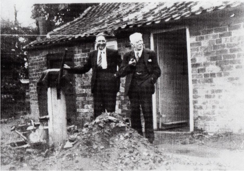
Fig. 43. Rear of The Cottage soon after purchase in 1951, with water pump and chimney for the copper visible (courtesy of Phyllis Pape)
