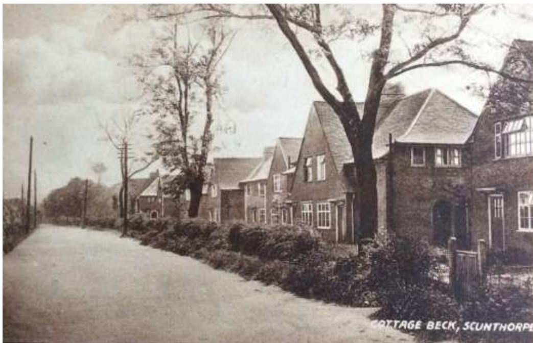
Figure 46 This postcard shows part of the northern section of the Redbourn Village Society scheme not long after completion. The view is actually of Roland Road and not Cottage Beck Road. There are aspects of this photo that could be said to be "garden city" esque and these would be the trees, modulated frontages, low eaves, gables fronting the road etc. Unknown copyright, used under fair use exemption.
