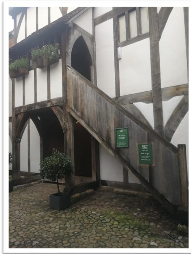
Figure 10. The door at Barley Hall that now is used as an exit for visitors.
