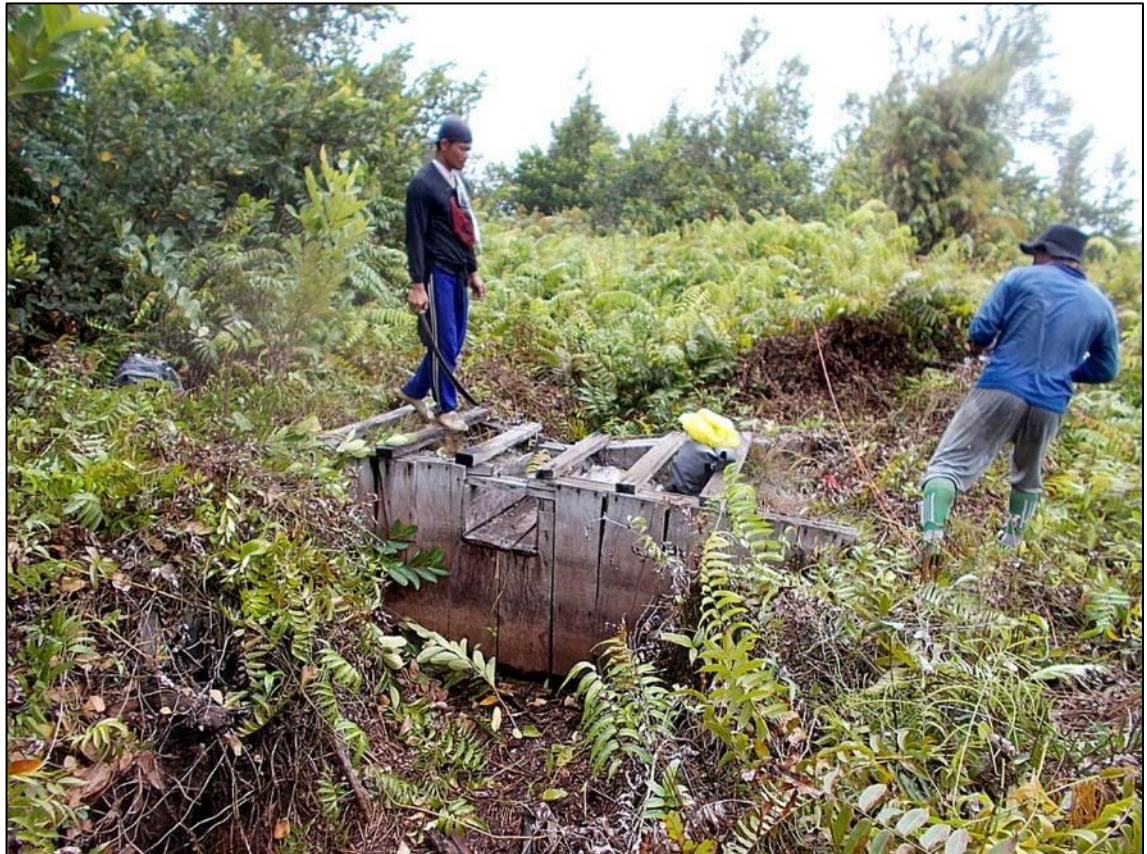
Figure 2.1 Drain blocking dam in the study site, Sebangau, Indonesia.
