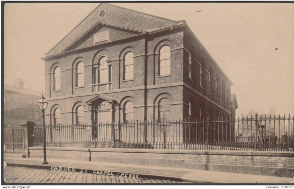
Figure 3.6: Sheffield Photo Company c. 1905. Monochrome original photographic postcard showing a view of the Methodist Chapel, Carver Street, Sheffield (No S.P.C. 535, 1905).
