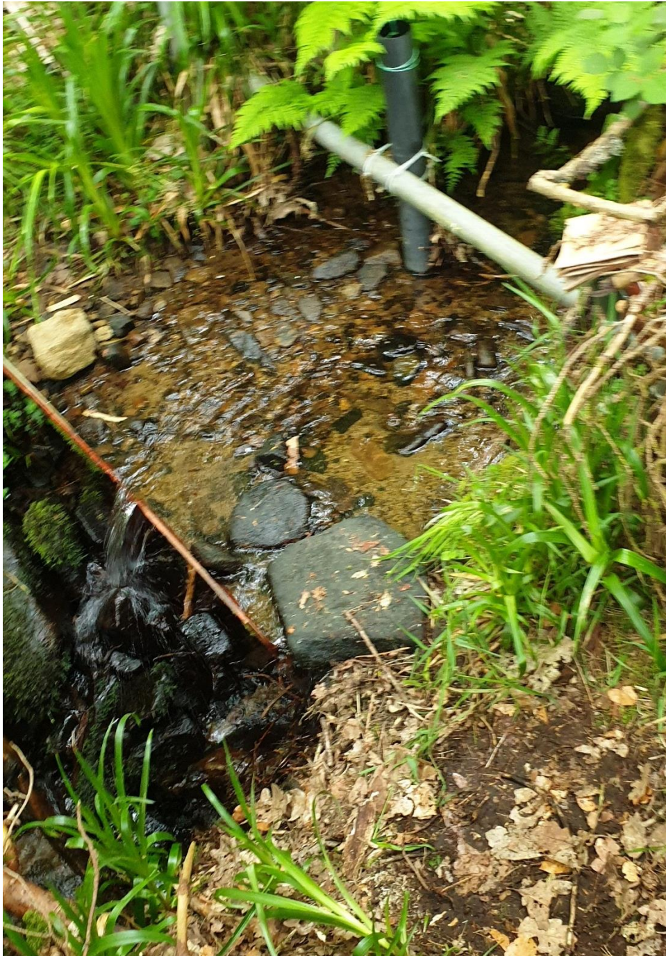
Figure B.2 – An example of increased sedimentation behind the V-Notch weirs
