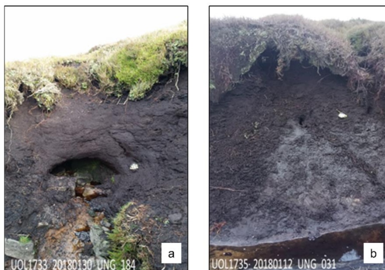
Figure 1.4 Typical examples of the outlets of two types of pipes: a) pipes that sit at interface of peat and bedrock and b) pipes that sit within the peat .
