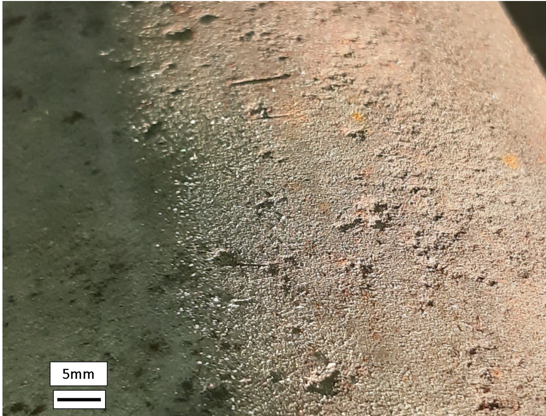
Figure 5.9: Image of the surface one of the donated axles, demonstrating visible corrosion damage
