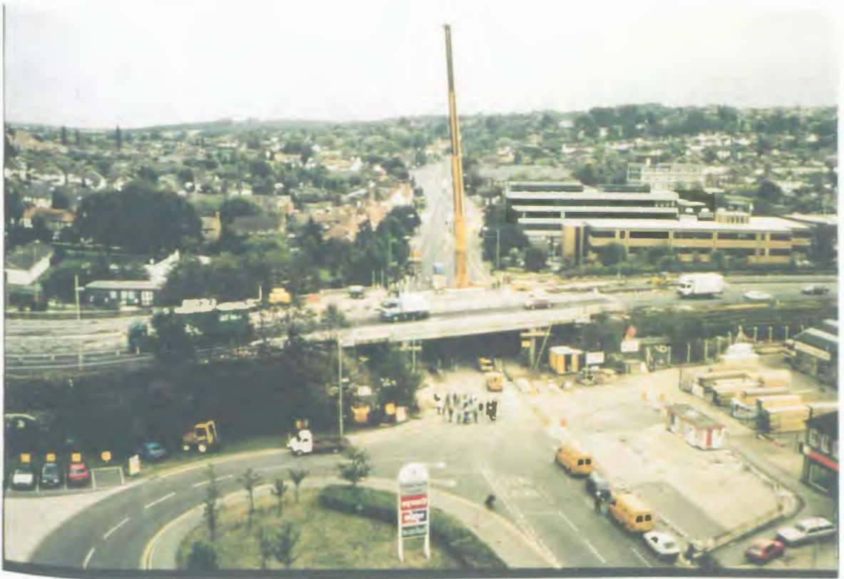
Plate 3.1 Aerial view of the Botley Flyover (Darby, 1996)
