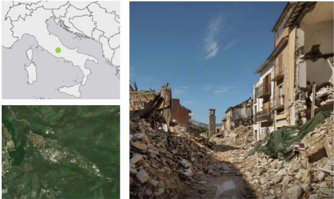
Figure 23: (Right) Geographic location of Amatrice (Left) The main street "Il Corso" after the 2016 earthquake
