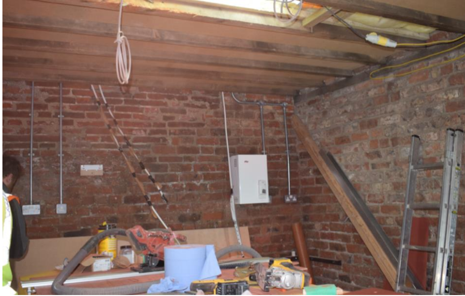
Figure 19: Visit to the building site on the 17-01-2018 ©images by the author
