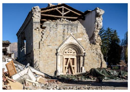
Figure 7.1: Progression of the damage to the façade of Sant'Agostino after the earthquakes of August 24 and October 30, 2016. To note the lack of propping systems that caused further damage to the building (November 2016). @Antonio Ranesi
