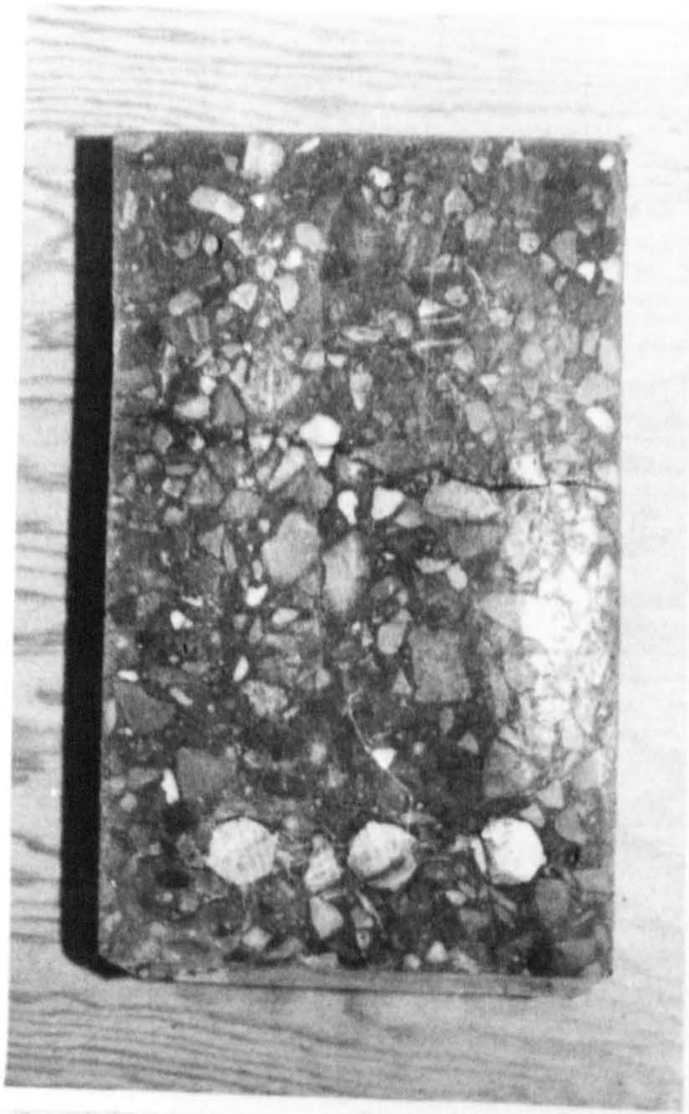
Section cut through a beam to test for carbonation of cement.
