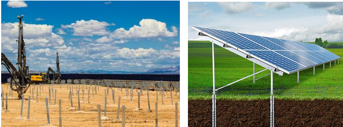
Figure 1 3: Screw piles for solar farm construction [39, 40]
