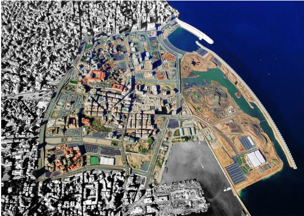
Figure 5-2: Aerial photo of Beirut Central District
