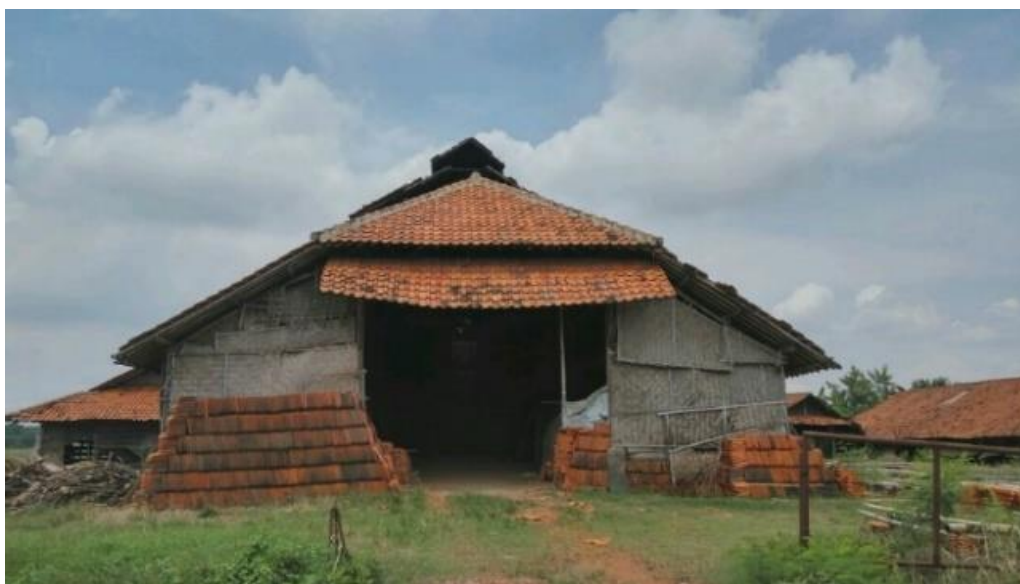
Figure 3-6 Tile kilns firing process
