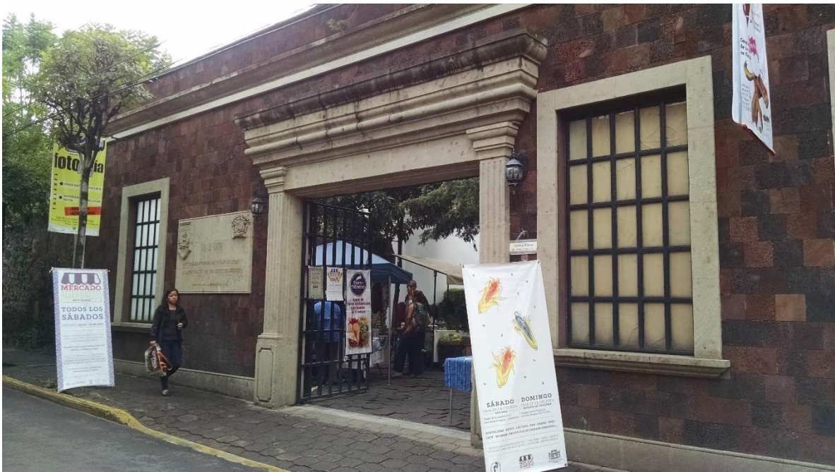
Figure 27. Exterior of the House of Culture where the AFM02 is set on Saturdays.
