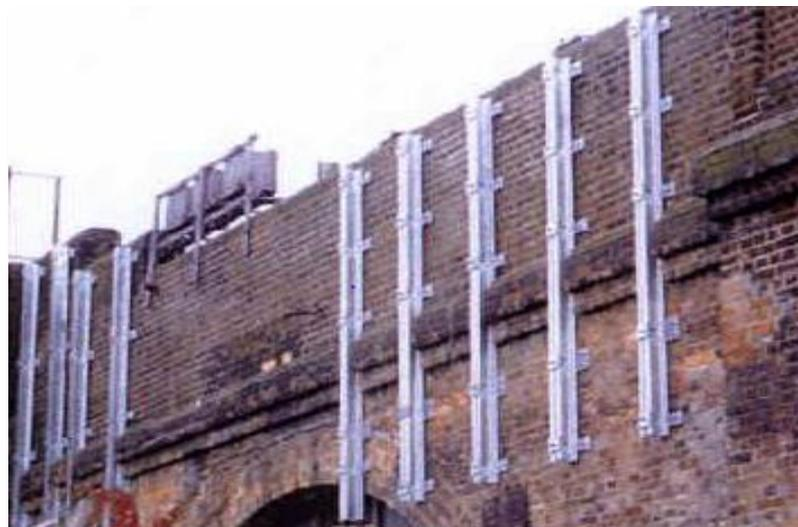
Figure 2.10: Externally strengthen wall with supplemental steel (Jansen & Tilly, 1999)
