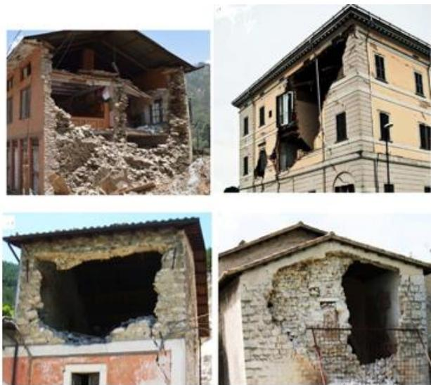
Figure 2.5. Out-of-plane failure modes of URM (De Santis et al., 2015)
