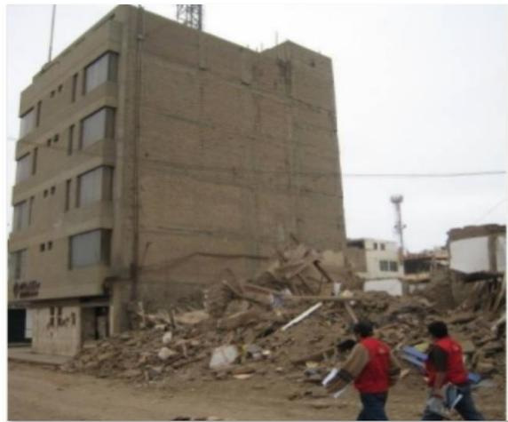
Figure 2.19: Performance of RC confined masonry in 2007 Pisco earthquake (Brzev, 2014)
